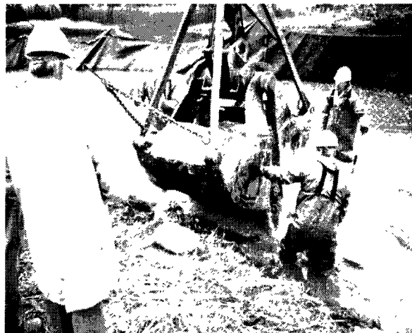
Figure 9. Land-based cap placement at Sheboygan River.
