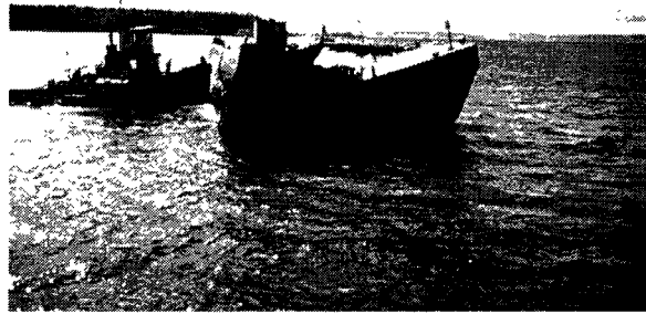
Figure 10. Spreading technique for capping by barge movement at Denny Way, Puget Sound.
