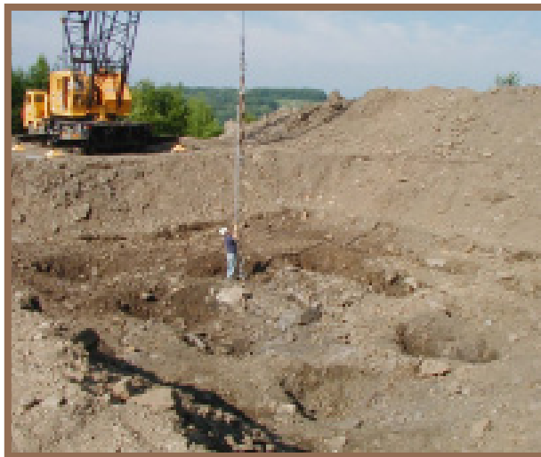
Step 1: Checking the stability of each proposed turbine location.
