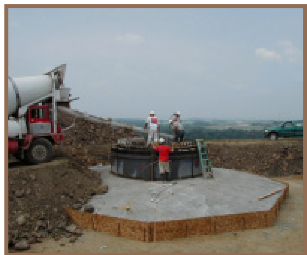
Step 3: Checking the stability of each turbine's foundation.
