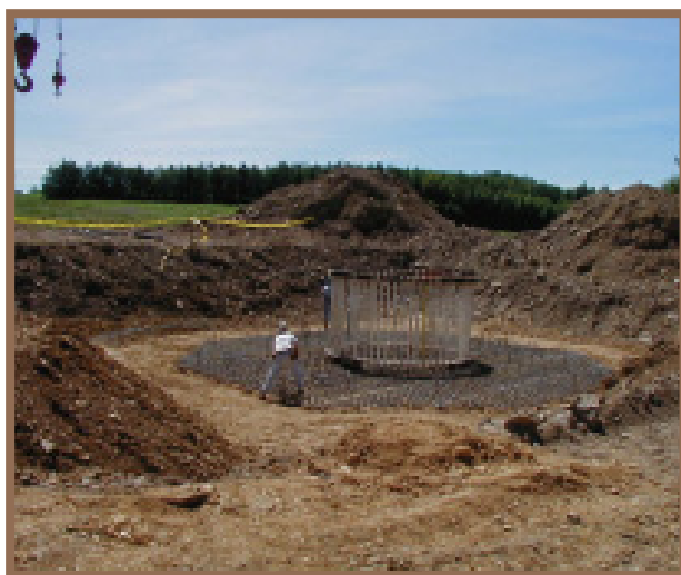
Step 2: Building each turbine's steel-reinforced concrete foundation.
