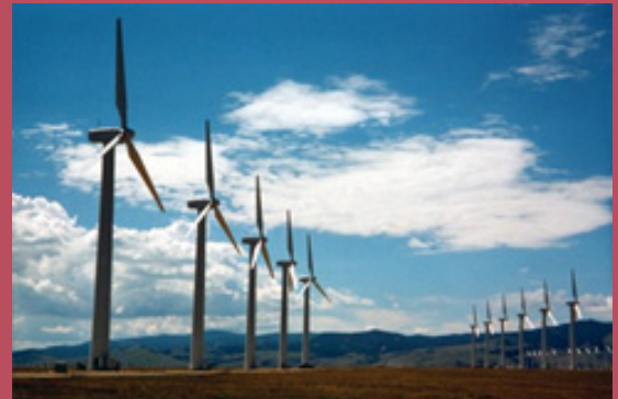
Wind farm in Wyoming. (source: National Renewable Energy Laboratory)
