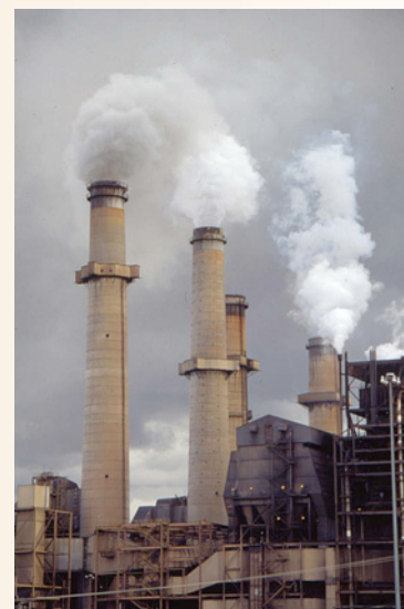
Four Corners Power Plant
