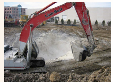
Sediment stabilization mixing operation
