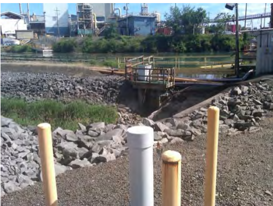
1635 – PHOTO 317 – Cooling water pond – receives Willamette River water from pump station on river for use throughout the plant. About to increase the pumping by ½ to allow replacing Pond 2 outfall flow into Truax Creek that
