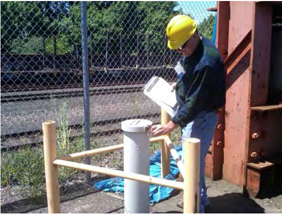
1328 PHOTO – 299 –View of well PW-47A – Well found locked, but with welded ring loose (requires maintenance), steel casing intact, cap present, measurement point visible, barrier posts present.
