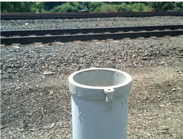
1340 – PHOTO – 300 – View of PW-24A – West toward railroad tracks and Second Lake – good steel casing present, locked well, measurement point present
