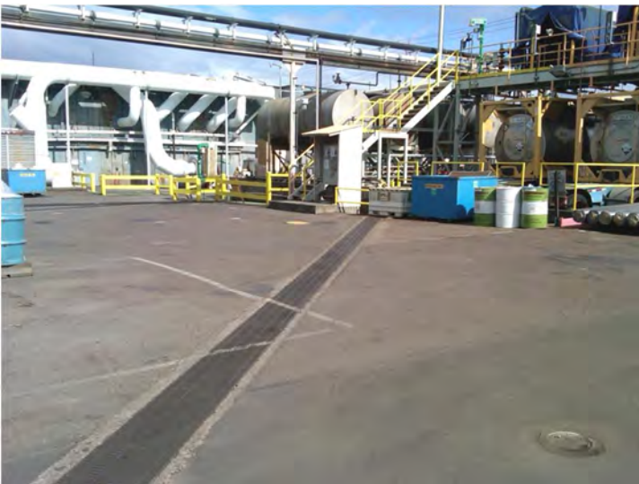
1645 – PHOTO 356 (Photo 355 deleted on site to better capture intended well pattern in courtyard) View southeast from area of PW-13 to show injection well in foreground toward the more distant TMW-4 and I-1 – the center of the apparent NAPL solvent source material which will require excavation or another remedial approach to achieve a protective remedy in this area
