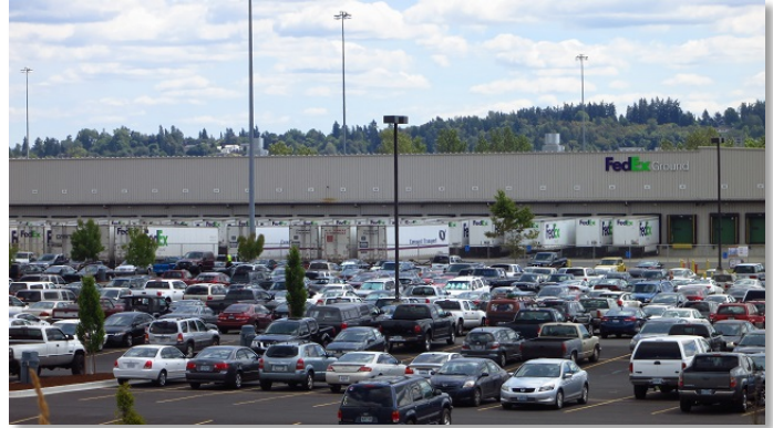
Figure 8. FedEx Ground facility on site.
