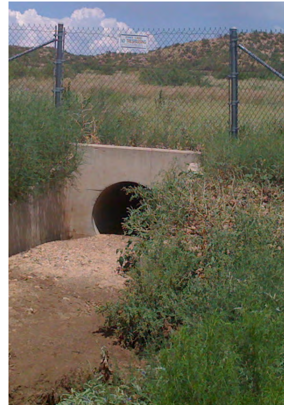
View of the Site's drainage features
