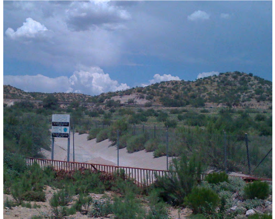
Concrete lined drainage channel
