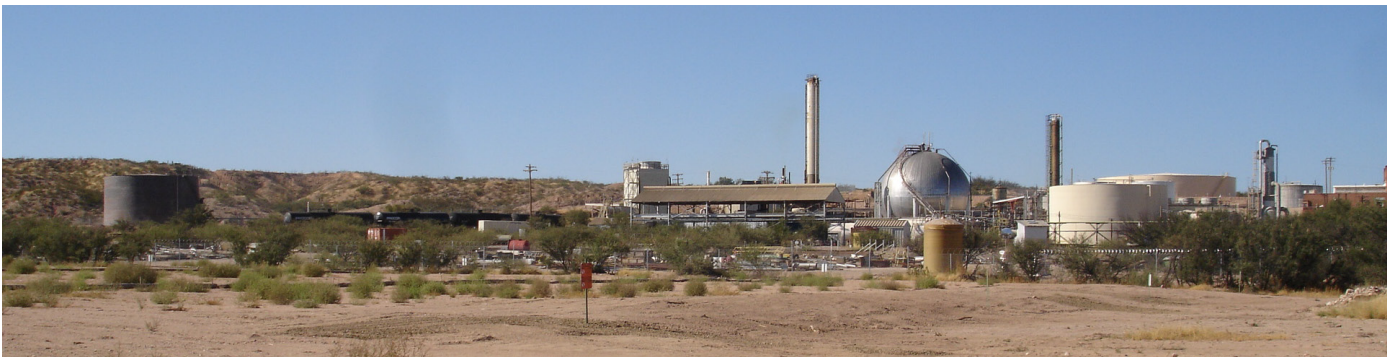
Top: Example of solar arrays installed at Nellis Air Force Base, Nevada. Bottom: ANP facilities at the Apache Powder Superfund Site, 2008.
