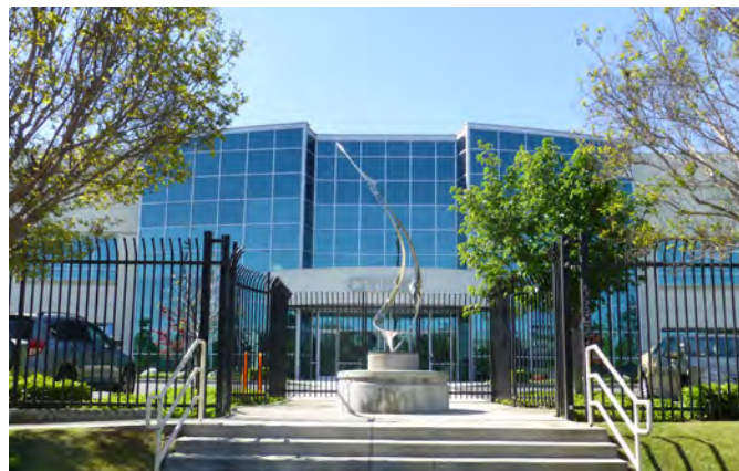
During construction of the new building on 1000 West 190th Street, sampling identified impacted soil, which the owner later removed.
