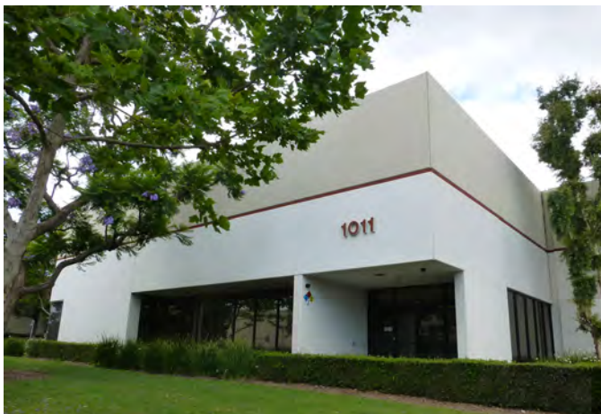
At 1011 Francisco Street, Shell removed and disposed of impacted soil during the tenant's planned construction activities.
