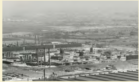
The chemical manufacturing facility on site before redevelopment.
