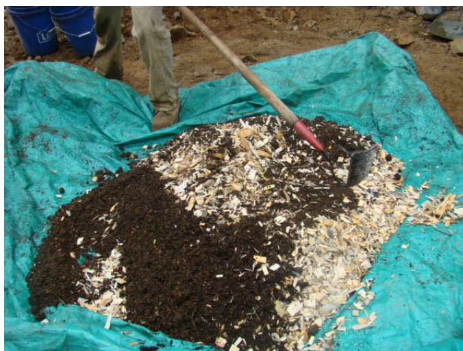
Exhibit 2-19. Mixing of a batch of BCR substrate.
