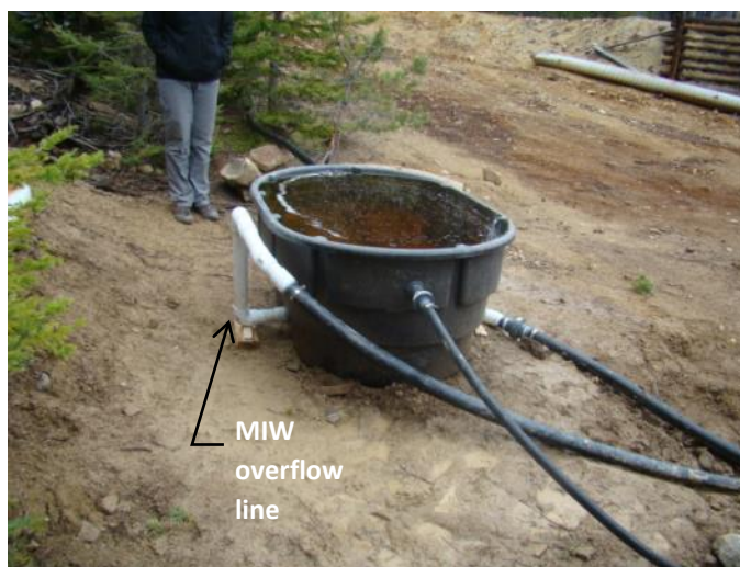
Exhibit 2-11. MIW overflow tank showing overflow pipe.
