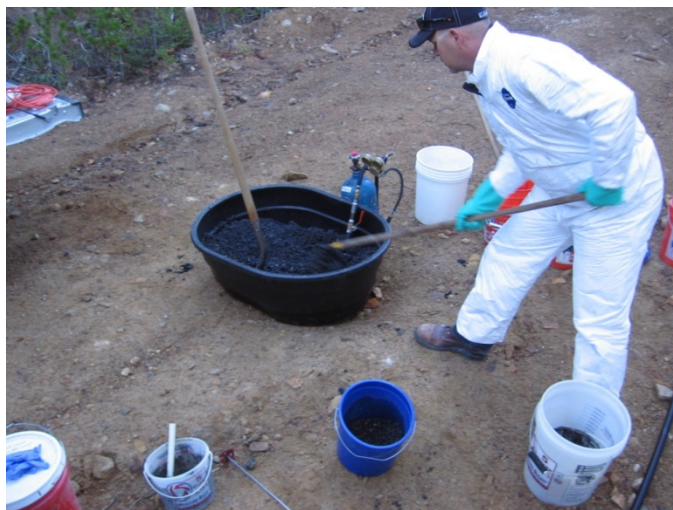
Exhibit 2-20. Mixing of pea gravel with the original Chitorem substrate.
