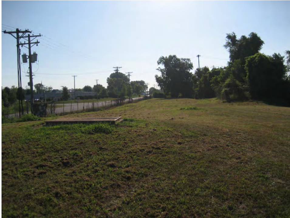
Lee Chemical looking east, with a bulkhead providing access to the soil washing operation in the foreground
