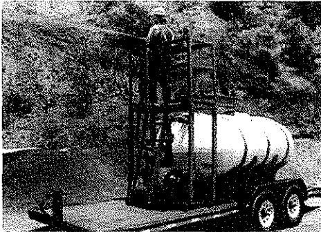
Figure 1 – Hydroseed application
