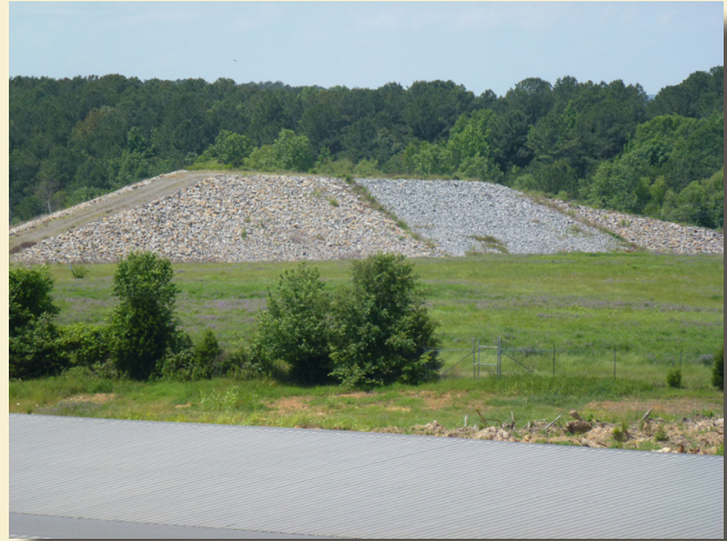
The site's cleanup included the construction of this above-ground vault known as the "Mount Vertac" landfill. It contains tons of contaminated soil and debris generated during site cleanup activities. Fencing restricts area access, landfill leachate is captured and treated, and ground water monitoring is ongoing.
