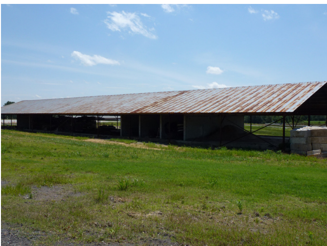
EPA drum storage sheds prior to their reuse by the City of Jacksonville.
