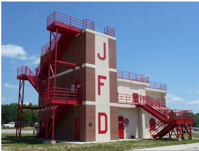
Fire training burn tower
