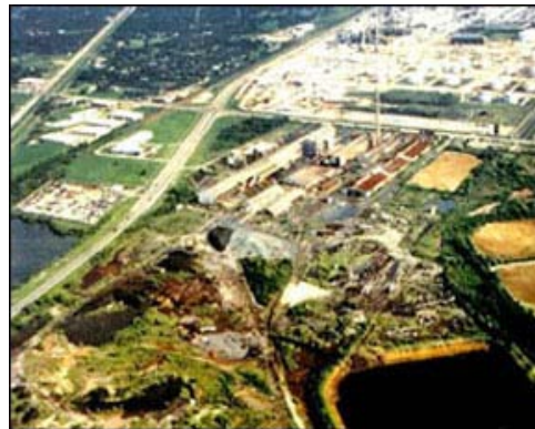
Pictured: Aerial view of the Tex Tin site prior to remediation. (Source: EPA)
