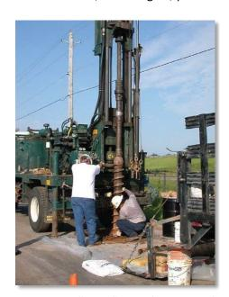
Figure 2. Well installation during remedy construction.
