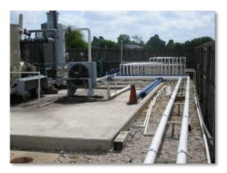
Figure 4. On-site LNAPL extraction and treatment system.
