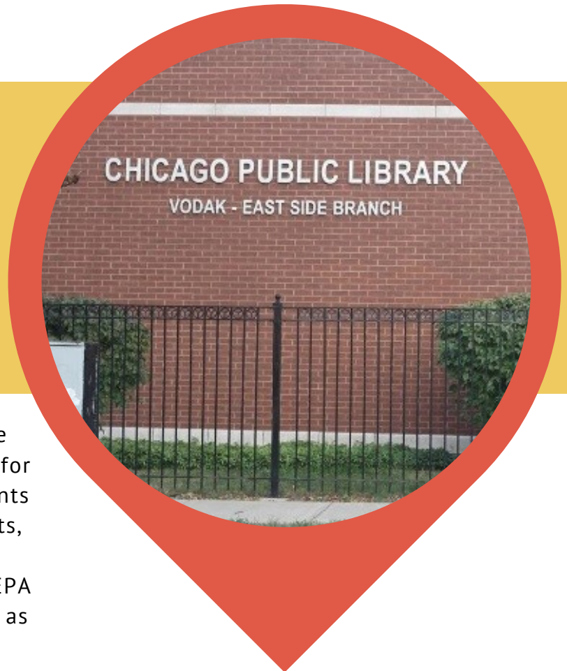
Vodak-East Side Branch Library
