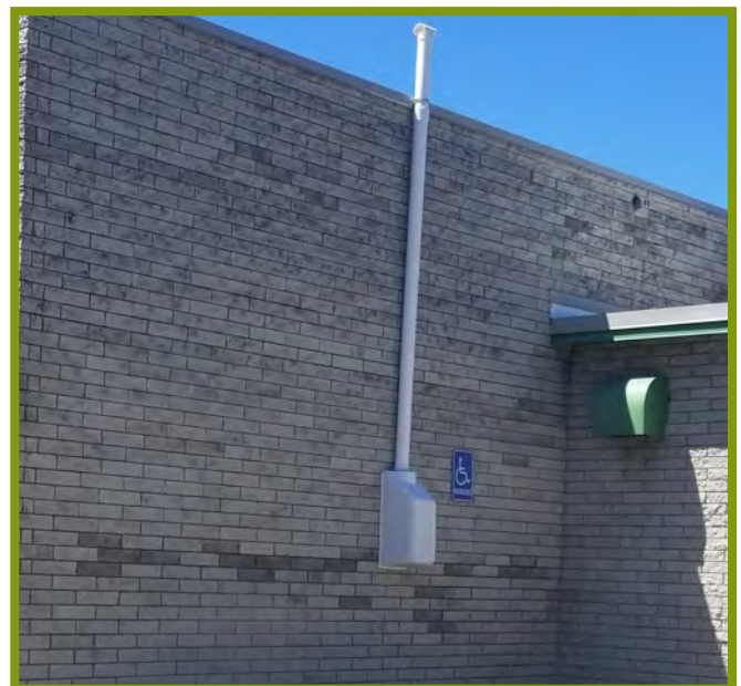
Photo of a soil vapor extraction system on the side of a building.
