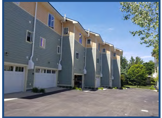
Vapor intrusion systems on side of condominium units.
