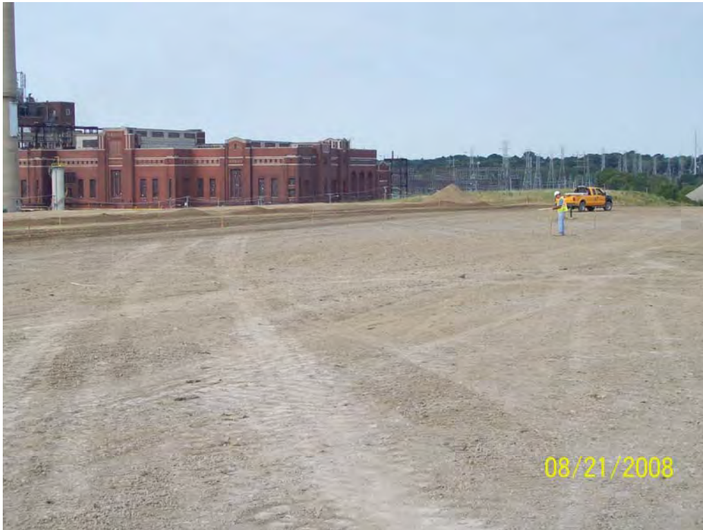
Photograph No. 5 Photographer: Chris R. Goffard Barrier layer surface complete on the west half of Area 1 Final Cover. Viewing west. Signature: Chris R. Goffard August 21, 2008
