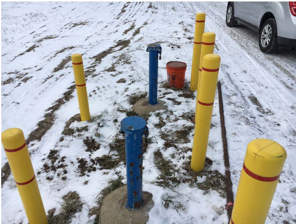
Monitoring well within waste disposal area, adjacent to landfill (typical)
