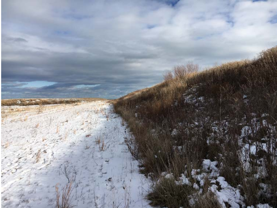
Photo looking east across northern berm separating Industrial Canal and Settling Basin.
