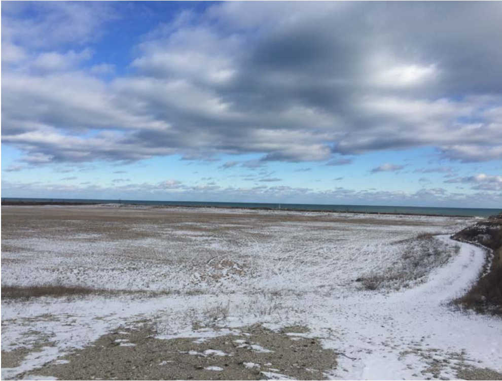
Photo looking northeast across Settling Basin
