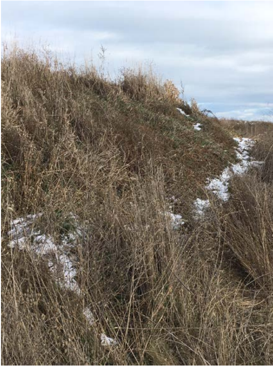
Northern berm along settling basin.
