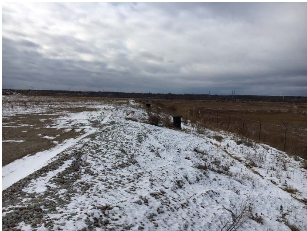
Photo looking west across stormwater pipe location between nature preserve and Industrial Canal
