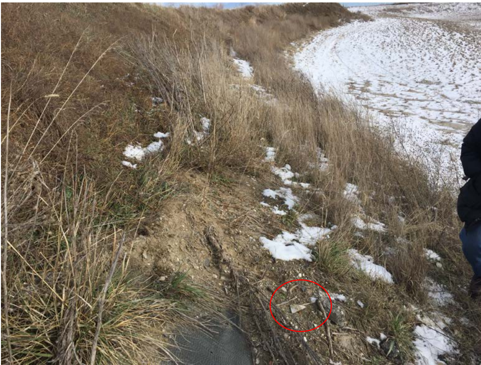
Material at base of animal burrow, potential asbestos containing material is shown (red circle). Burrow to be repaired and material disposed.
