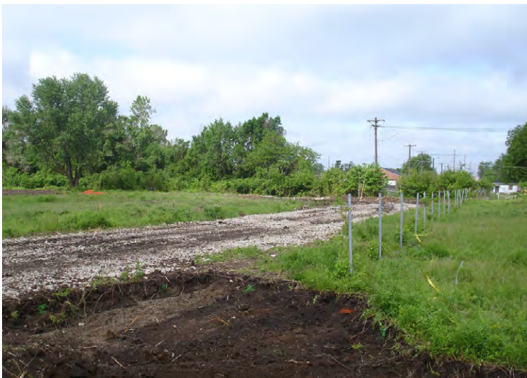
Former little league site during removal action
