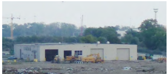
Waste Management's on-site maintenance building is a potential location for a roof-top mounted solar PV system.
