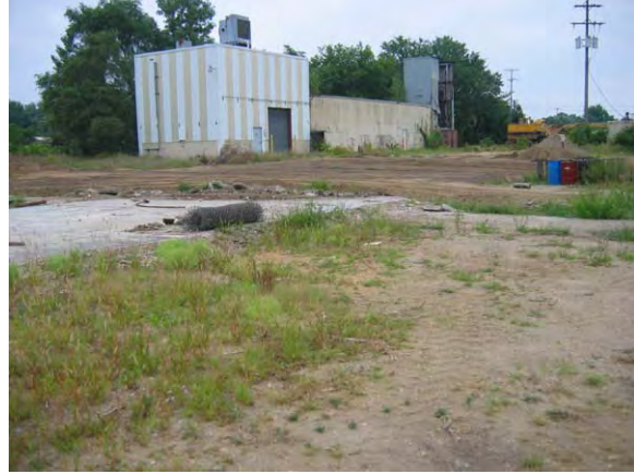
F. Striped building houses treatment system
