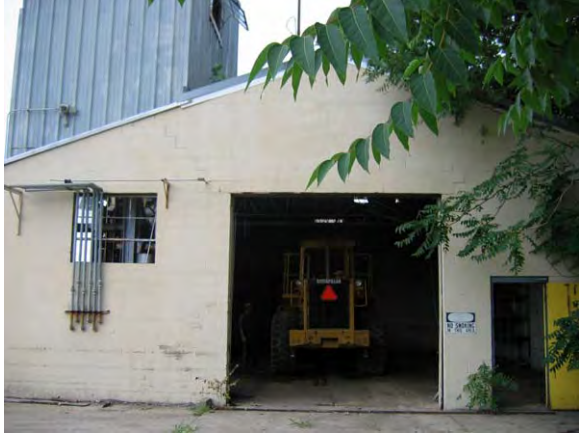
E. Former treatment building
