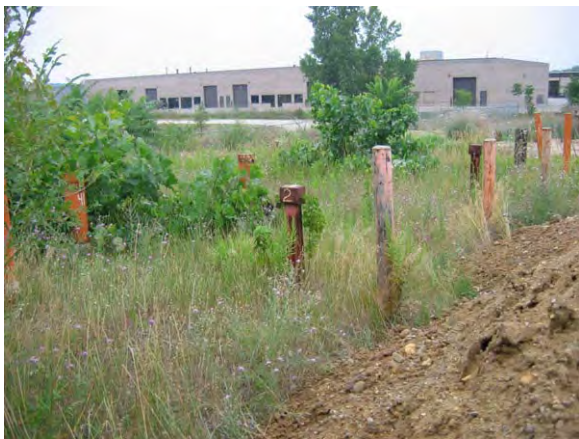
G. Monitoring wells protected by earth berms
