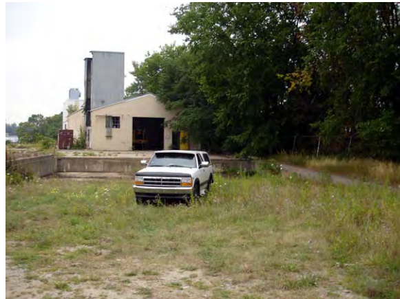
B. Former loading dock and solvent building
