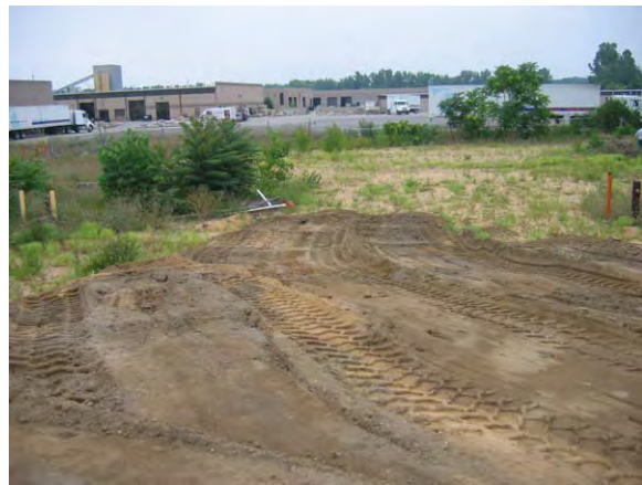
J. Lower level, northern portion of site
