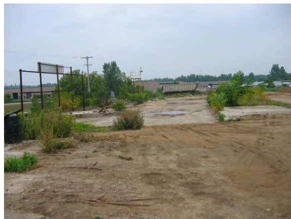
D. Former concrete slabs located throughout site
