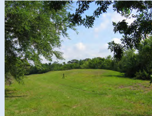
Soil cap with a monitoring well installed
