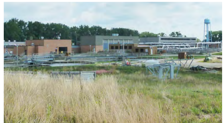
The City of Grand Rapids Waste Water Treatment Plant, located across the Grand River from the site (see Figure 3), receives electricity from Consumers Energy.
