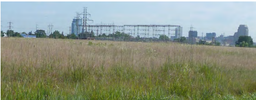
Capped area in Eastern Landfill Unit adjacent to the Consumers Energy substation
