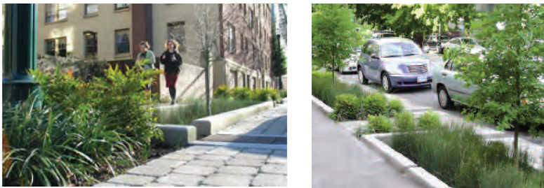
Porous sidewalk pavers and stormwater planters serve as pedestrian amenities and help to reduce runoff and improve water quality
