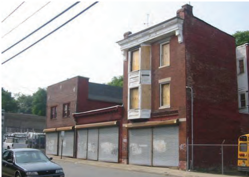
Valley Arts partner, Hands Inc., renovated the former West Orange Brass Company complex.
