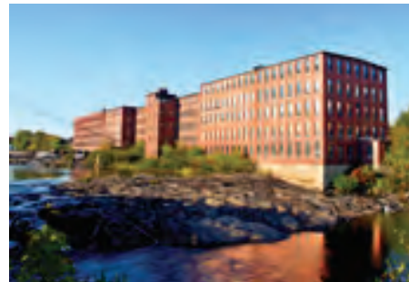
Presumpscot woolen mill building
