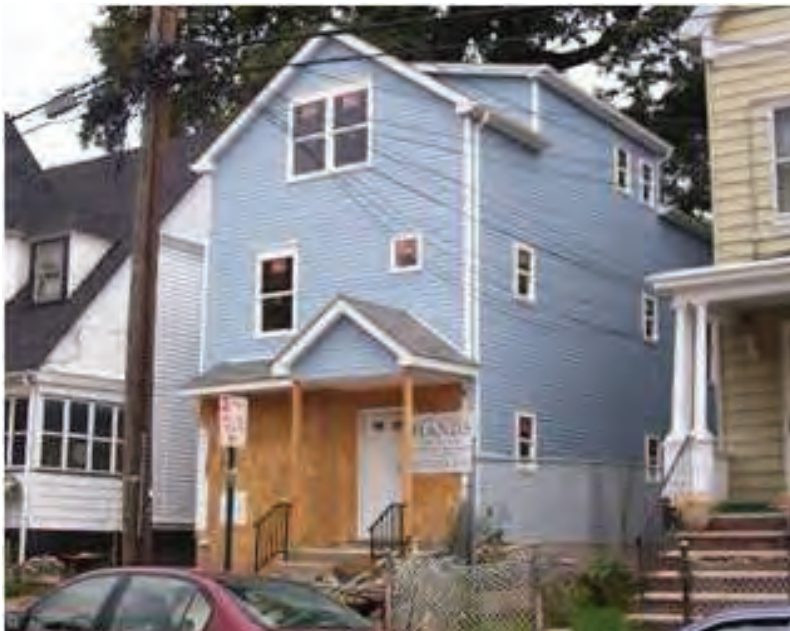
HANDS, Inc. housing rehabilitation examples in Orange, New Jersey
