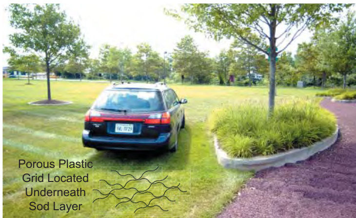
Left: Grassy pavers and gravel parking area, low-impact design techniques used to allow stormwater to percolate through the soil, directly recharging the groundwater supply, rather than quickly running into a stormwater sewer system and local streams. Source: E 2 Inc
