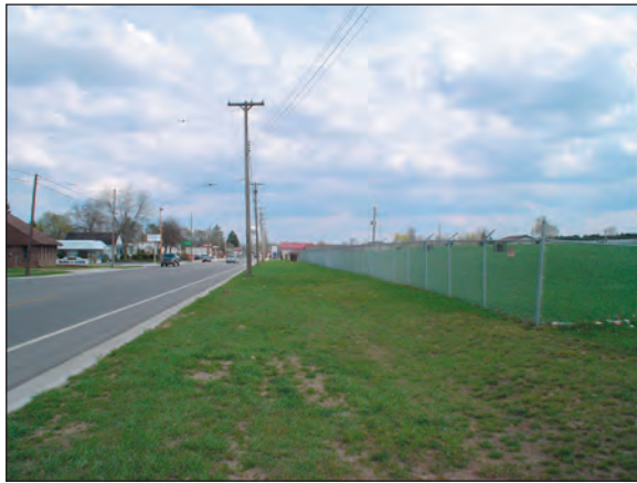
View along U.S. Highway 10 at the containment cell
