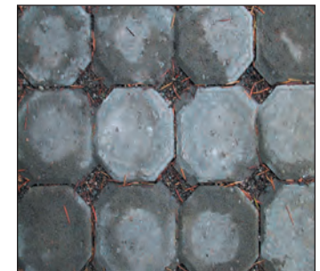
Top View of Porous Block Paving. Beveled corners allow for water to filter through to underlying soil
