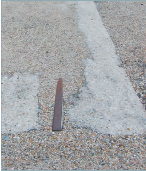
Exposed Rail Line in the Central Part of the Site
