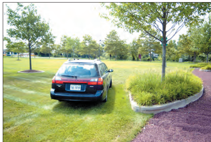
Grass 'Pavement', a Low Impact Design (LID) Technique: Underneath the grassy layer is a mesh of plastic honeycomb that is a durable parking surface for vehicles and is also porous enough for grass to grow and for rainwater to filter into underlying soil.
