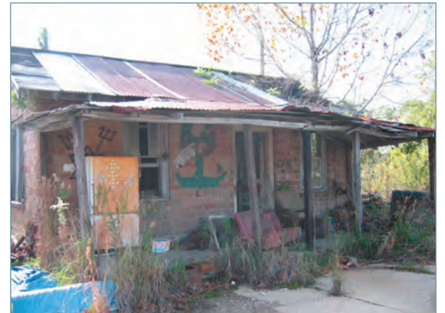
A Former Wood Treating Facility Office Building
