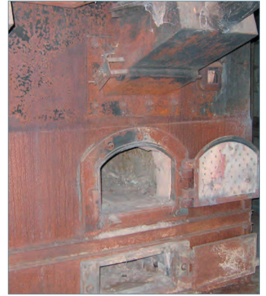
Remnant Boiler Room Machinery
