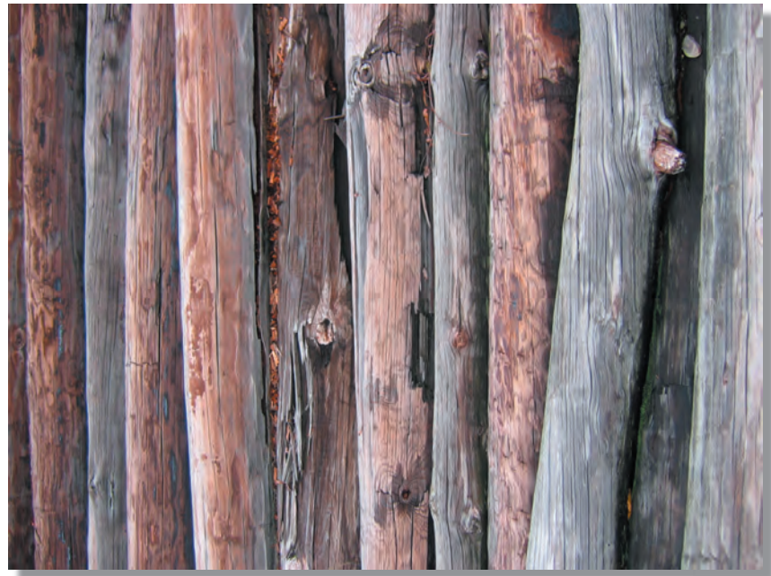
Remnant Stack of Treated Wood at the Picayune Wood Treating Superfund Site (2005)
