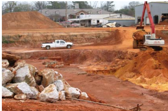
Remediation of contaminated soils at the site.
