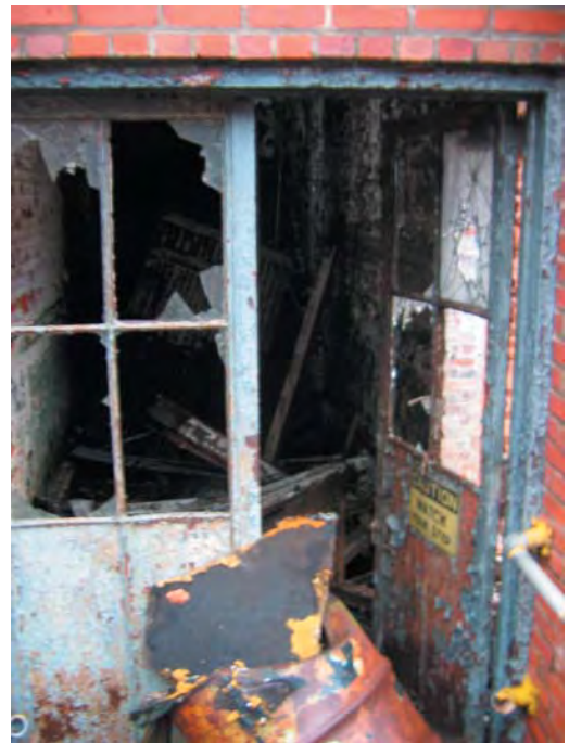
Doorway into Basement of Storage Buildings A, B, and C
