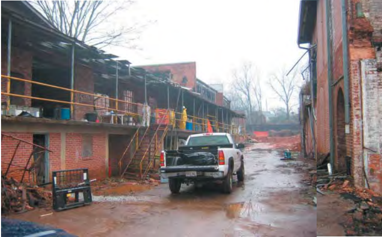
View of Buildings A, B, and C (on left)
