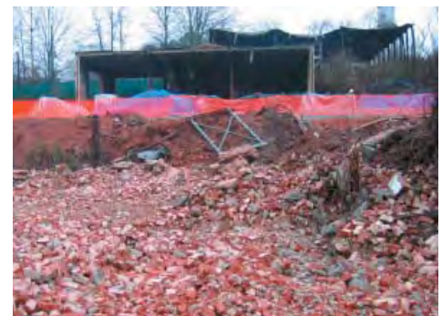
View of Brick Debris, Shed #4, (see photo below), and Pole Shed #5
