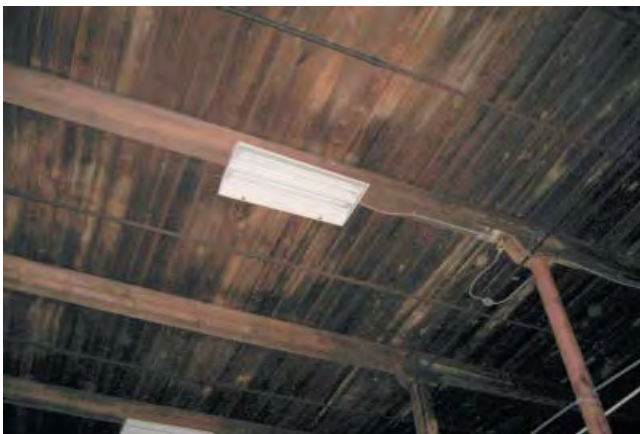
View of Wood Ceiling and Florescent Light Fixture in Building A
