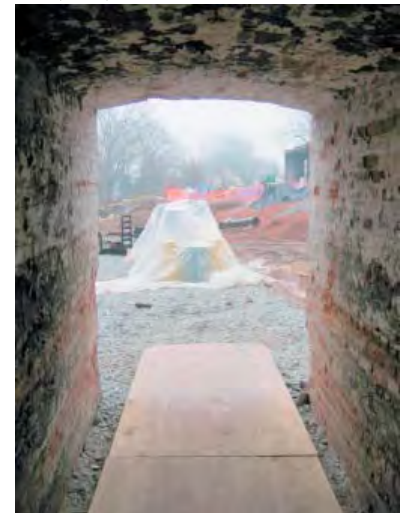
View of Former Main Mill Building Entry Way
