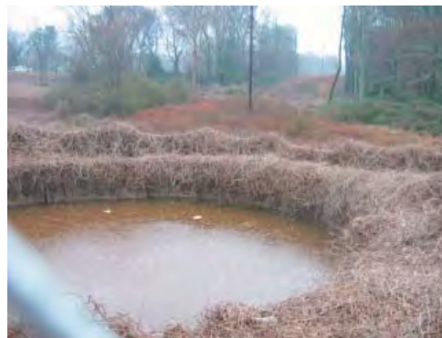
View of the Cistern
