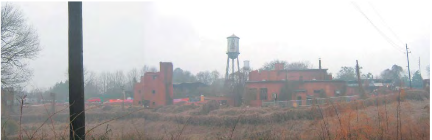
Eastern View of the Former Social Circle Cotton Mill, March 2007
