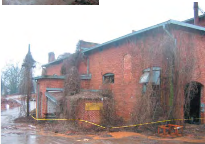
View of the Eastern Face of the Former Main Mill Building
