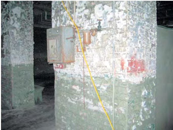
Brick Column with Peeling Paint
