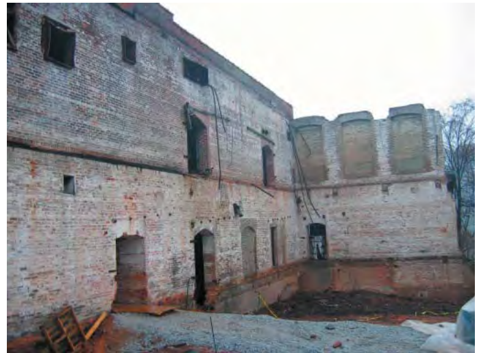
View of the Southern Face of the Former Main Mill Building
