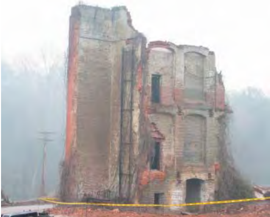
View of Remnant Mill Building #3, Western Face
