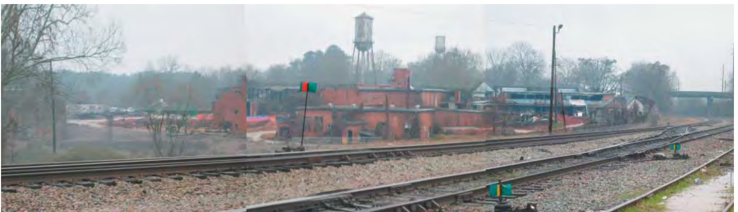
View of the Former Social Circle Cotton Mill and CSX Rail Line, Taken from the Historic Train Depot Located Northeast of the Site
