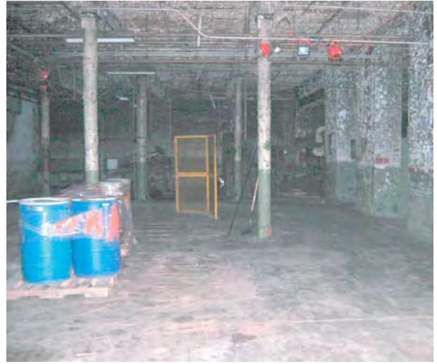
View of Former Main Mill Building Interior
