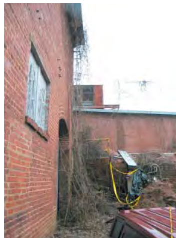
View of the Northern Face of the Former Main Mill Building
