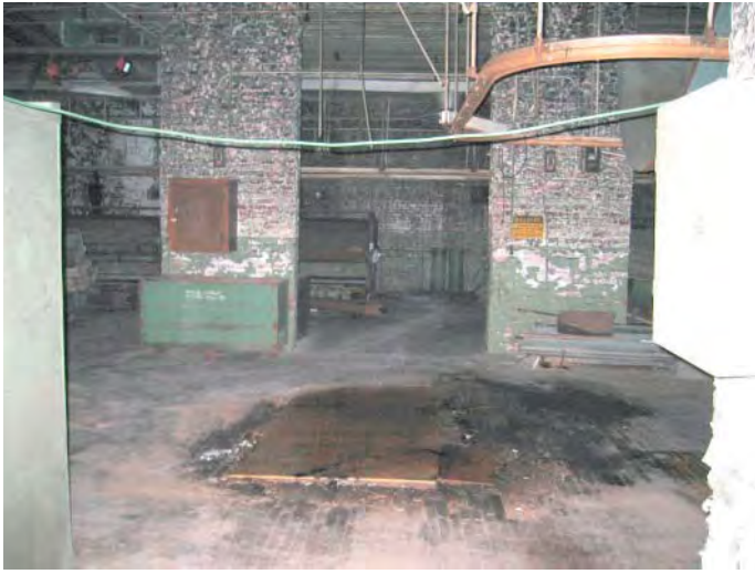
View of Former Main Mill Building Interior
