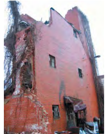
View of Remnant Mill Building #3, Eastern Face
