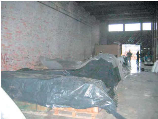
View of Building B's Interior, Looking Towards the Entry Way
