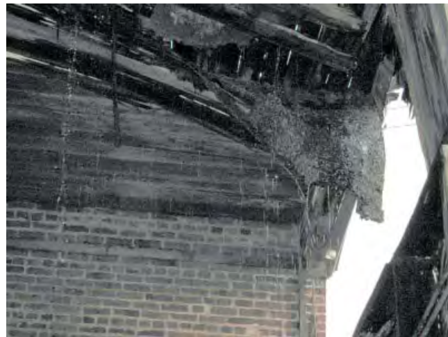
View of Wood Ceiling and Roof Damage in Building A
