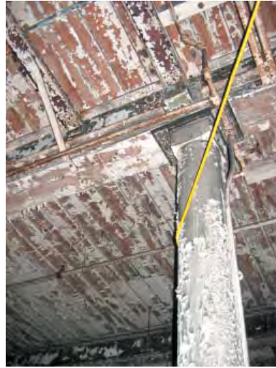
View of Ceiling and Steel Post
