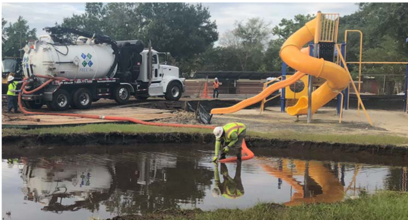
Picture of stormwater being removed with vacuum truck
