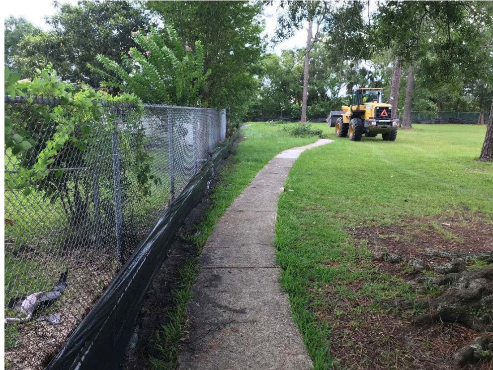
Silt fence placed around excavation area
