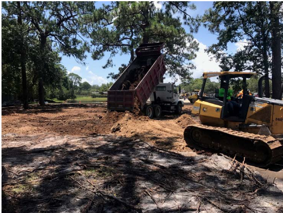
Backfilling operations
