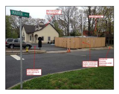
Photos of ERH systems installed in occupied residential and dense urban settings.
