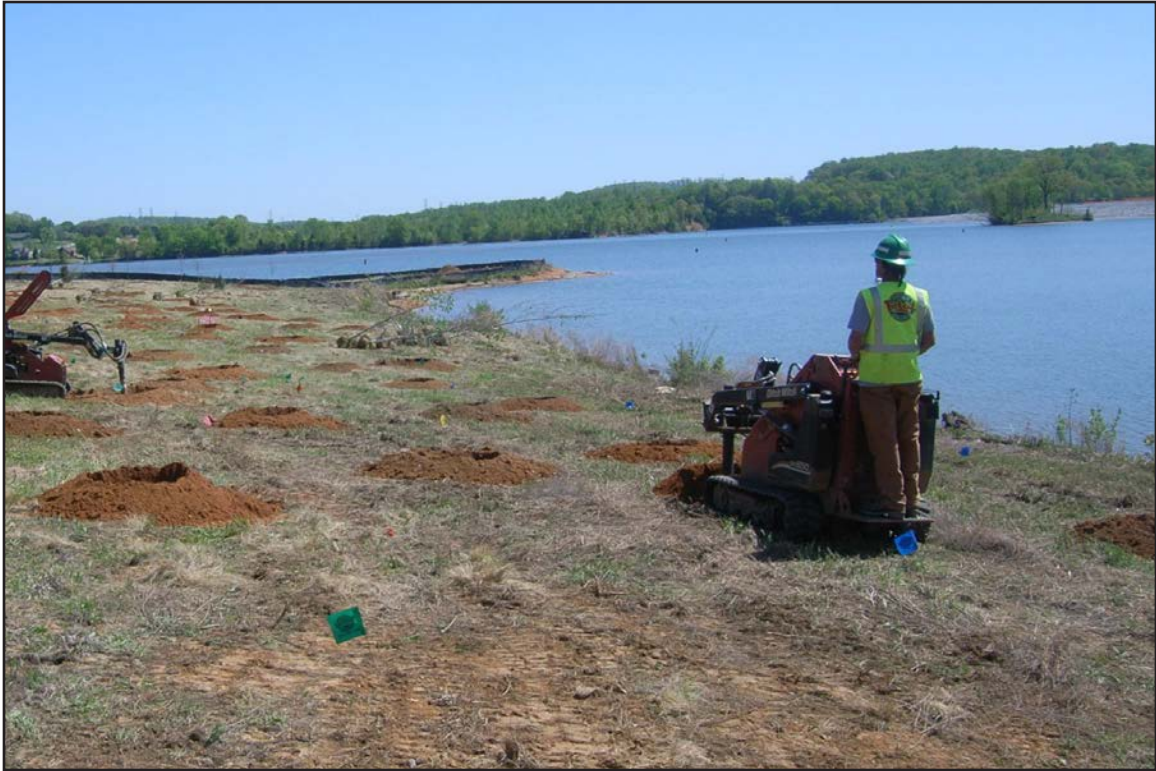
5A – Plantings - Augering holes for trees. April 23, 2014.
