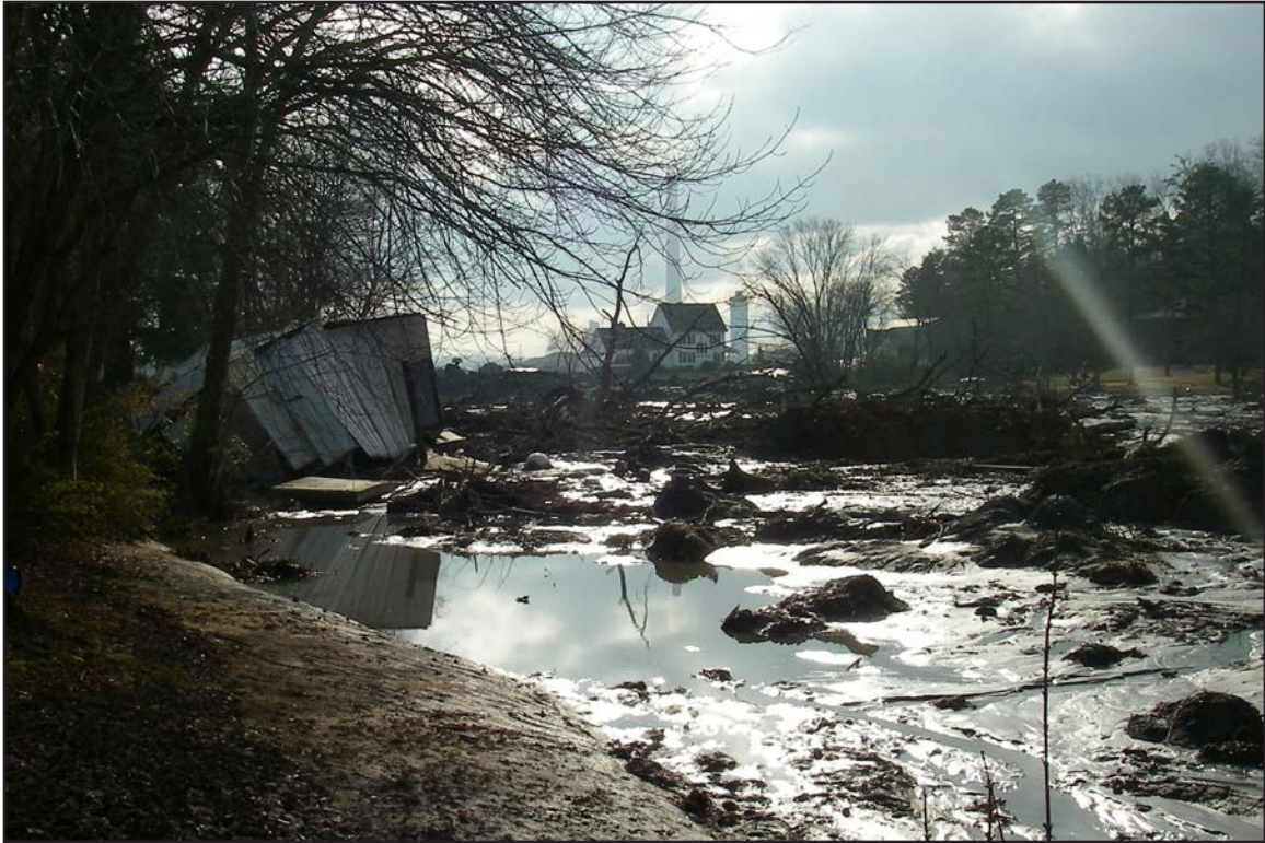
1E – East Embayment following SPEER Non-Time-Critical Removal Action. July 29, 2014.
