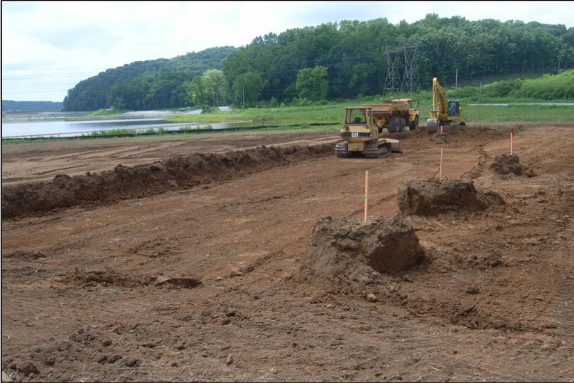
10A – Wetlands construction - Grading for wetland in the North Embayment. June 10, 2014.
