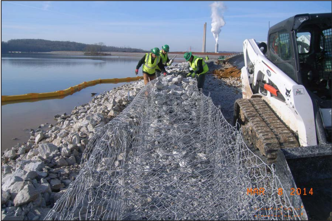
11A – Vegetative slope stabilization - Placing gabions. March 8, 2014.
