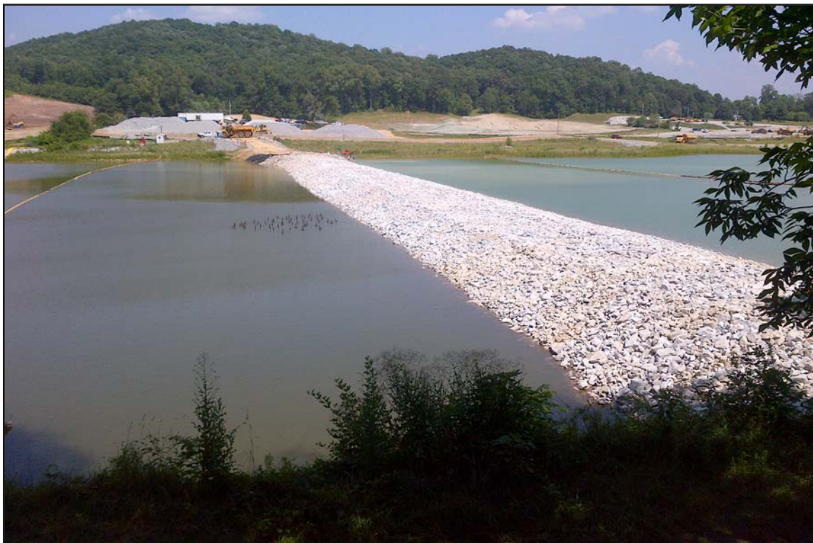
3B – North Embayment riprap armoring of the North Berm dike. July 7, 2014.
