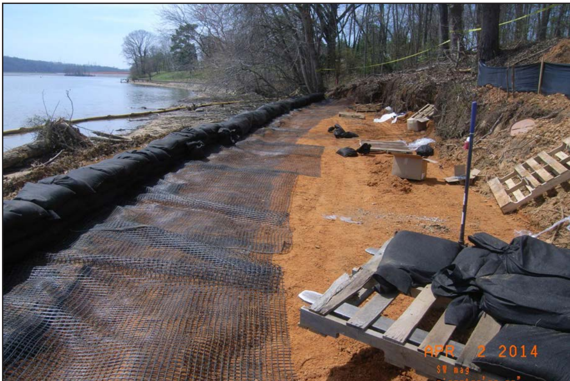
11B – Vegetative slope stabilization - Placing geogrid tiebacks. April 2, 2014.
