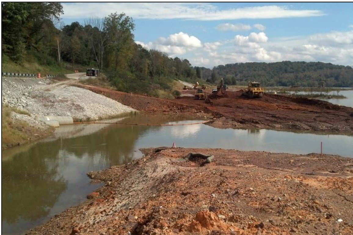
4B – Grading of clean water ditch - Filling in Middle Embayment. October 20, 2014.
