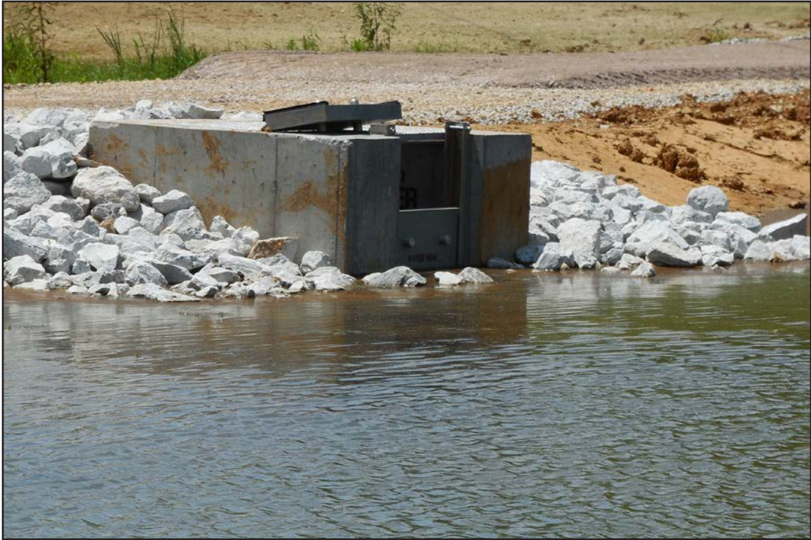
13A – Weir 1 at the transitional wetlands in the North Embayment. July 29, 2014.
