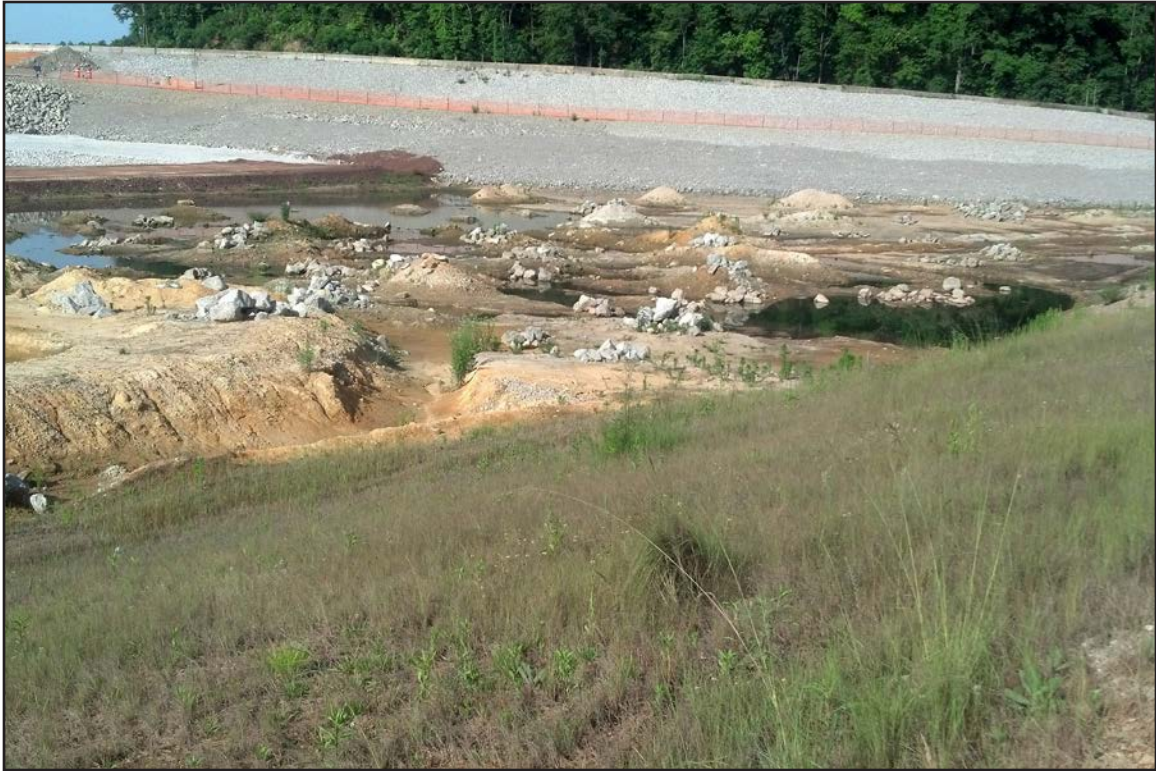
2A – Middle Embayment before inundation with rock piles as fish habitat. May 24, 2014.
