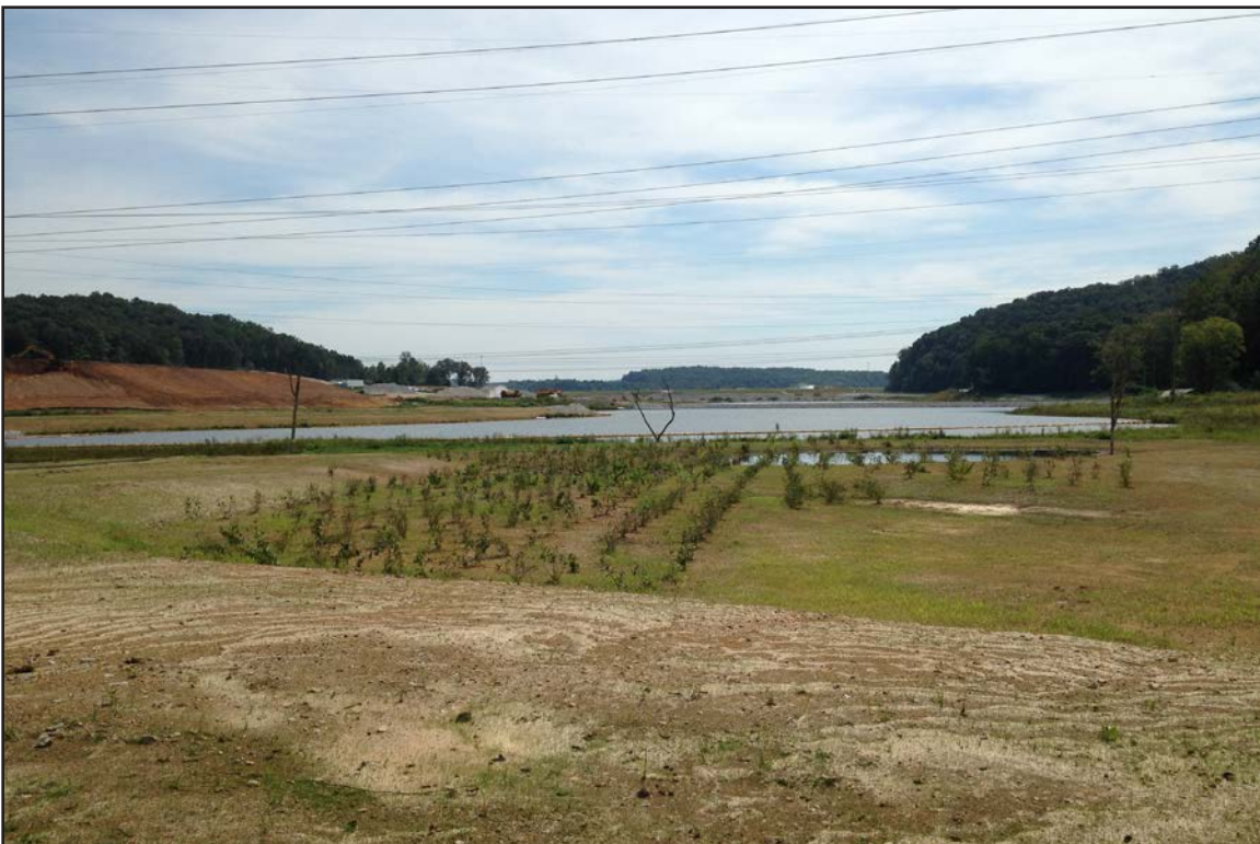
10B – Wetland construction - Completed wetland in the North Embayment. September 18, 2014.
