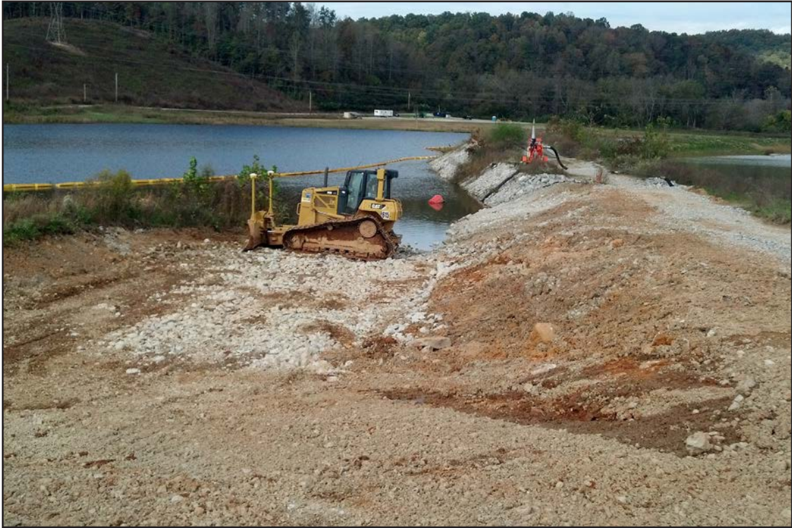
4A – Grading of clean water ditch - Filling in North Embayment. October 20, 2014.
