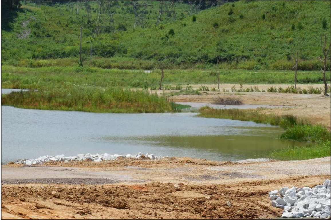
3A – North Embayment grading of transitional wetlands area. July 29, 2014.
