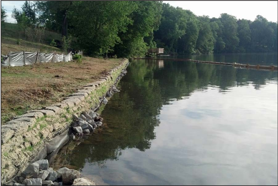
12A – Vegetative slope stabilization - Emory River shoreline. May 24, 2014.
