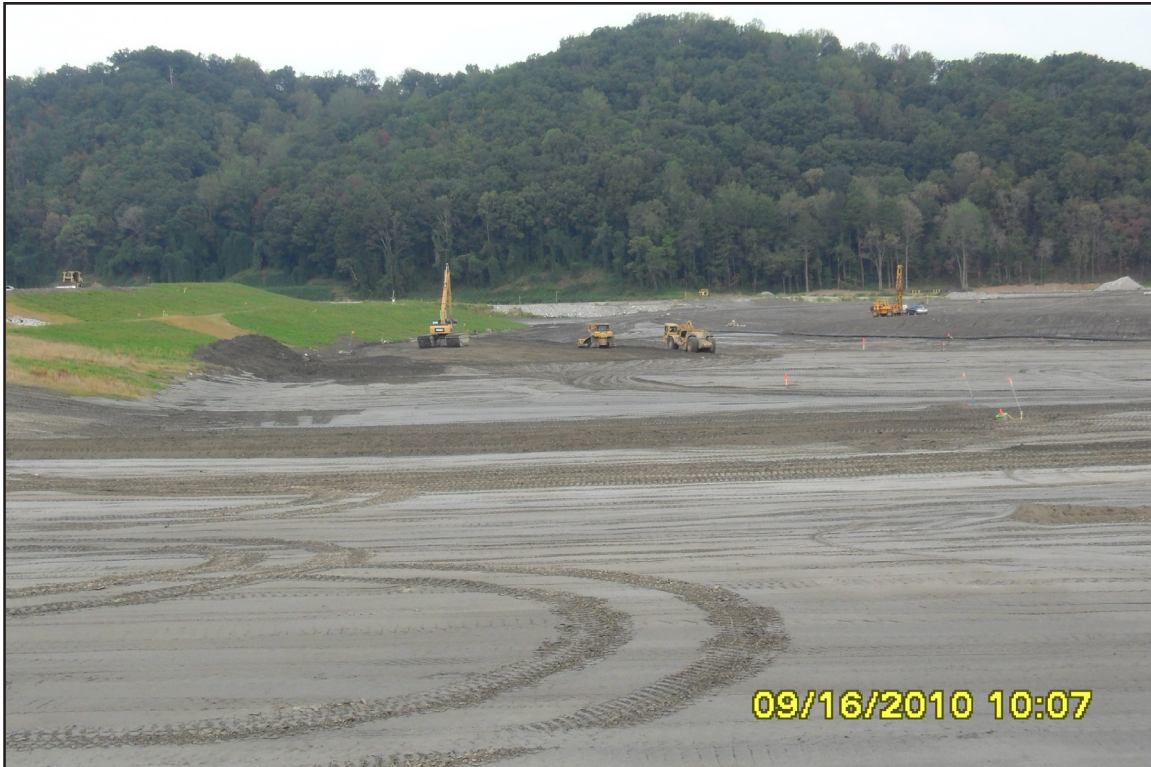
18A – Ash Stacking: Stacking in the Dredge Cell during the subgrade recontouring phase. September 16, 2010.
