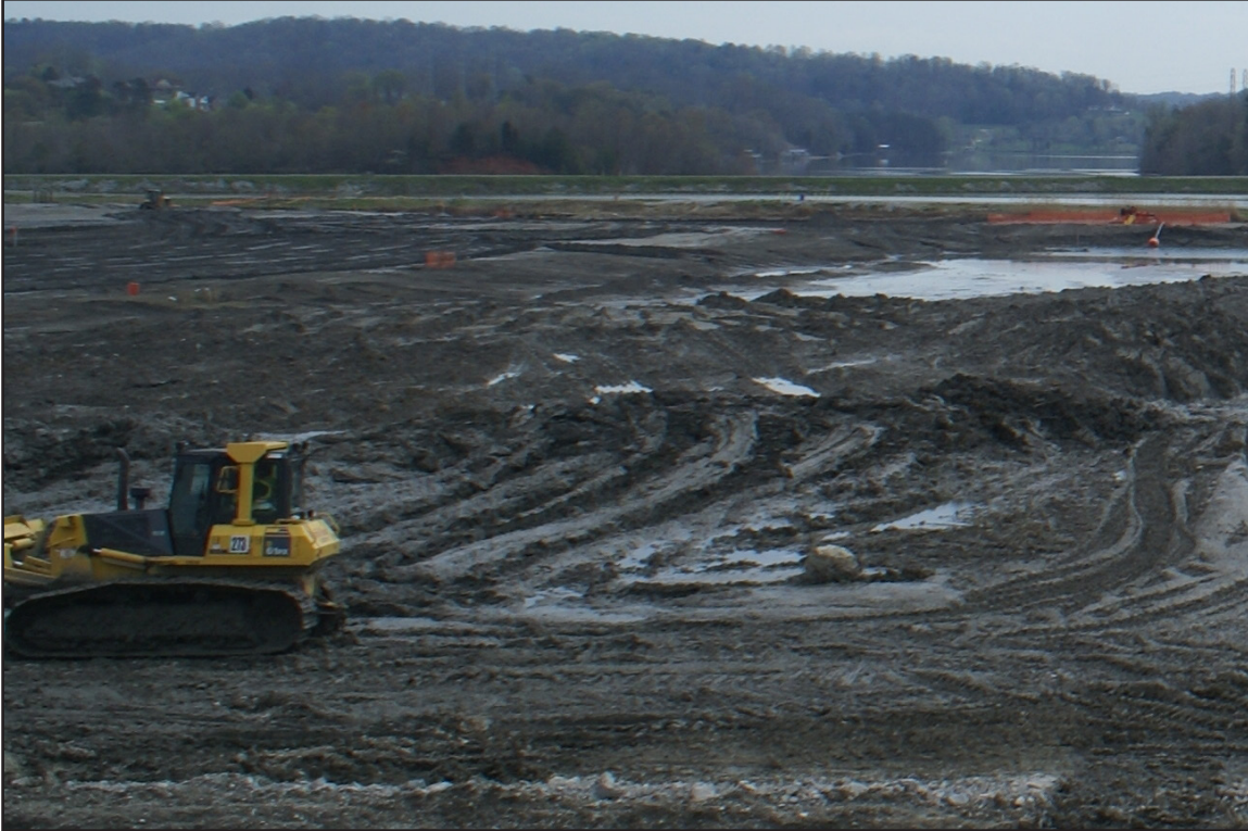
20A – Ash Stacking: Stacking in the Ash Pond during the subgrade recontouring phase. March 18, 2012.
