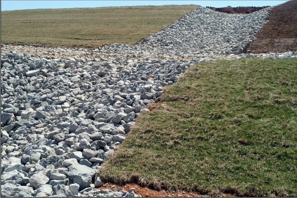
44A – Cap and Closure: Riprap-lined downslope flumes of completed cap and cover. March 20, 2014.
