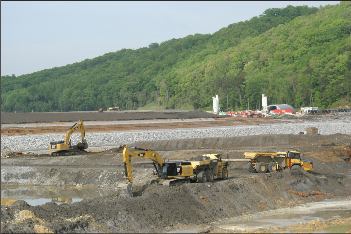
9A – Ash Removal: Excavating ash from the Middle Embayment using trackhoes and articulated dump trucks. April 30, 2013.
