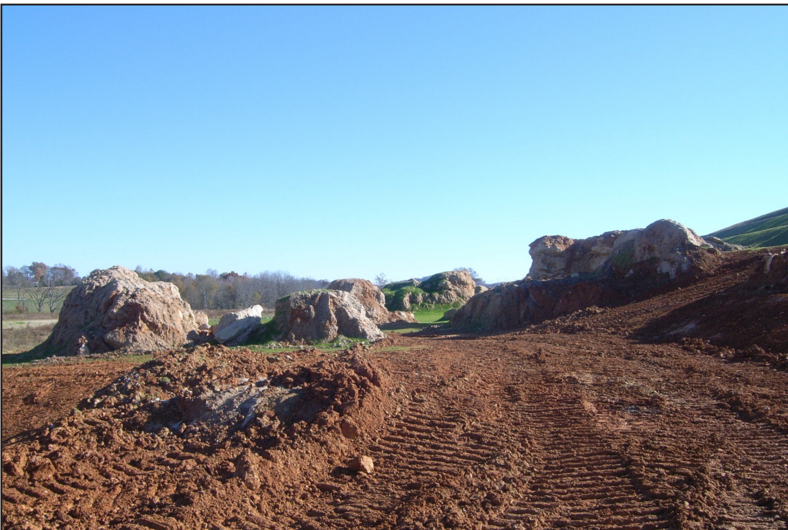
46B – Borrow Area: Rock outcrops encountered in borrow pits. November 8, 2013.
