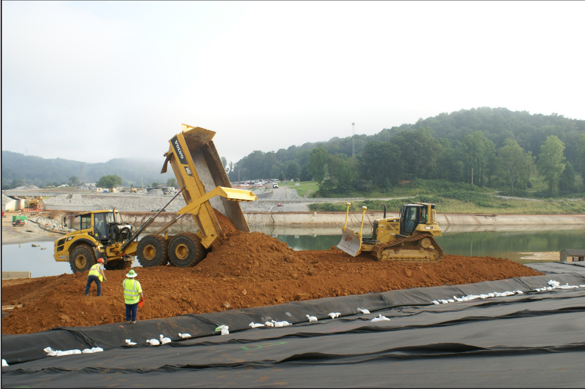
42A – Cap and Closure: P&J placing cap soil over the geocomposite. July 18, 2013.
