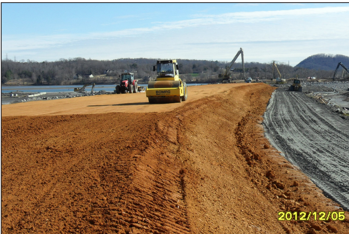
37B – Perimeter Containment: Placing clay as embankment for construction of the perimeter containment berm. December 5, 2012.
