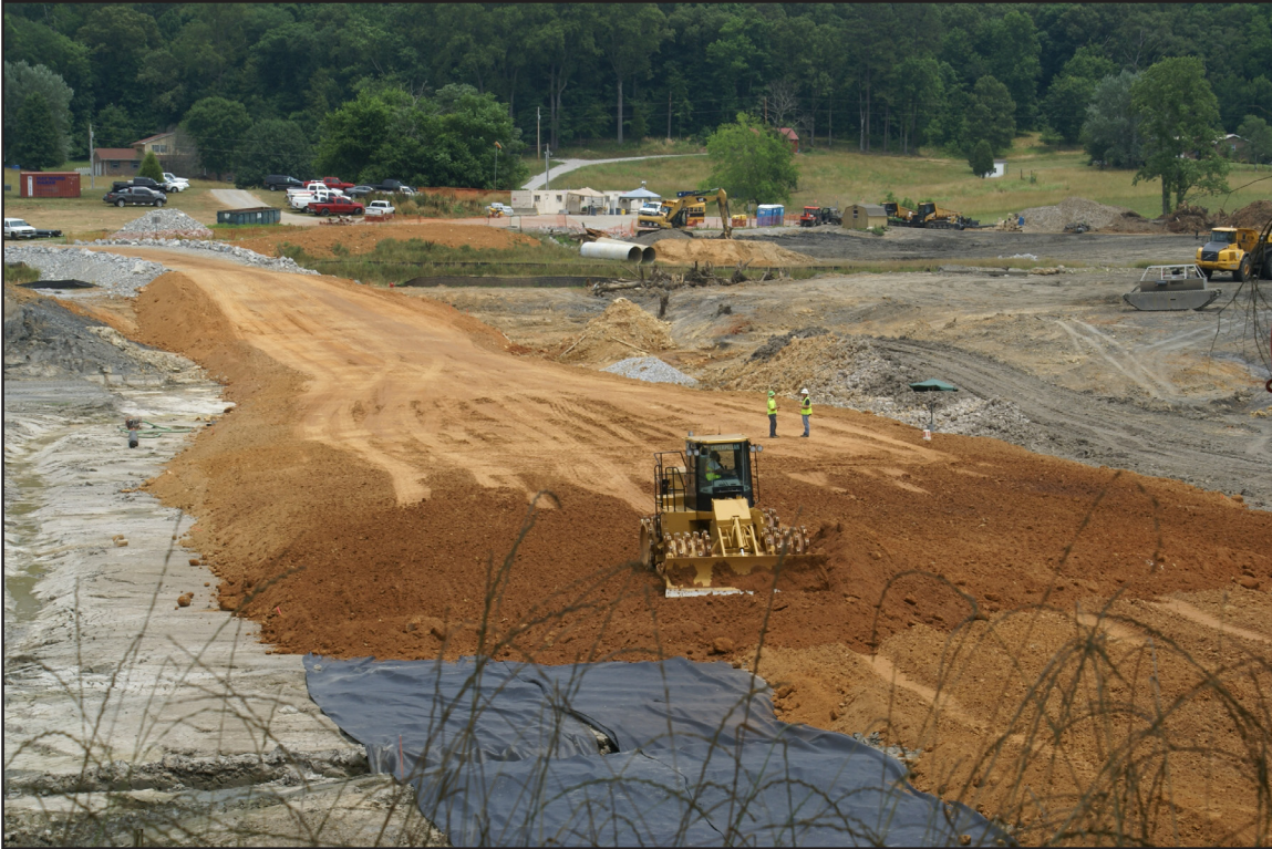
8A – Ash Removal: Construction of the North Berm through the North Embayment. June 13, 2011.
