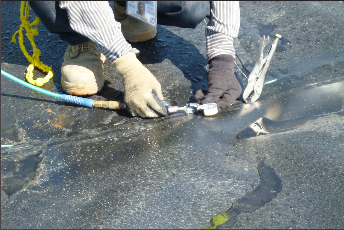
40A – Cap and Closure: CCS field seam testing for quality control of the flexible membrane liner (FML). September 30, 2013.
