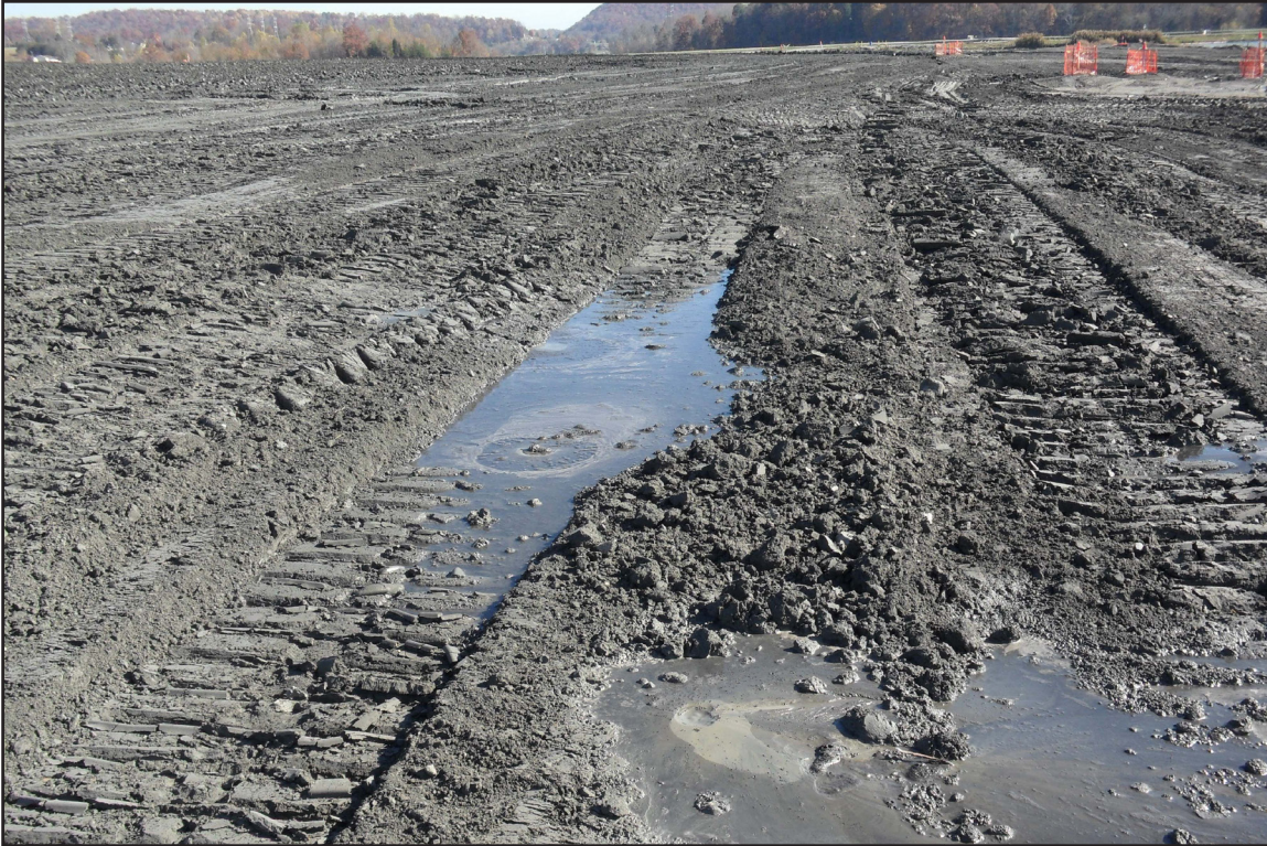
22A – Ash Stacking: Mud boils inducing wet subgrade conditions during ash stacking in the Lateral Expansion. November 8, 2011.
