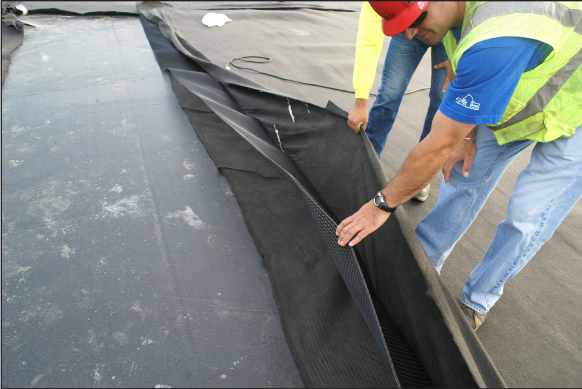
41A – Cap and Closure: Geocomposite drainage layer (geonet between layers of geotextile). July 18, 2013.
