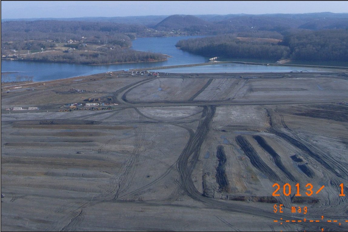
16A – Ash Processing: Using windrows in the Central Dredge Cell area. January 3, 2013.
