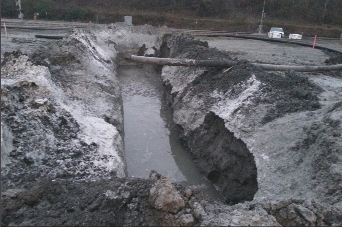
31A – PWS: Slurry trench overnight drop in slurry level to several feet below ground surface. December 4, 2013.
