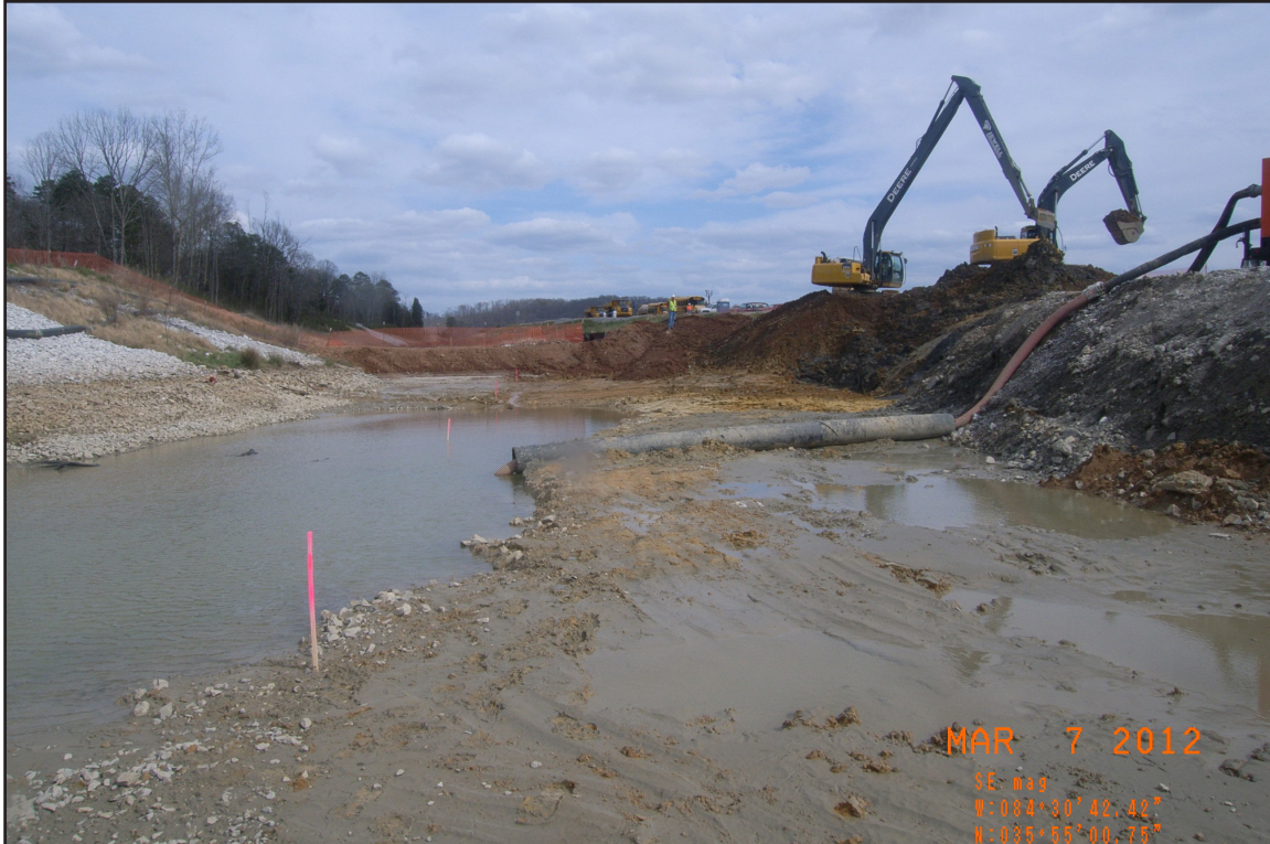
10A – Ash Removal: Excavating ash from the Clean Water Ditch in the Middle Embayment prior to rebuilding the ditch. March 7, 2012.
