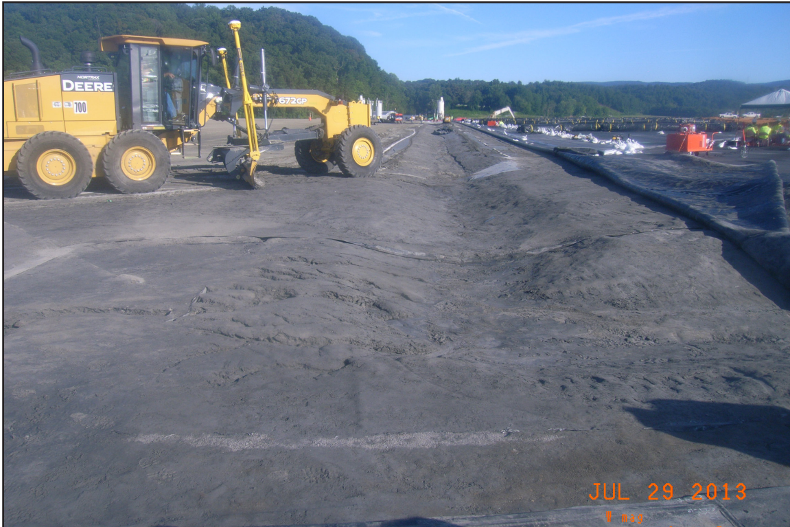
38A – Cap and Closure: Preparing subgrade using GPS grader. July 29, 2013.
