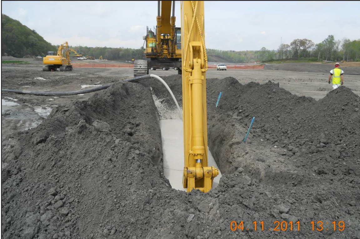
26A – PWS: Slurry trench excavation. April 11, 2011.
