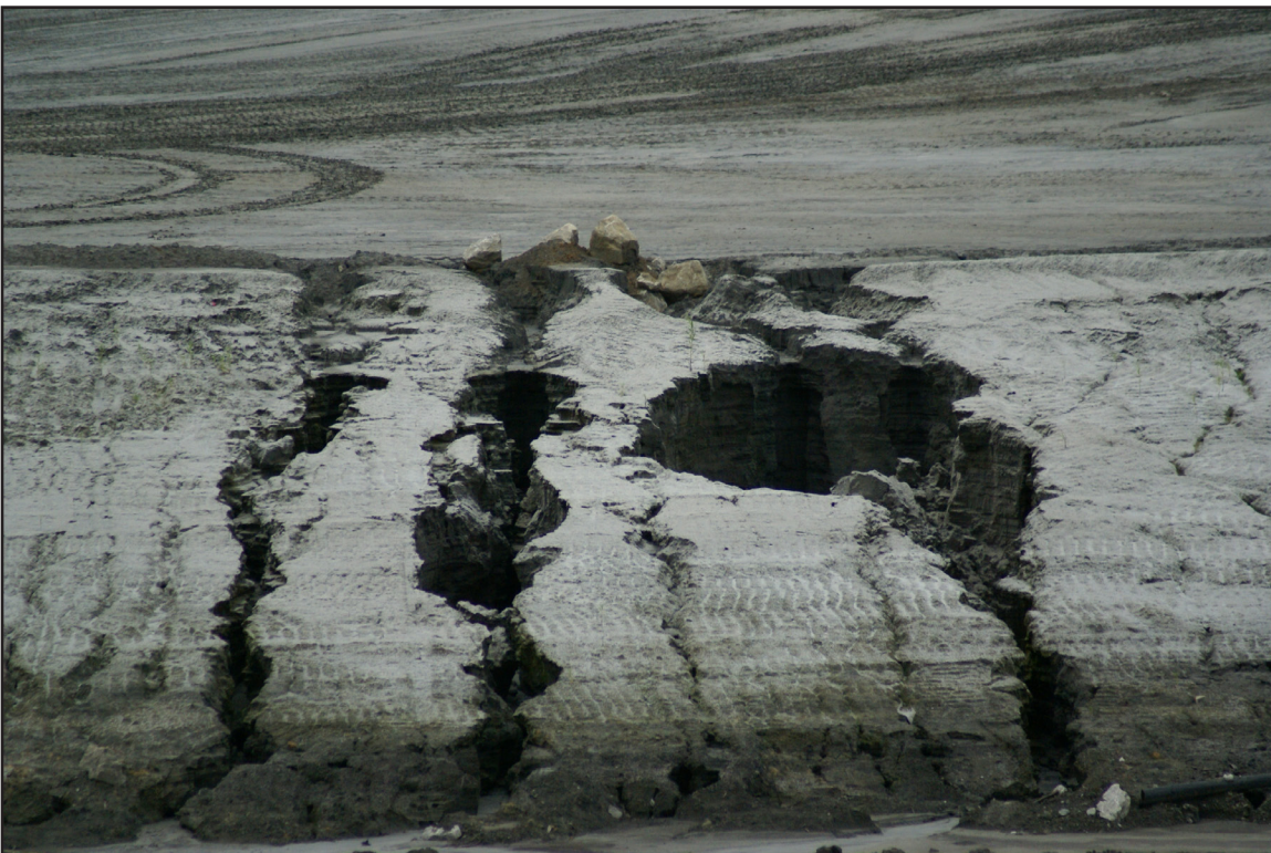
21B – Ash Stacking: Erosion damage to edge of ash stack following storm event. August 12, 2013.
