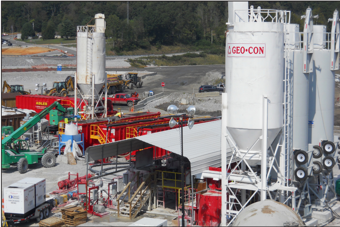
28A – PWS: Batch Plant used to supply cement slag-bentonite slurry for the PWS construction. May 23, 2011.
