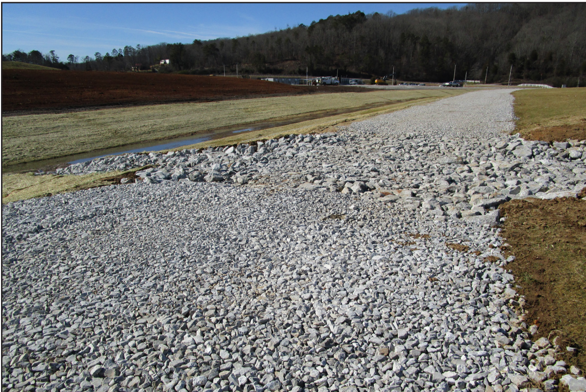
44B – Cap and Closure: Riprap at low water crossing of perimeter road. January 28, 2015.
