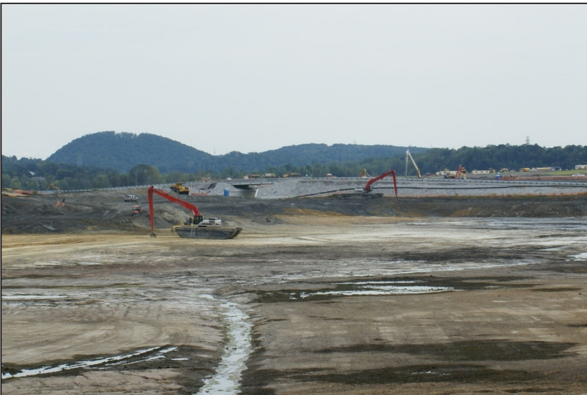
7B – Ash Removal: Bottom of the North Embayment following ash removal. September 19, 2011.
