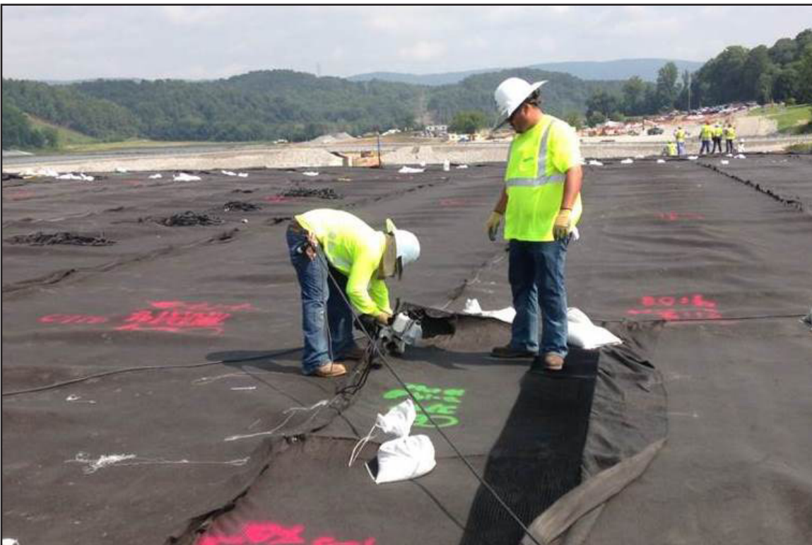
41B – Cap and Closure: CCS sewing seam of geocomposite drainage layer. September 14, 2013.
