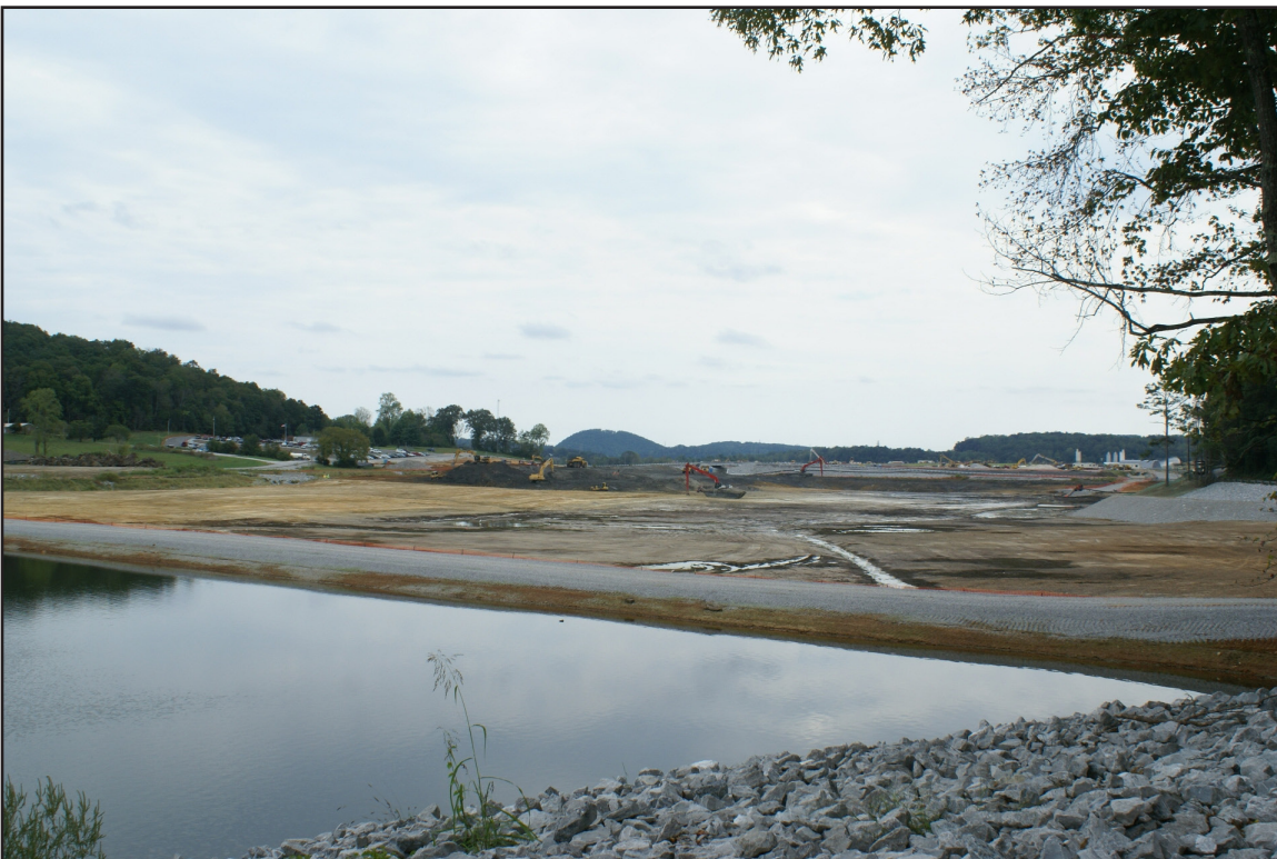
8B – Ash Removal: Completed North Berm diverting stormwater from the lower half of the North Embayment. September 18, 2011.
