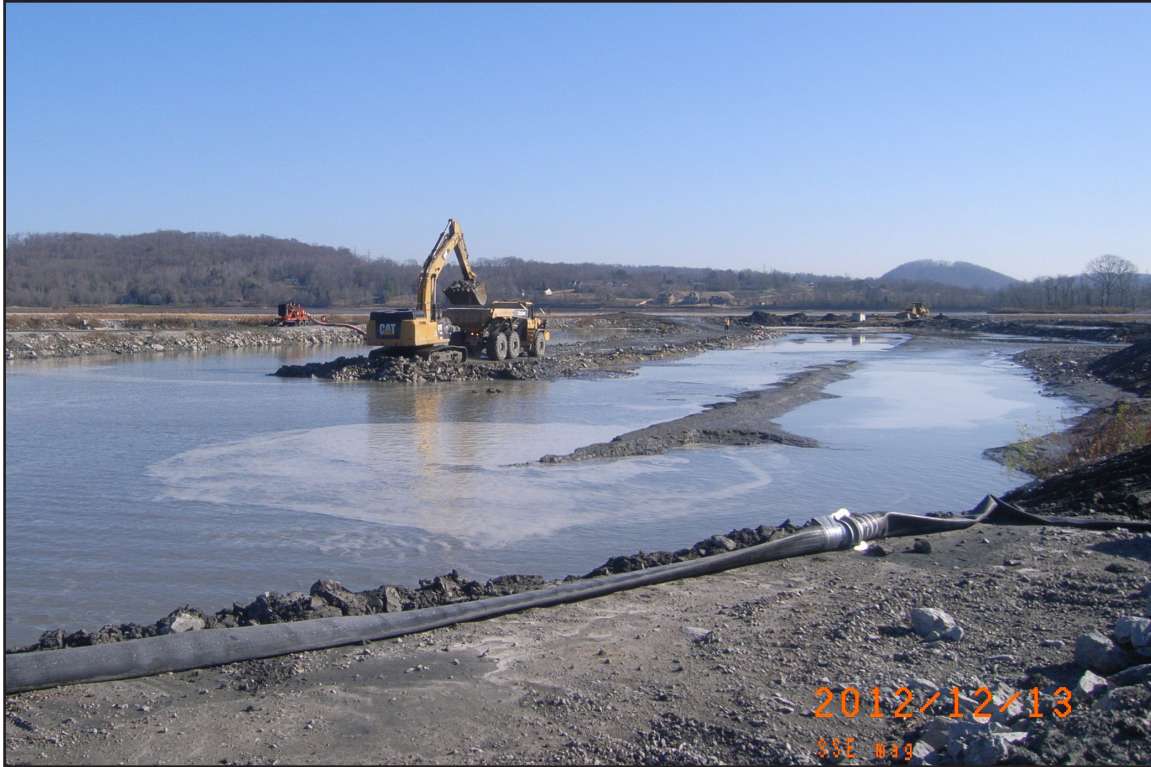
11A – Ash Removal: Excavating ash and removing finger dikes from the Sediment Basin. December 13, 2012.
