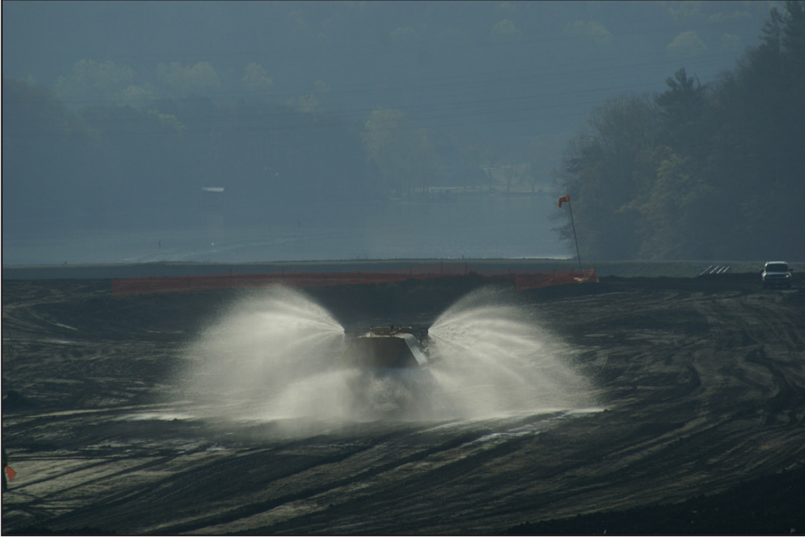
49A – Dust and Erosion Control: Holleman spraying haul roads with water to minimize dust. April 8, 2013.
