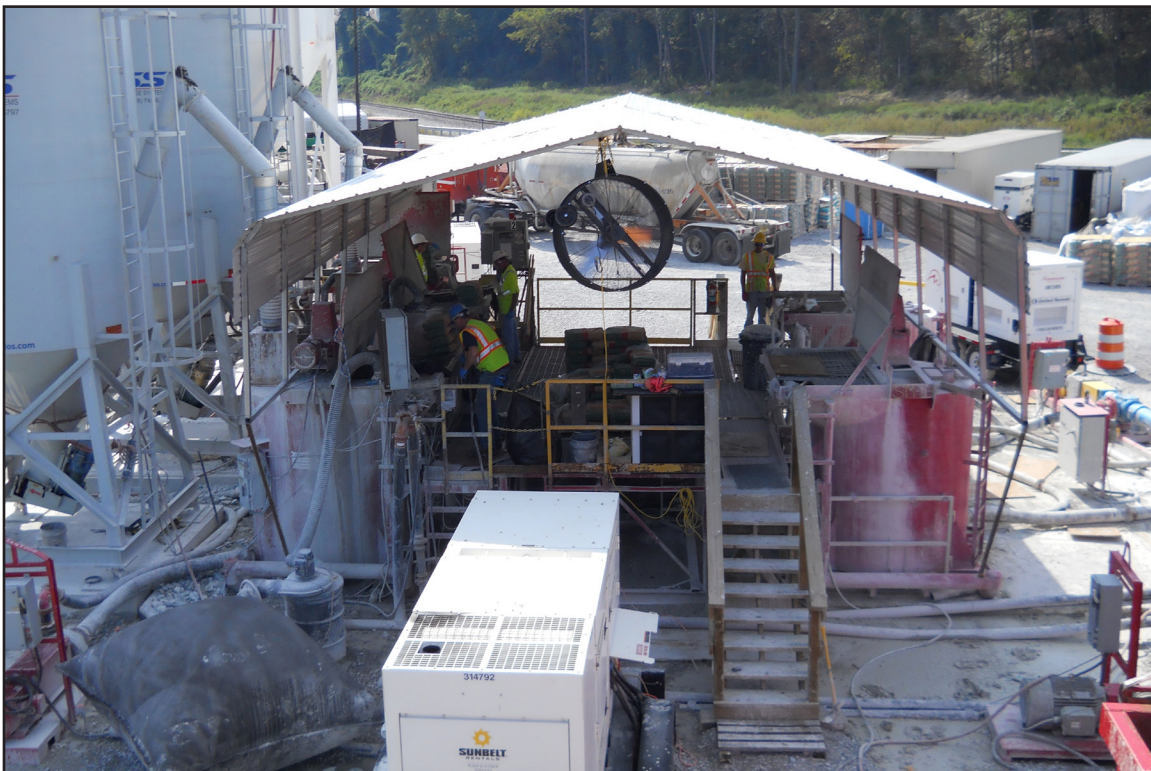
28B – PWS: Batch Plant used to supply cement slag-bentonite slurry for the PWS construction. April 13, 2011.
