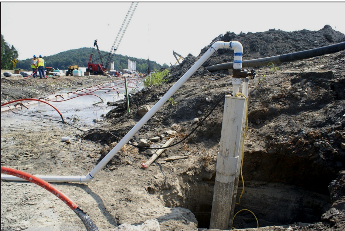
32B – PWS: Slurry trench construction stabilized using Griffin dewatering system (deep wells and shallow well points). June 14, 2012.
