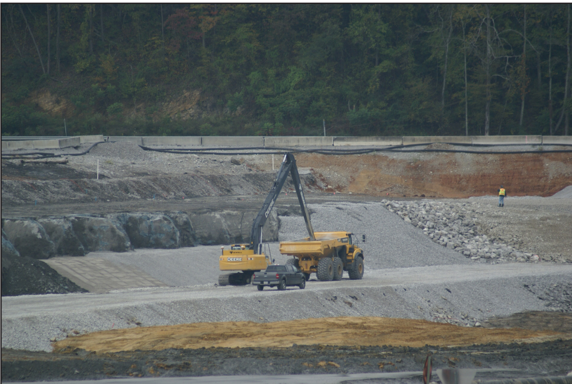
35B – Perimeter Containment: Placing No. 02 stone as rock buttress along Segment 8 of the perimeter wall. October 09, 2012.
