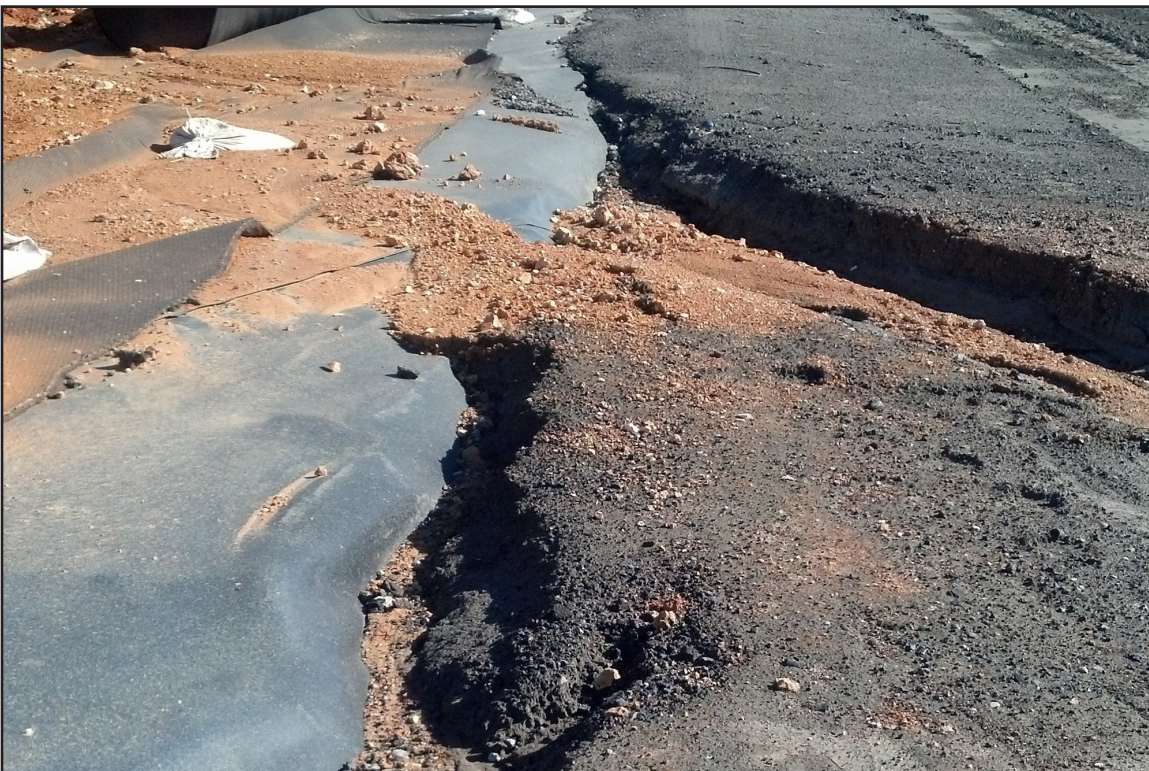
40B – Cap and Closure: Edge of FML installed in an anchor trench to prevent erosion undermining of the FML. January 20, 2014.
