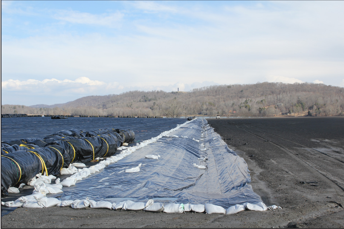
47A – Stormwater Management: Ditch lined with plastic tarp for erosion control. August 10, 2013.
