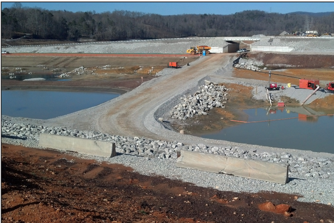
10B – Ash Removal: Haul roads traversing the Middle Embayment during the Non-Time-Critical Removal Action. December 31, 2013.
