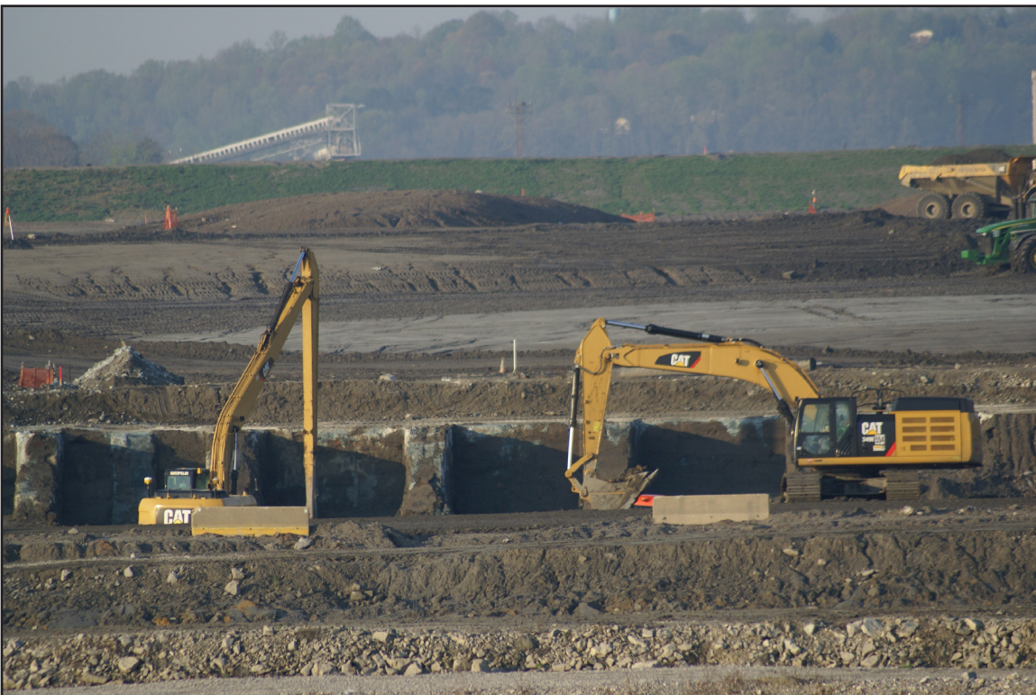
27B – PWS: Cured walls exposed at the buttress along the Middle Embayment. March 20, 2012.
