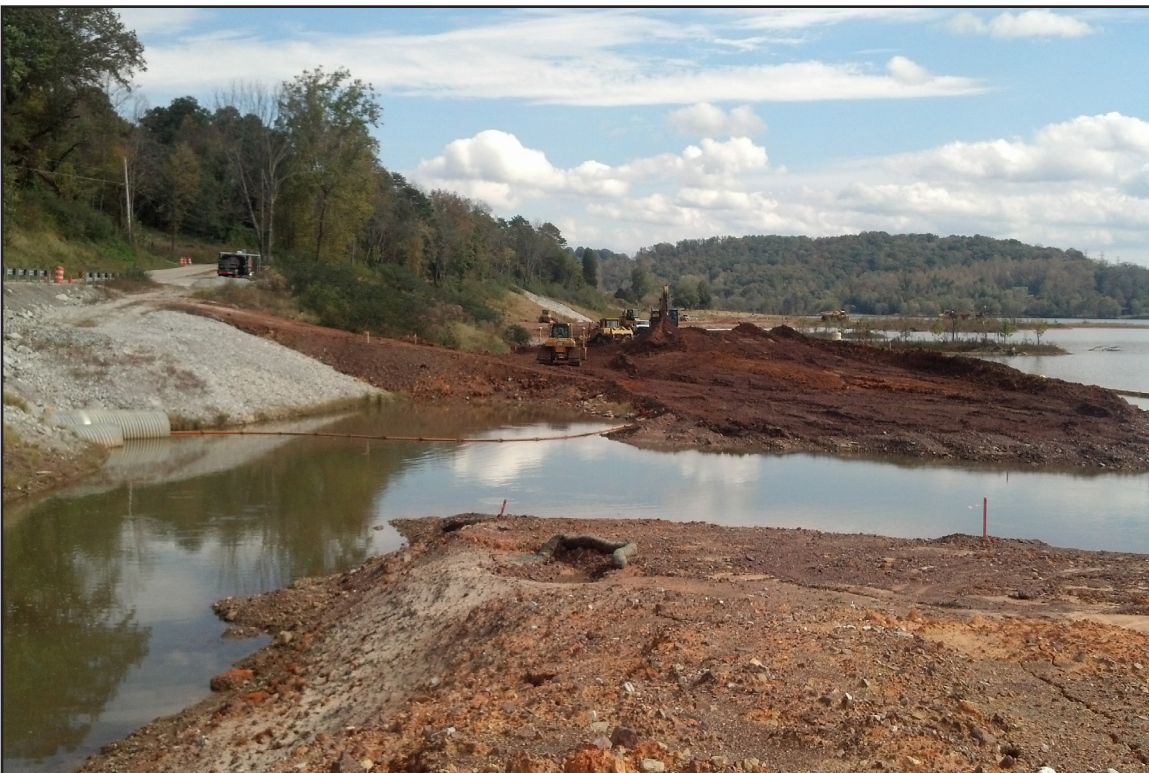
13B – Ash Removal: Removal of the Clean Water Ditch from operation by filling with borrow soil. October 20, 2014.
