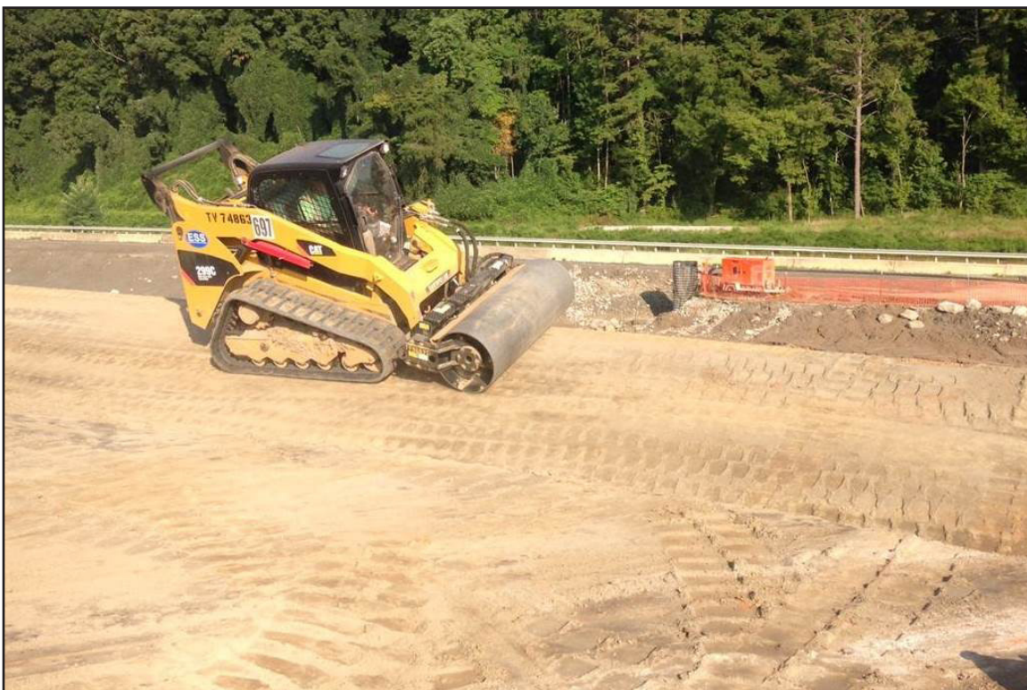
38B – Cap and Closure: Preparing subgrade using skid steer roller preparing subgrade for ditch at top of perimeter slope. August 2013.
