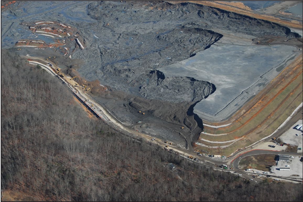
2A – Oblique of the failed Dredge Cell after release (viewing from the southwest). January 8, 2009.
