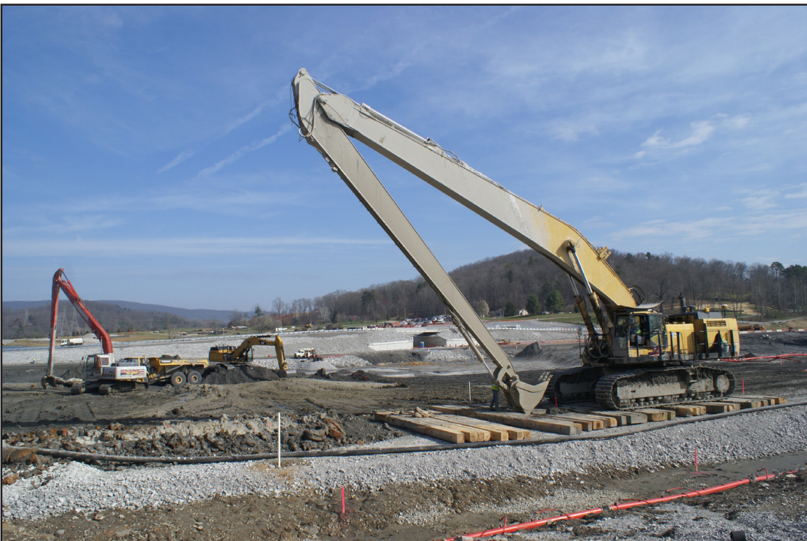
31B – PWS: Slurry trench construction platform stabilized with rock surfacing on inboard side of wall. March 6 2012.
