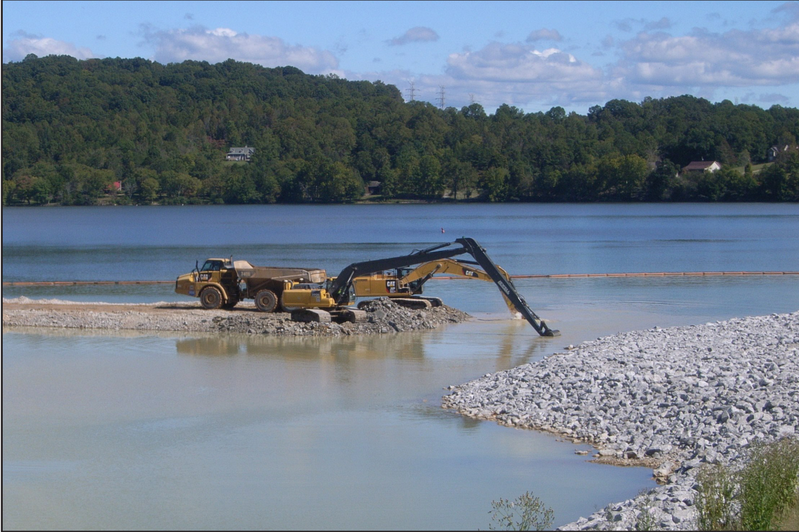
13A – Ash Removal: Removal of Dike 3 and flooding of the Middle Embayment. September 25, 2014.
