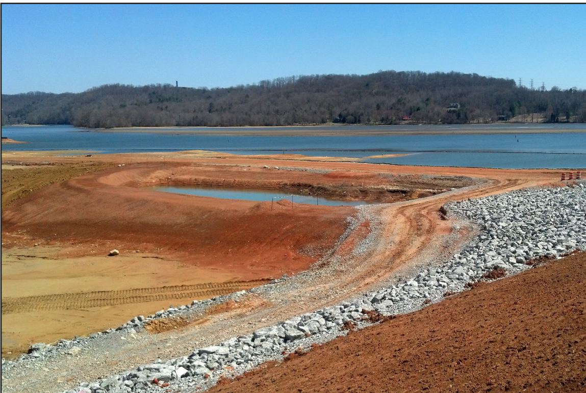
12B – Ash Removal: Retaining pond used to reduce seepage through a riprap section of Dike 3. March 20, 2014
