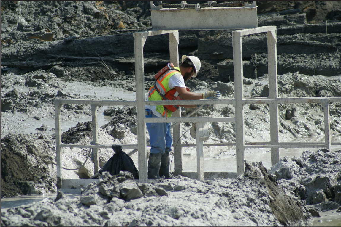
27A – PWS: Quality control of slurry trench included measuring trench depth and obtaining grab samples. August 30, 2011.
