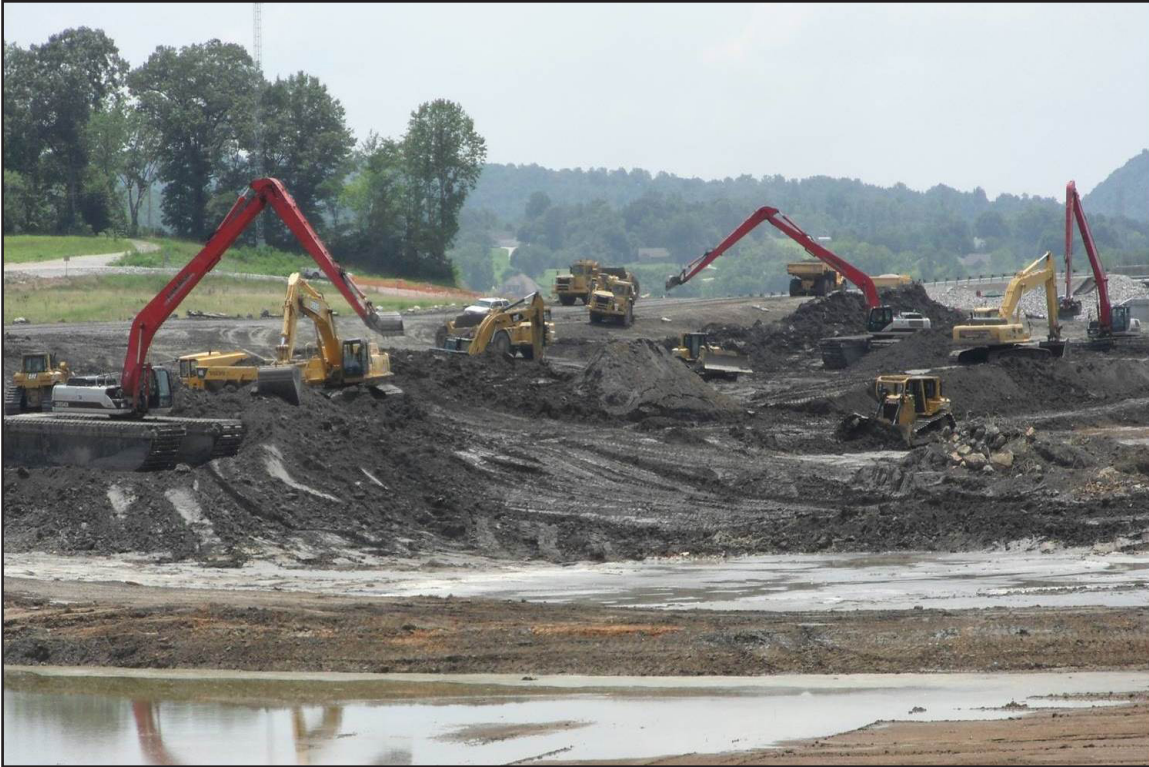
7A – Ash Removal: Excavating ash from the North Embayment using amphibious long-reach backhoe excavators and trackhoes. August 16, 2011.
