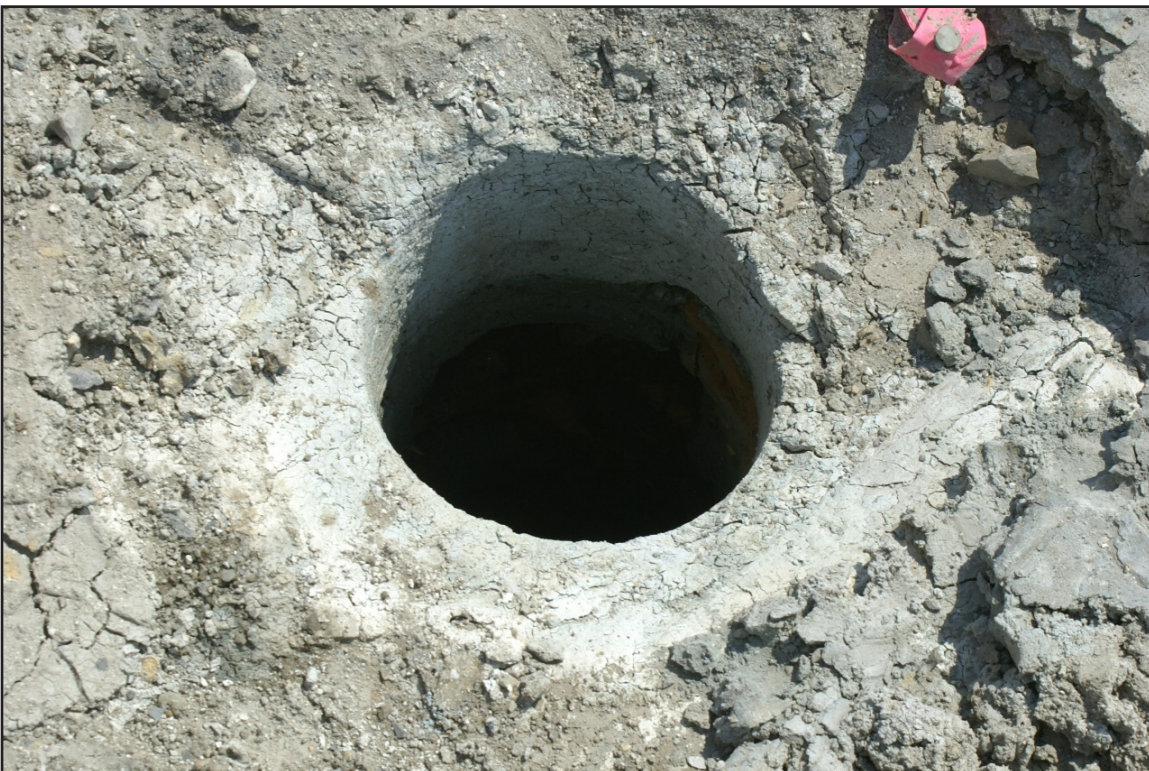
33B – PWS: Predrilled hole in wall for mitigation of wall defects. August 30, 2011.
