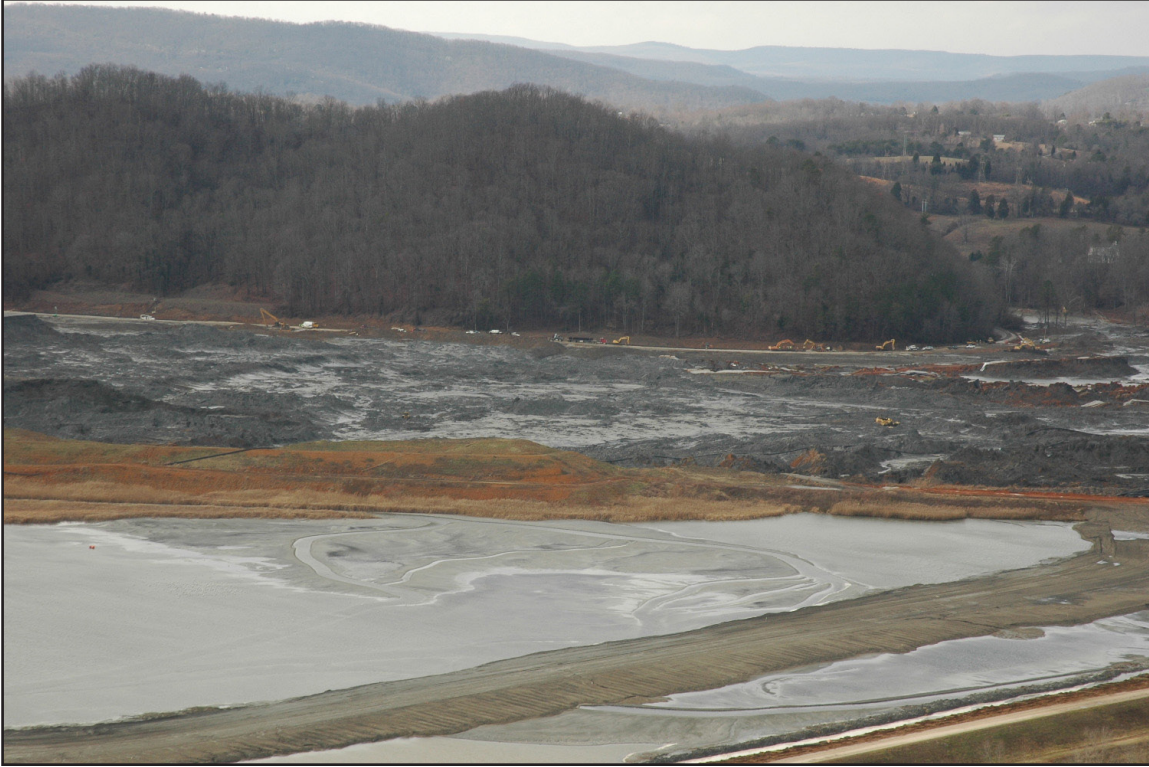
4A – Oblique of the failed Dredge Cell after release (viewing from the east). January 7, 2009.
