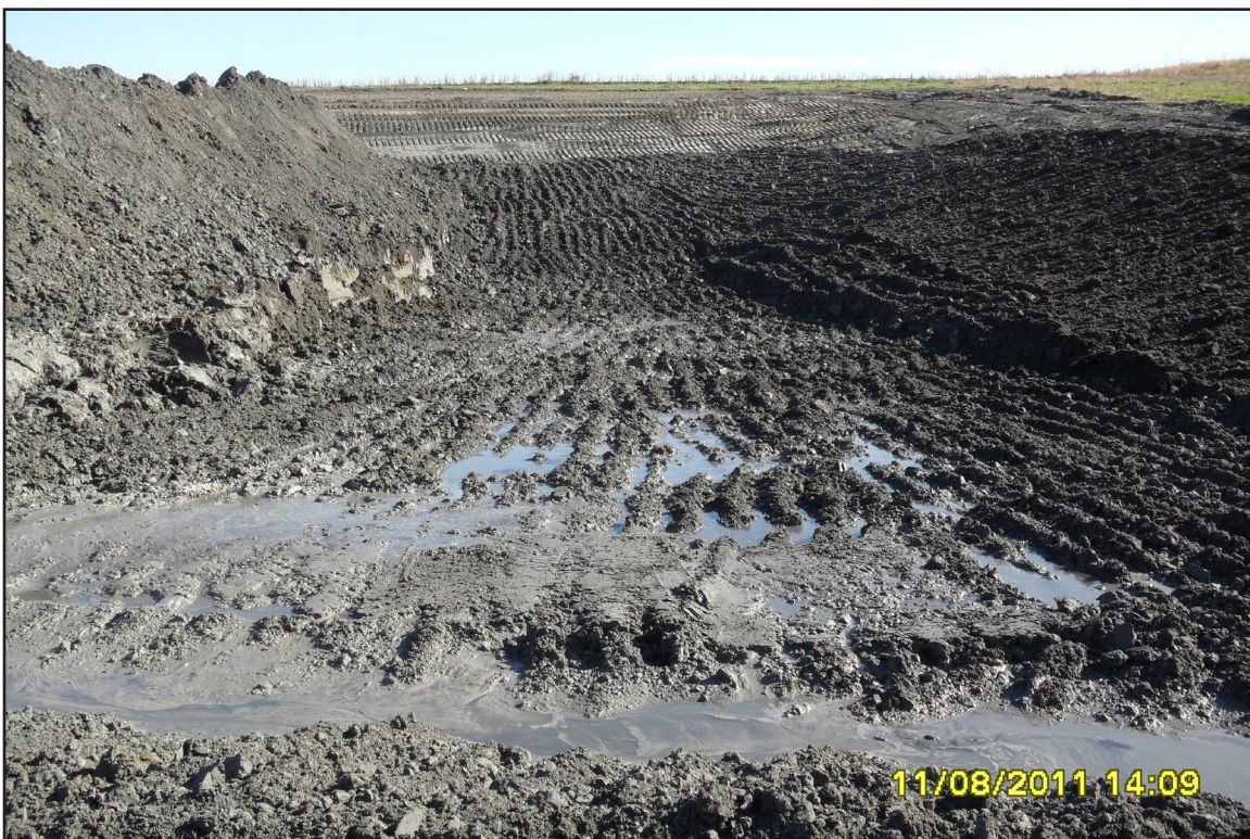
22B – Ash Stacking: Repair of mud boils by excavation of wet subgrade for construction of French drains. November 8, 2011.
