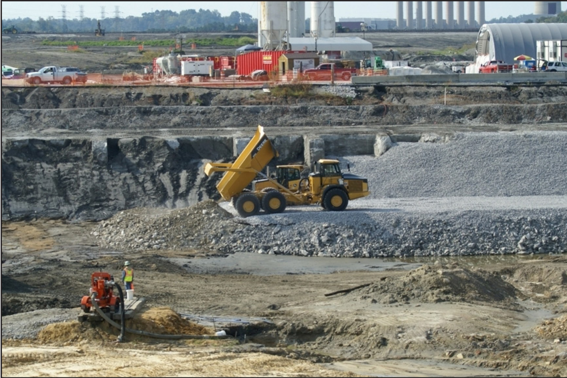
35A – PWS: Constructing haul road at toe of rock buttress along Segment 8 of the perimeter wall. September 24, 2012.
