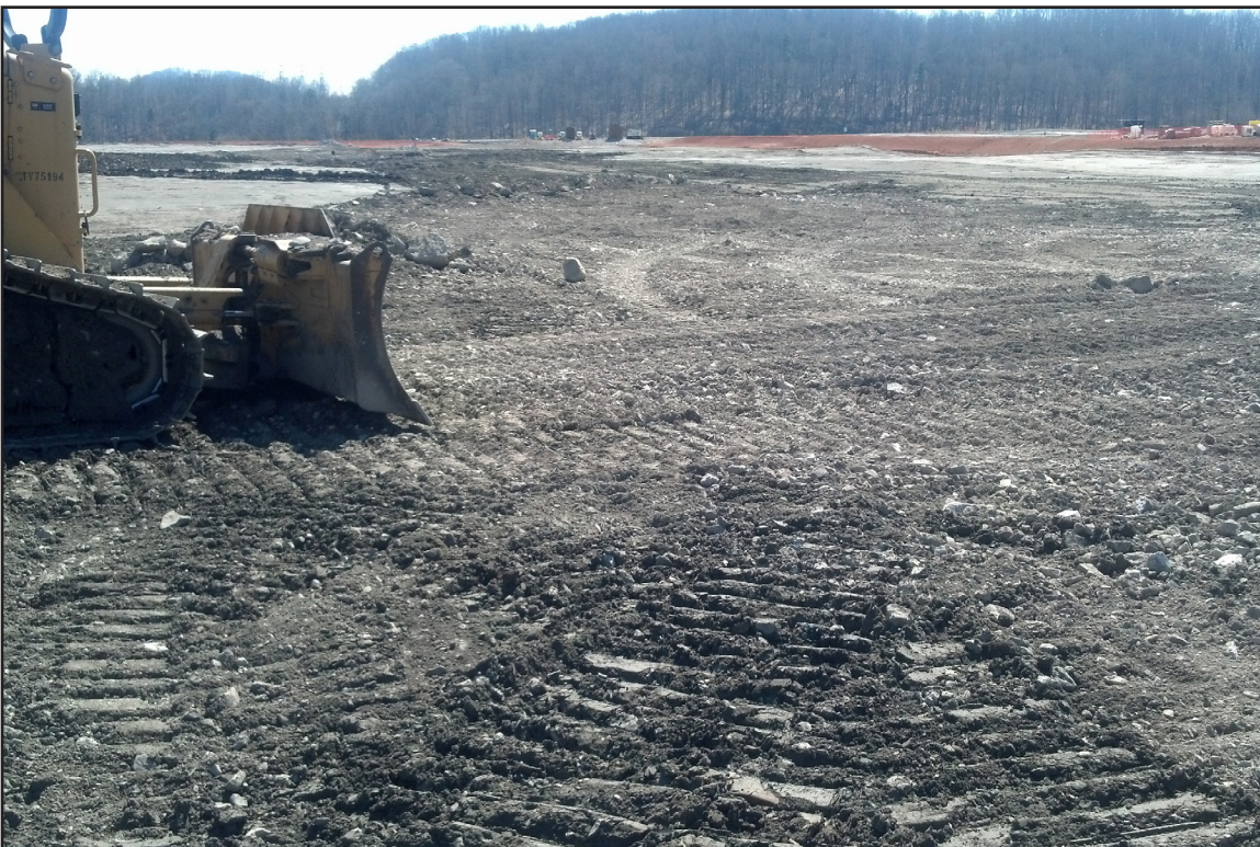
20B – Ash stacking: Stabilization of the subgrade in the Ash Pond using a gravel base. March 20, 2014.
