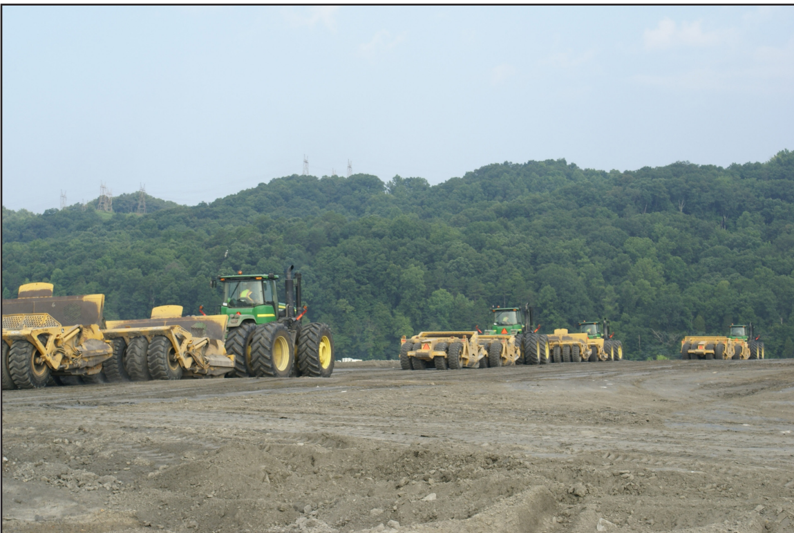
14B – Ash Removal: Removal of ash from the relic portion of the southern Dredge Cell using tractors equipped with pan scrapers. July 18, 2013.
