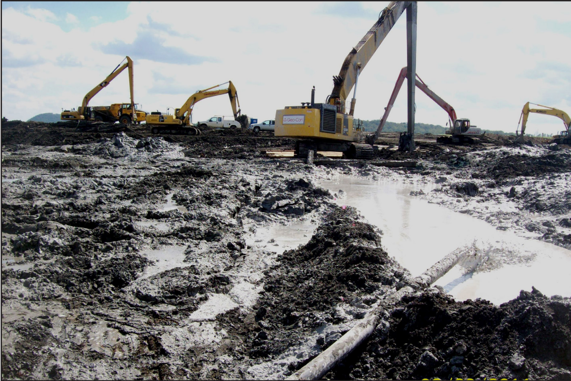
29A – PWS: Platform deterioration occurred due to rainfall and high water table, resulting in very wet conditions under excavator. September 29, 2011.
