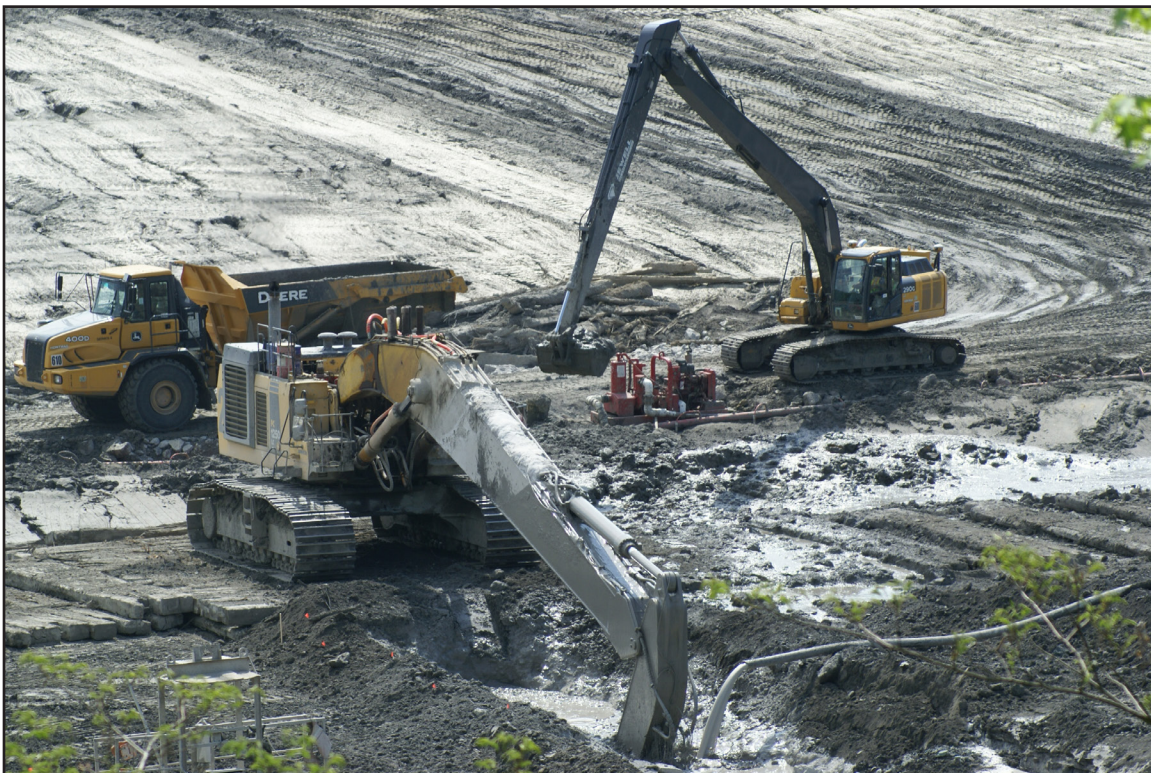
26B – PWS: Management of spoils from the slurry trench excavation. May 13, 2013.
