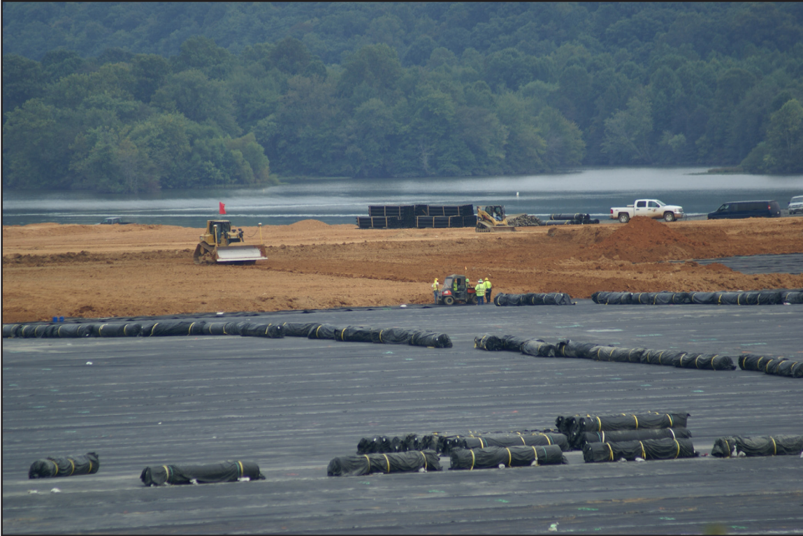
39A – Cap and Closure: Phillips & Jordan (P&J) placing multilayer cap - flexible membrane liner, geocomposite, and cap soil. September 16, 2013.
