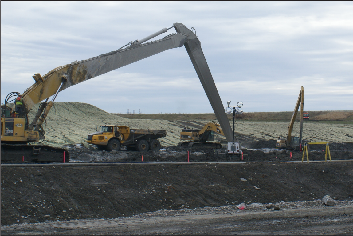
32A – PWS: Slurry trench construction platform stabilized by raising the platform above ground. February 12, 2012.
