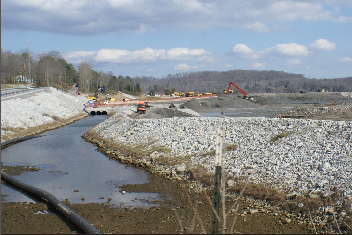
48A – Stormwater Management: Clean Water Ditch used to bypass stormwater around the Middle Embayment. April 5, 2013.
