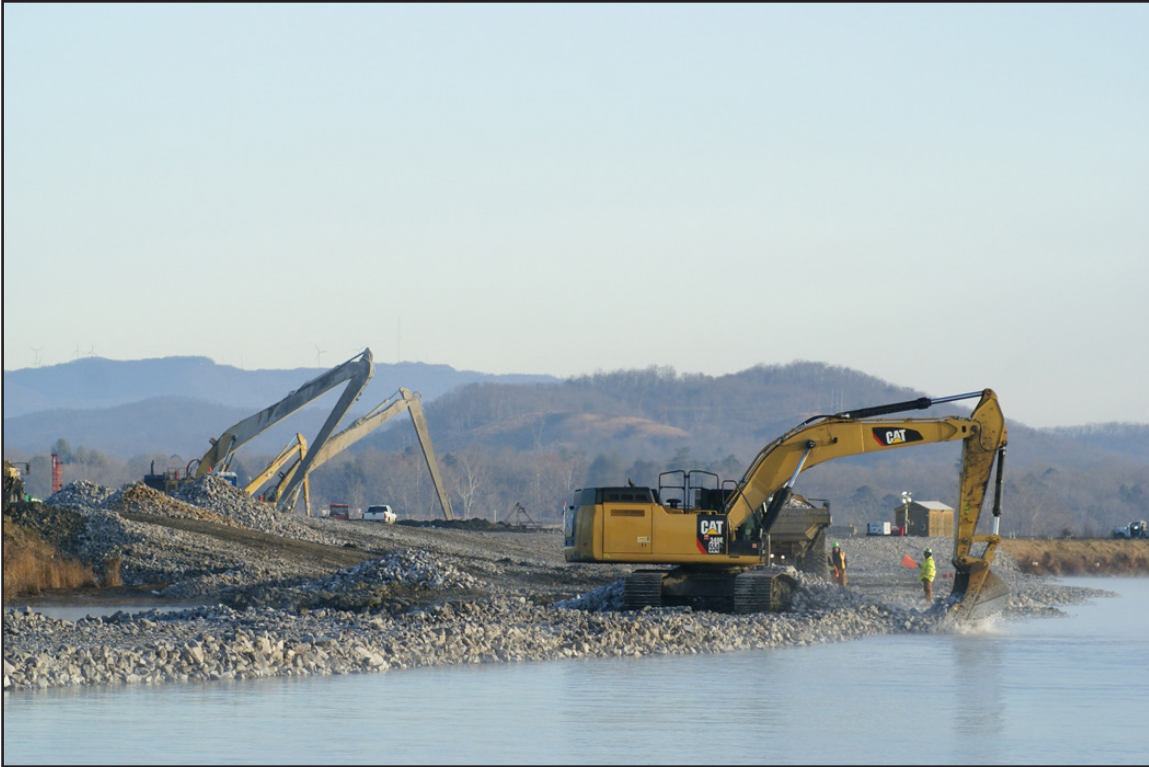
36A – Perimeter Containment: Placing rock in Stilling Pond as a buttress to stabilize the divider dike prior to slurry wall construction. December 11, 2012.
