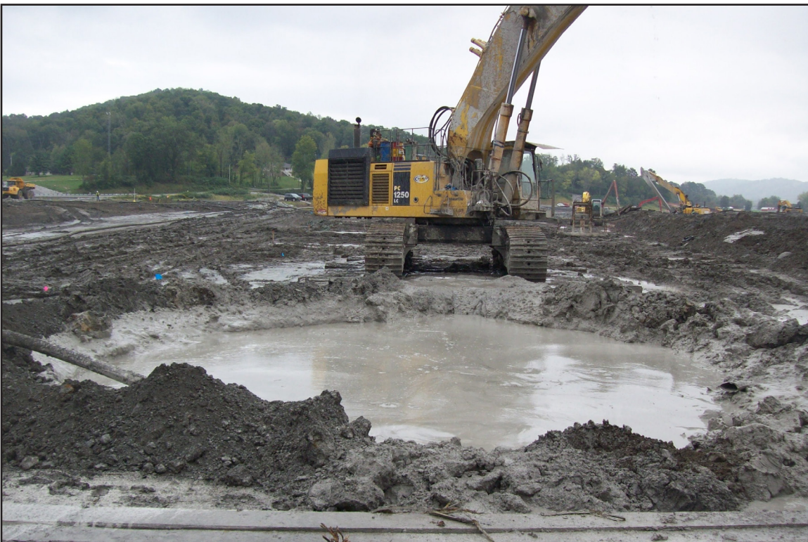
30B – PWS: Slurry trench collapse, resulting in wide trench at top. September 23, 2011.
