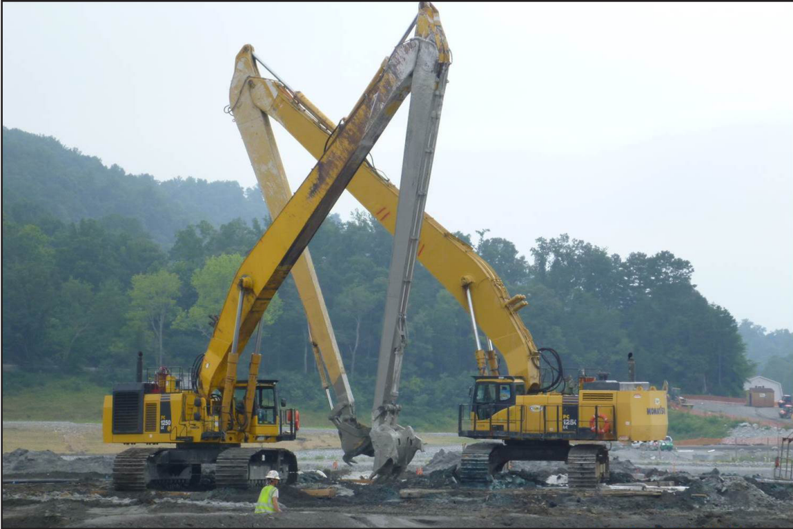
25A – Perimeter Wall Stabilization (PWS): Long-reach excavators used for slurry trench construction. July 21, 2011.
