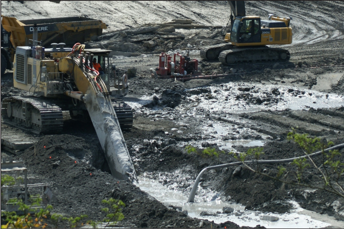
30A – PWS: Platform deterioration due to spoils spillage onto ground surface next to the trench. May 13, 2013.
