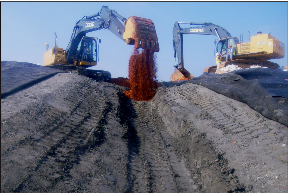
47B – Stormwater Management: Placing clay to line ditch in flumes for erosion control. August 28, 2013.
