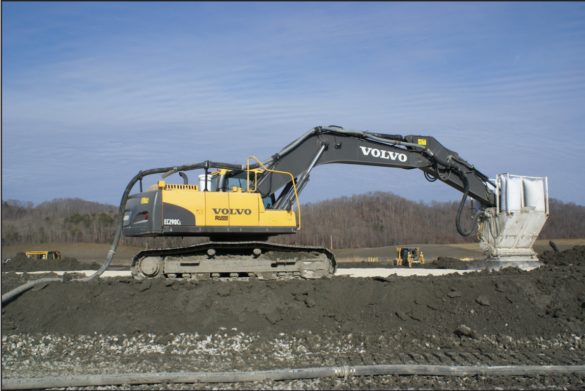
17A – Ash Processing: Using lime treatment plots in the Ball Field area; application of lime. February 8, 2011.
