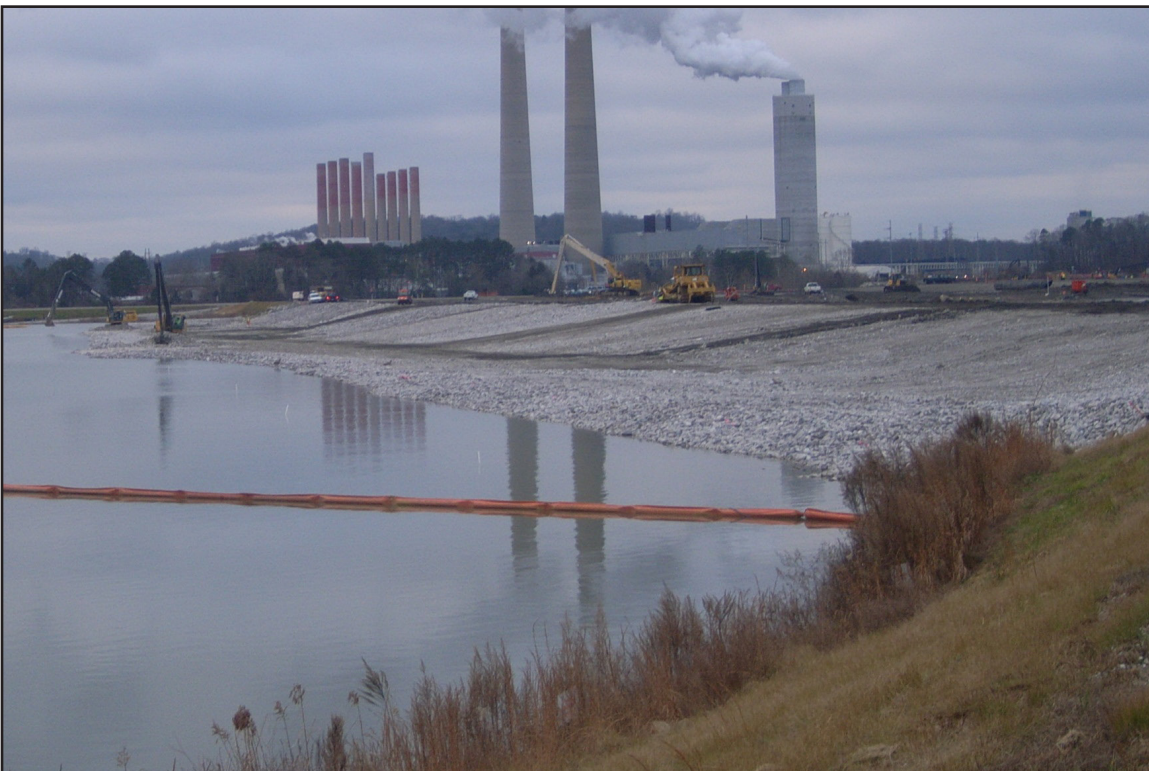
36B – Perimeter Containment: Completed buttress along the divider dike. December 27, 2012.
