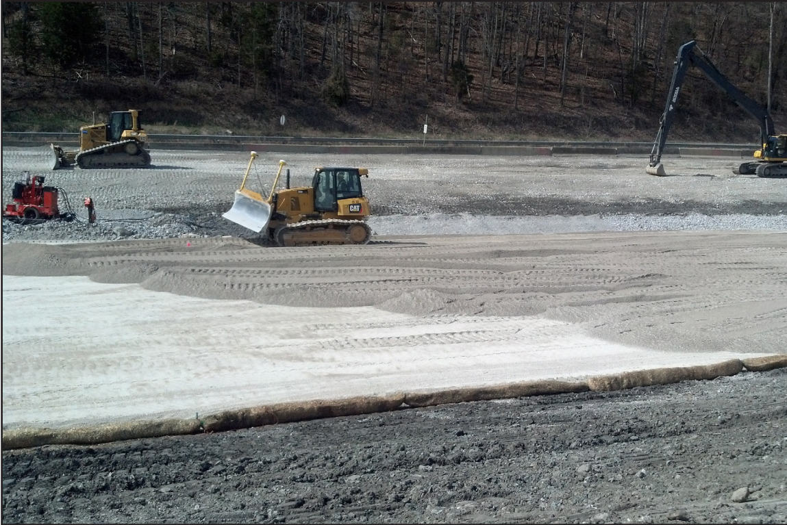
37A – Perimeter Containment: Placing sand as filter layer for construction of the perimeter containment berm. March 20, 2014.
