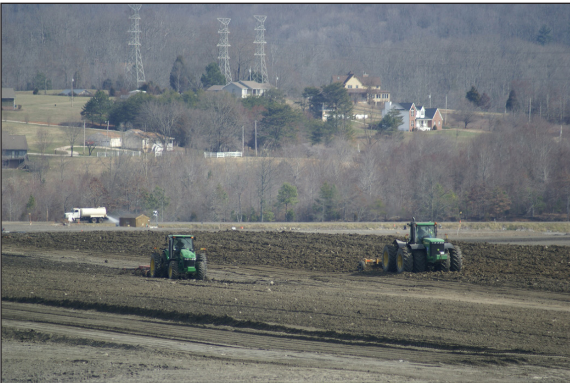
16B – Ash Processing: Using sundrying plots in the relic area of the Dredge Cell. February 17, 2013.
