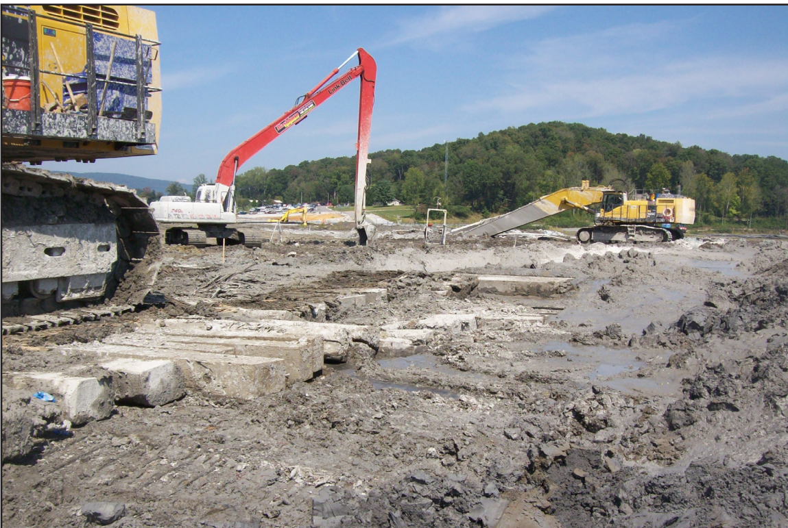
29B – PWS: Platform deterioration resulted in use of crane mats oftentimes stacked several layers thick. September 14, 2011.
