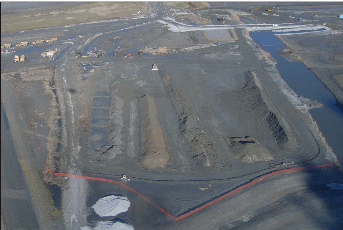
15B – Ash Processing: Using windrows in the Ball Field area. January 3, 2013.
