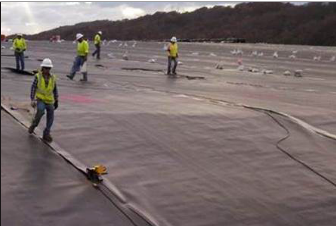
39B – Cap and Closure: Chesapeake Containment Systems (CCS) hot seam welding of the flexible membrane liner. July 2013.
