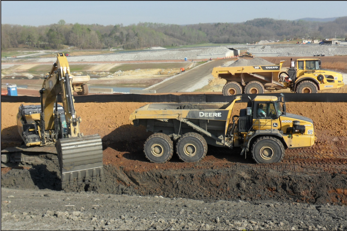
19A – Ash Stacking: Infill stacking next to the perimeter berm in the Dredge Cell. April 10, 2013.
