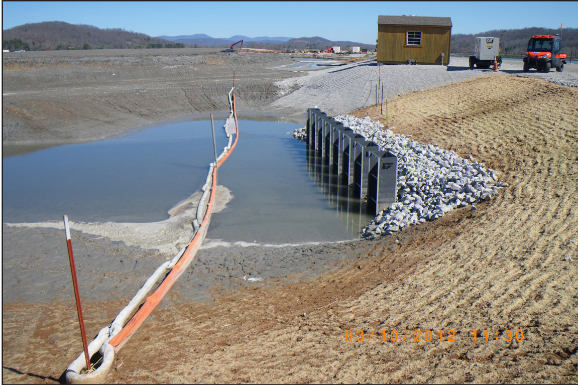
24A – Ash Pond Outlet Structure (Agridrains). March 10, 2012.
