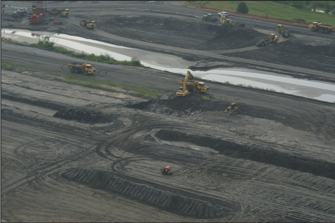
15A – Ash Processing: Using windrows in the Ball Field area. May 23, 2011.
