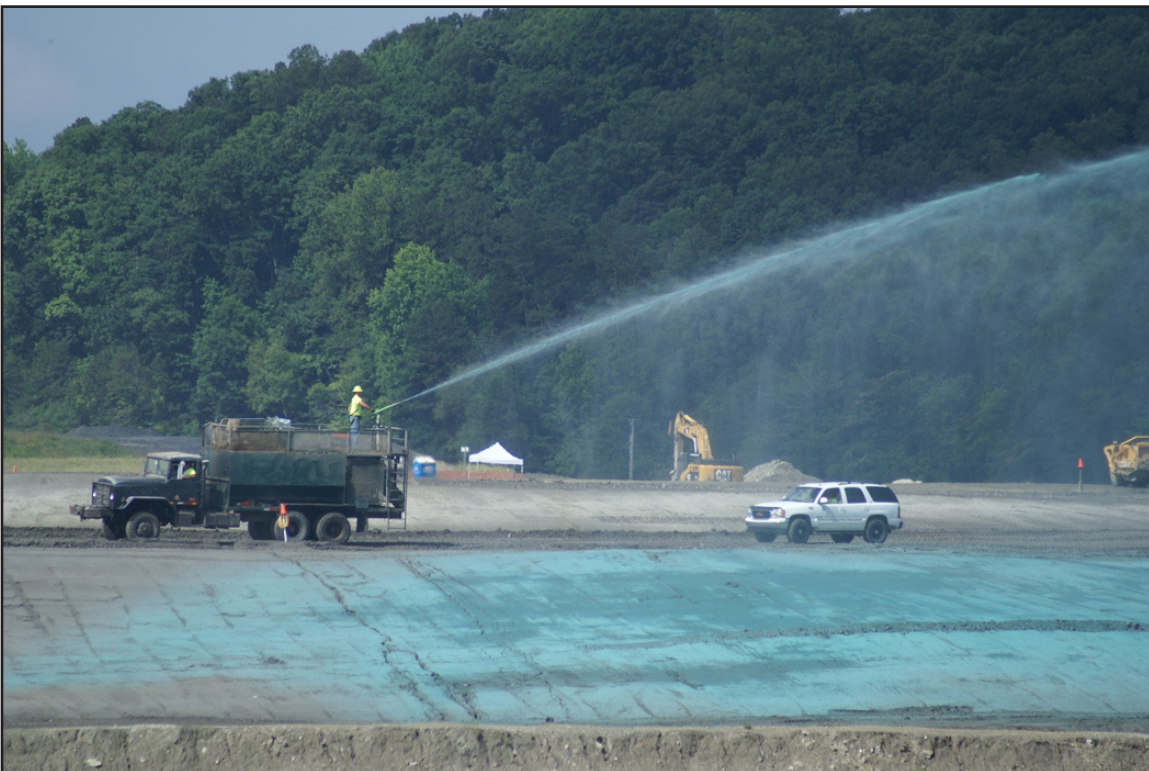
49B – Dust and Erosion Control: Holleman spraying Flexterra to minimize dust and erosion. May 29, 2012.
