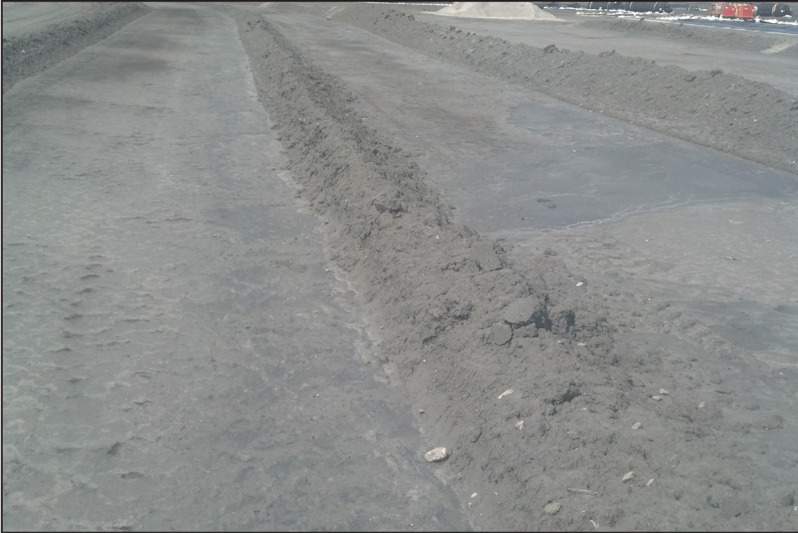
21A – Ash Stacking: “Clipping” off wet subgrade to allow stacking to continue in wet or freezing weather during the winter. April 3, 2014.
