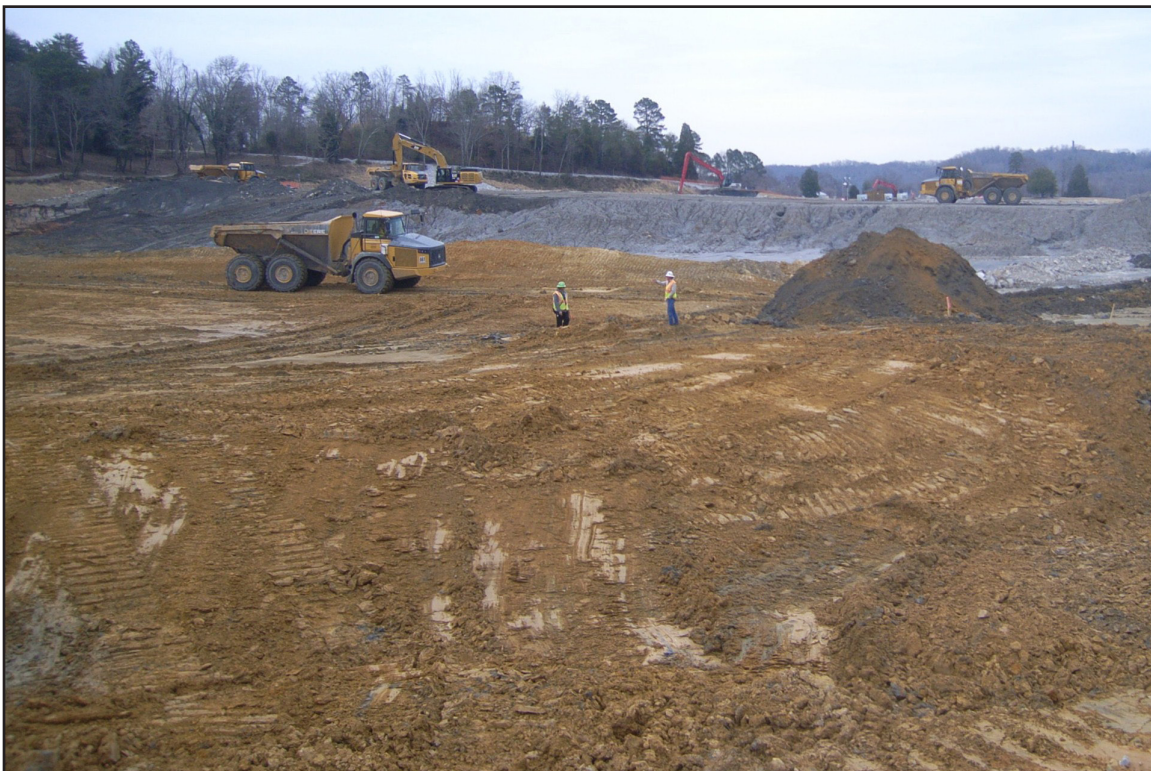
11B – Ash Removal: Bottom of Sediment Basin following ash removal and excavating Dike 2. February 7, 2013.
