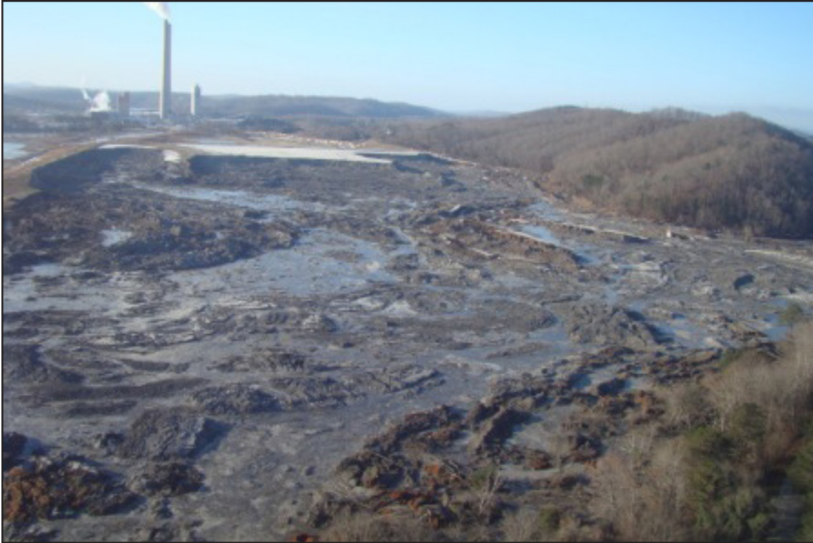
3A – Oblique of the failed Dredge Cell after release (viewing from the north). January 8, 2009.
