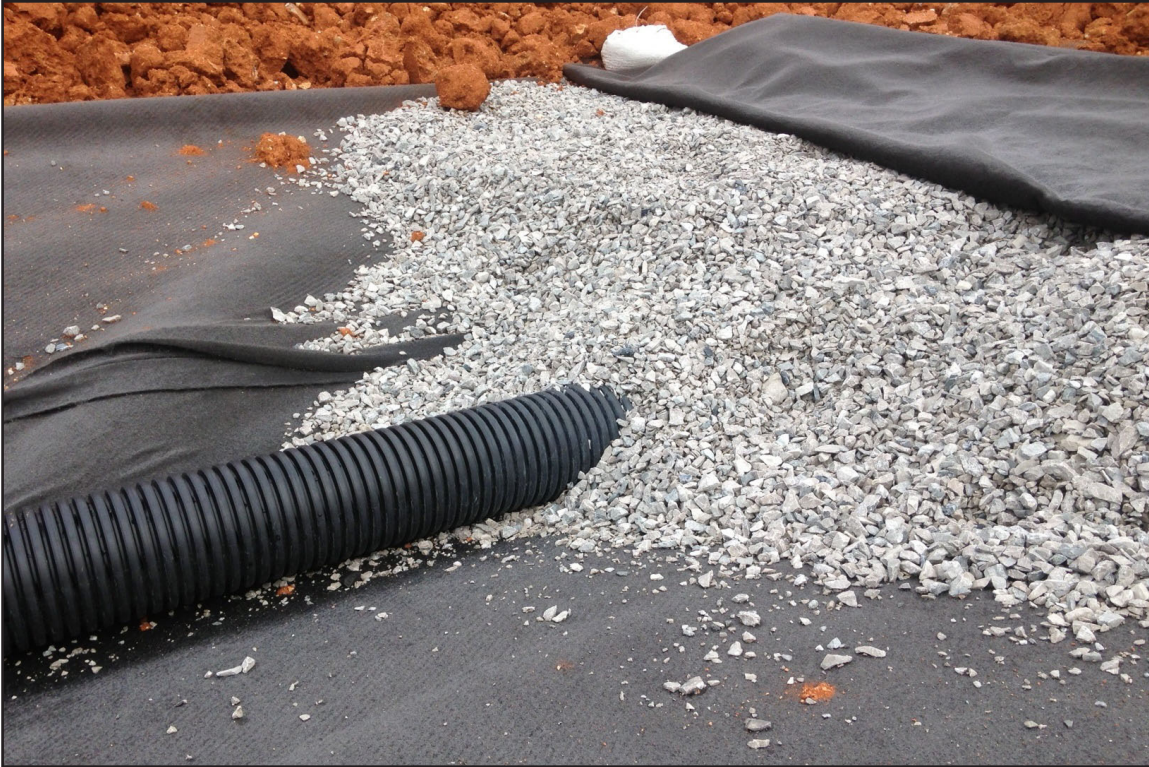
43A – Cap and Closure: Underdrain pipe in geotextile-wrapped gravel bedding for drainage of the cap soil. August 10, 2013.
