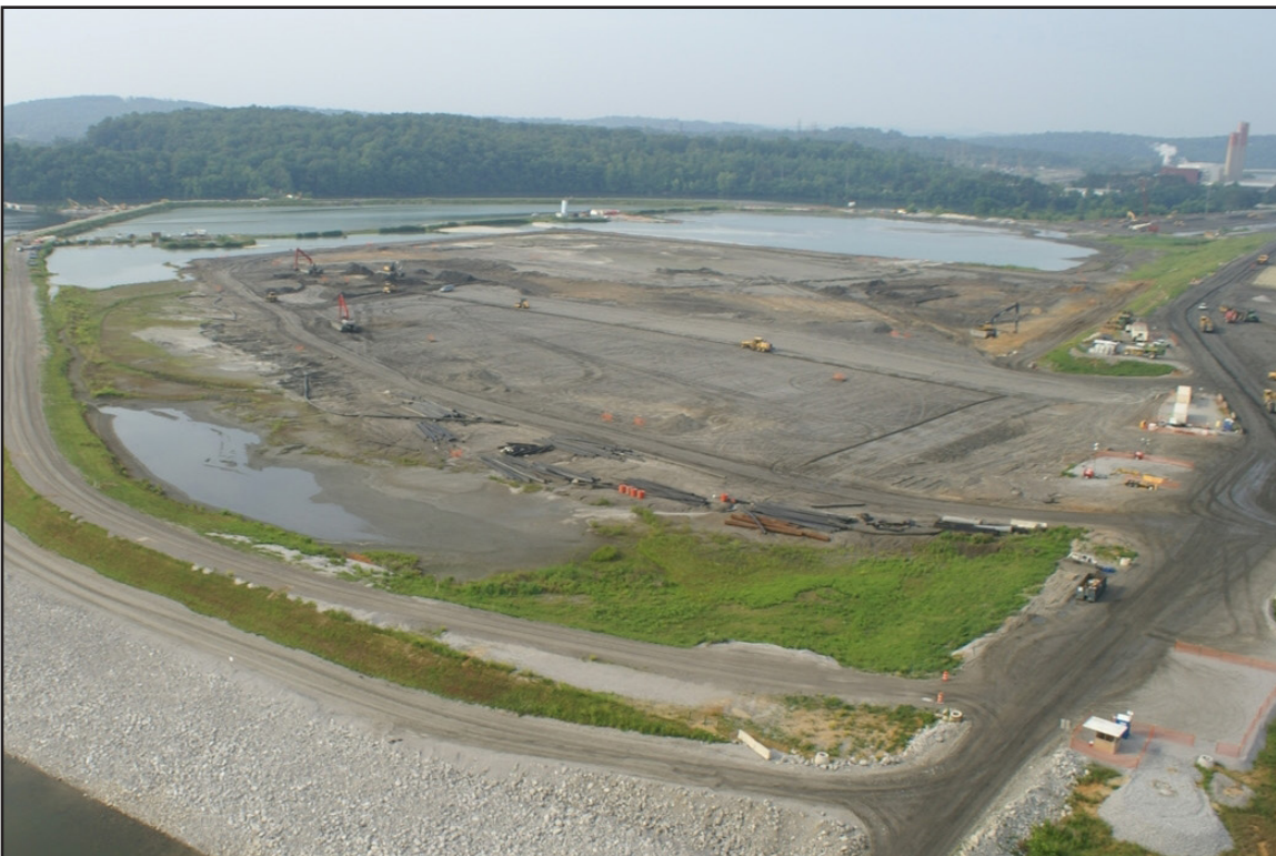
19B – Ash stacking: Stacking in the Lateral Expansion during the subgrade recontouring phase. May 23, 2011.
