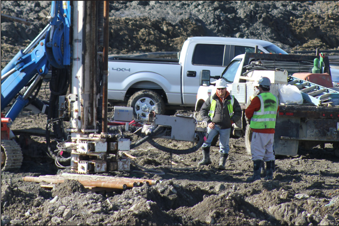
33A – PWS: GeoCon (Armstrong Drilling) predrilling holes for jet grout mitigation of wall defects. January 20, 2014.
