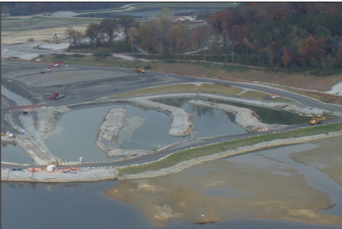
48B – Stormwater Management: Sediment Basin in the Middle Embayment used to treat stormwater from the Site. November 2, 2011.
