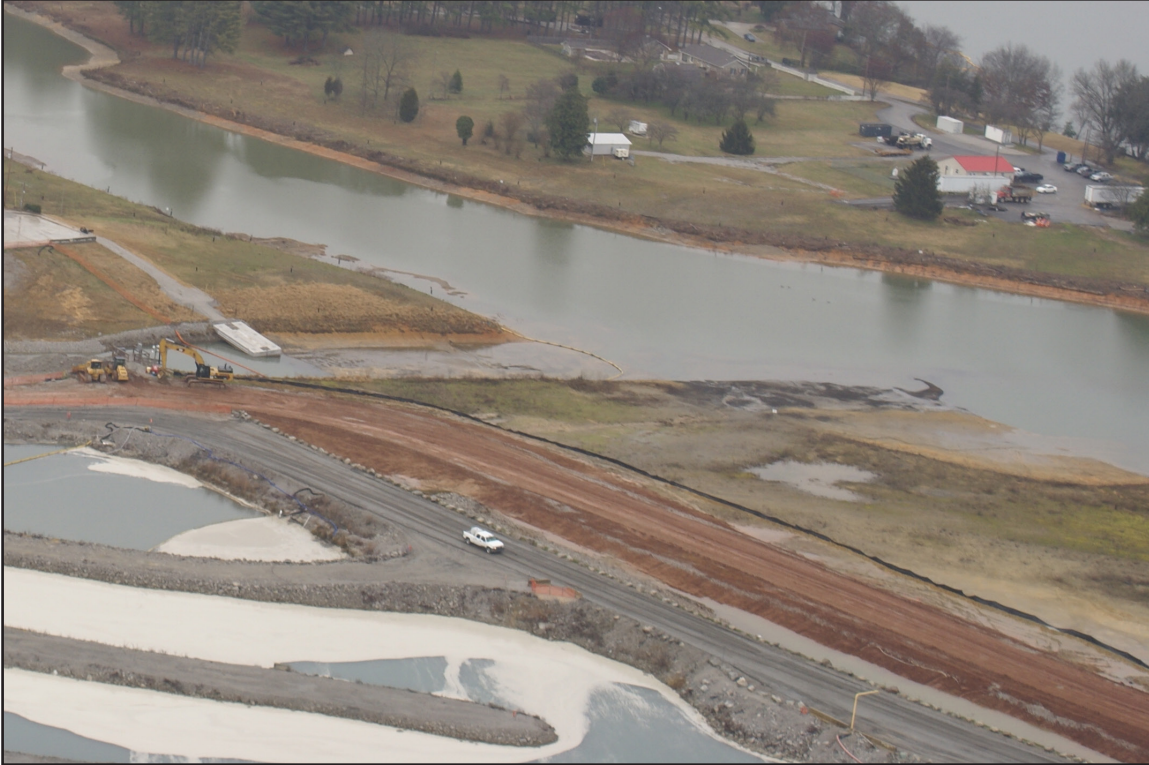
12A – Ash Removal: Construction of Dike 3 on the east side of Dike 2 as a cofferdam for holding back the Emory River from the embayments. June 18, 2013.
