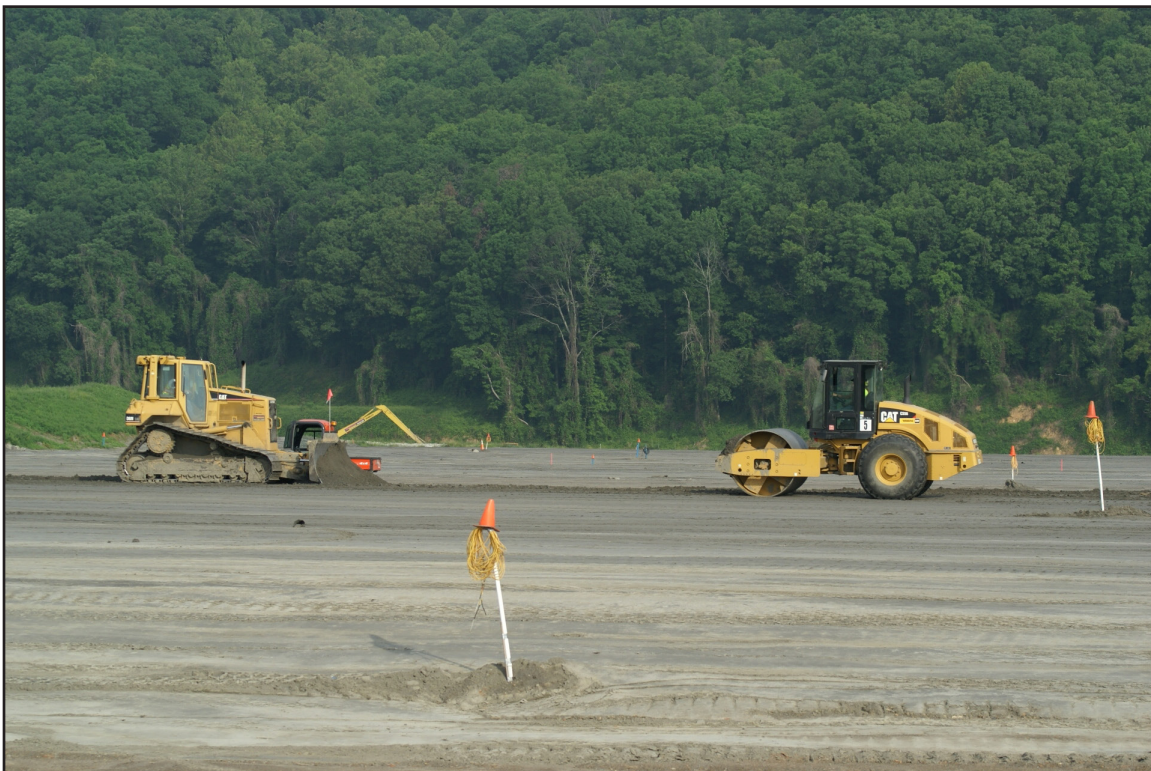
18B – Ash Stacking: Using dozer and smooth drum roller in the Dredge Cell to stack the ash. May 11, 2011.
