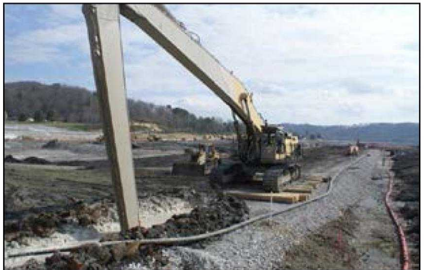
Construction of the slurry wall
