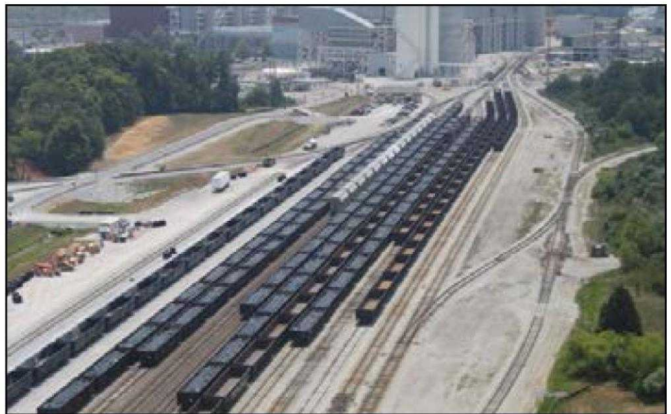
Dewatered ash loaded onto rail cars and ready for shipment
