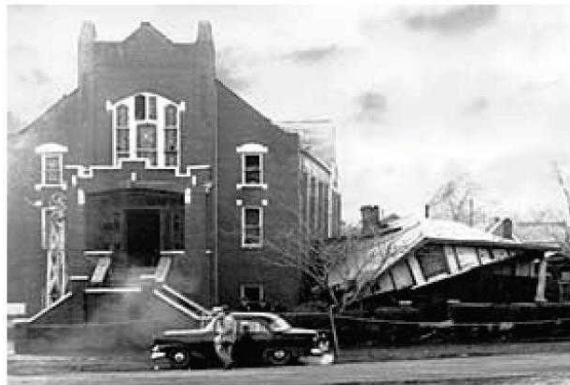
Top: Bethel Baptist Church and the parsonage following a bombing during the Civil Rights movement. Photo courtesy of the Fred Shuttlesworth Foundation
