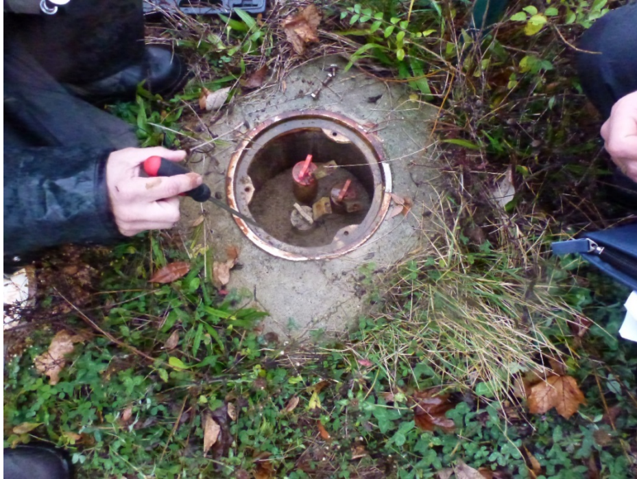
Open wells MW 12 S, M and D. All wells observed were flush mounted, locked and appeared to be in good working order, labels are on inside
