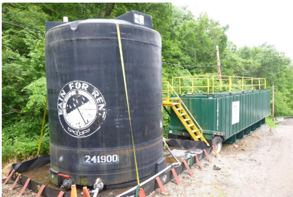
Backup tanks for the current leachate treatment system
