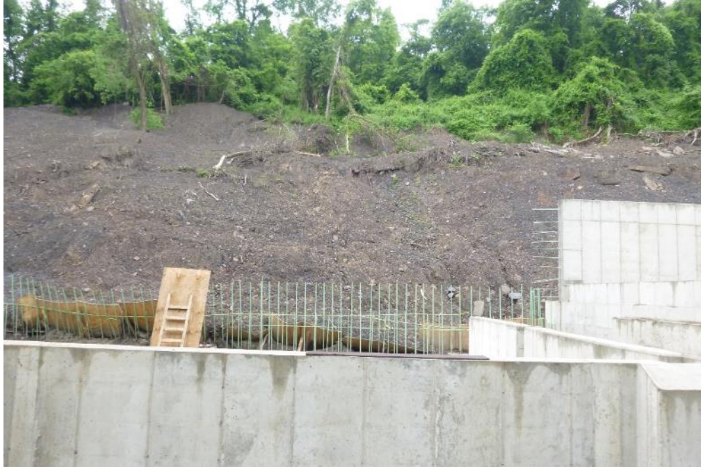
Slumped slope behind retaining wall
