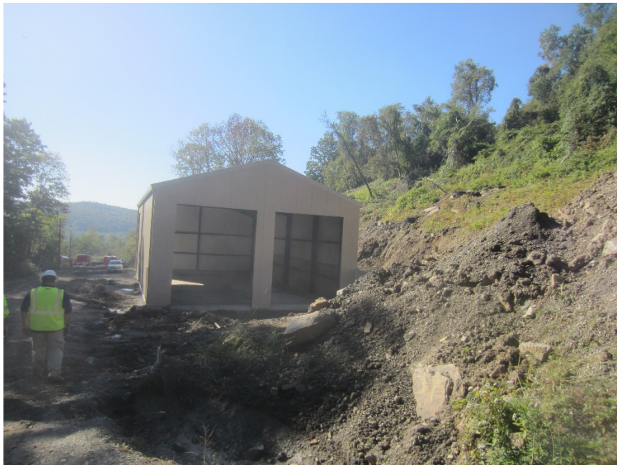
View of the treatment system enclosure on September 23, 2015.
