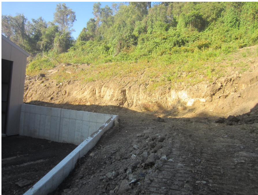
View of the retaining wall and slope adjacent to the new treatment system enclosure at the time of the September 2015 site visit
