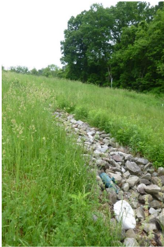
Landfill drainage channel
