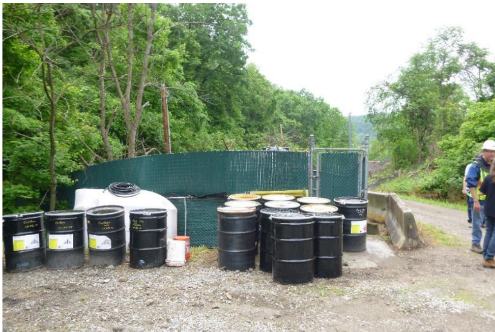
Drums of spent carbon and oil staged outside the treatment system enclosure
