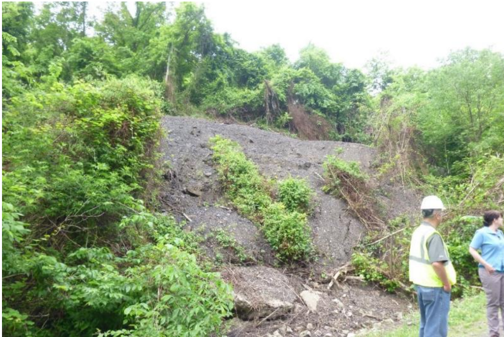
Slumped slope located across the access road from the current leachate treatment system
