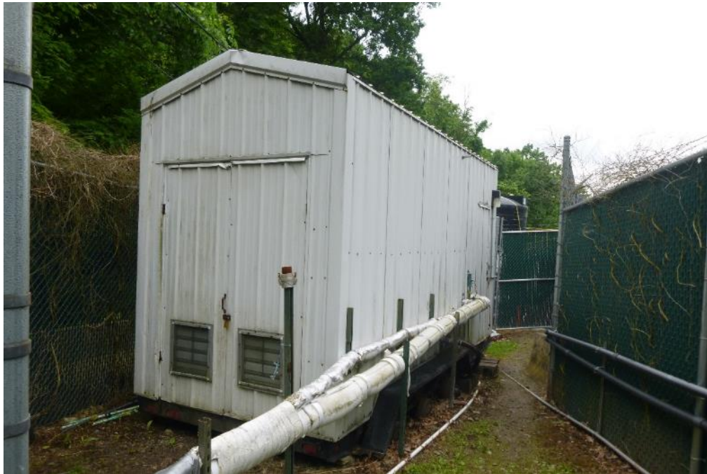
Locked aqueous phase treatment system trailer
