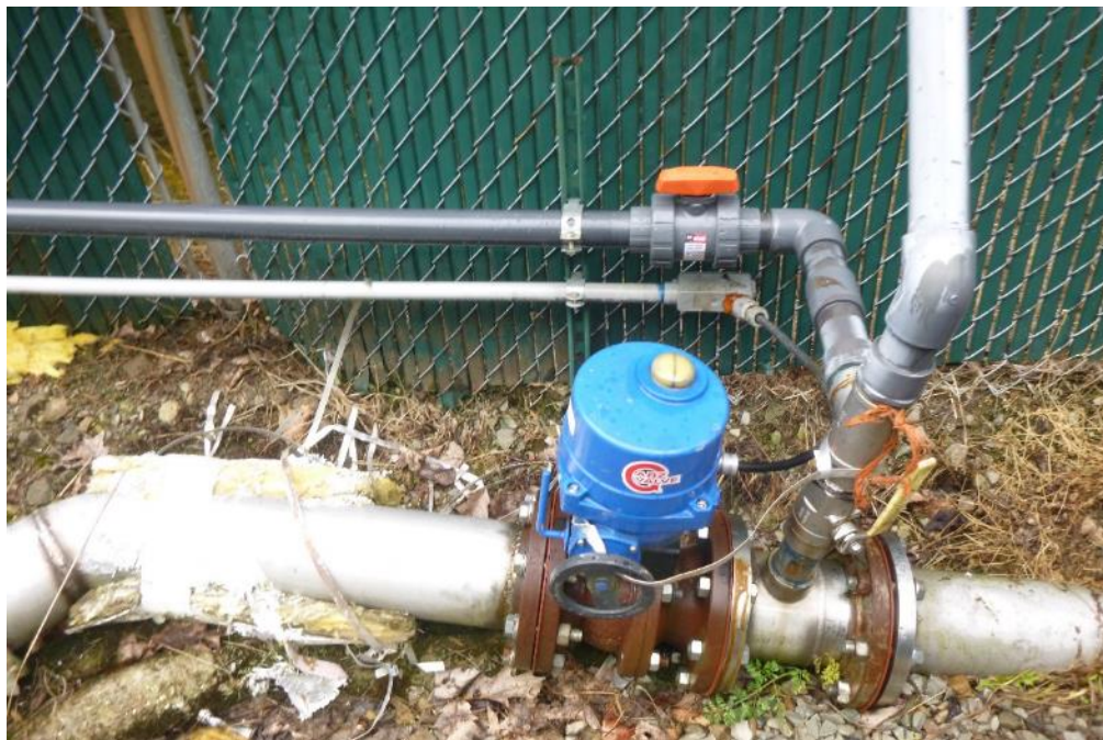
Valve before OWS to bypass to backup tanks, if needed
