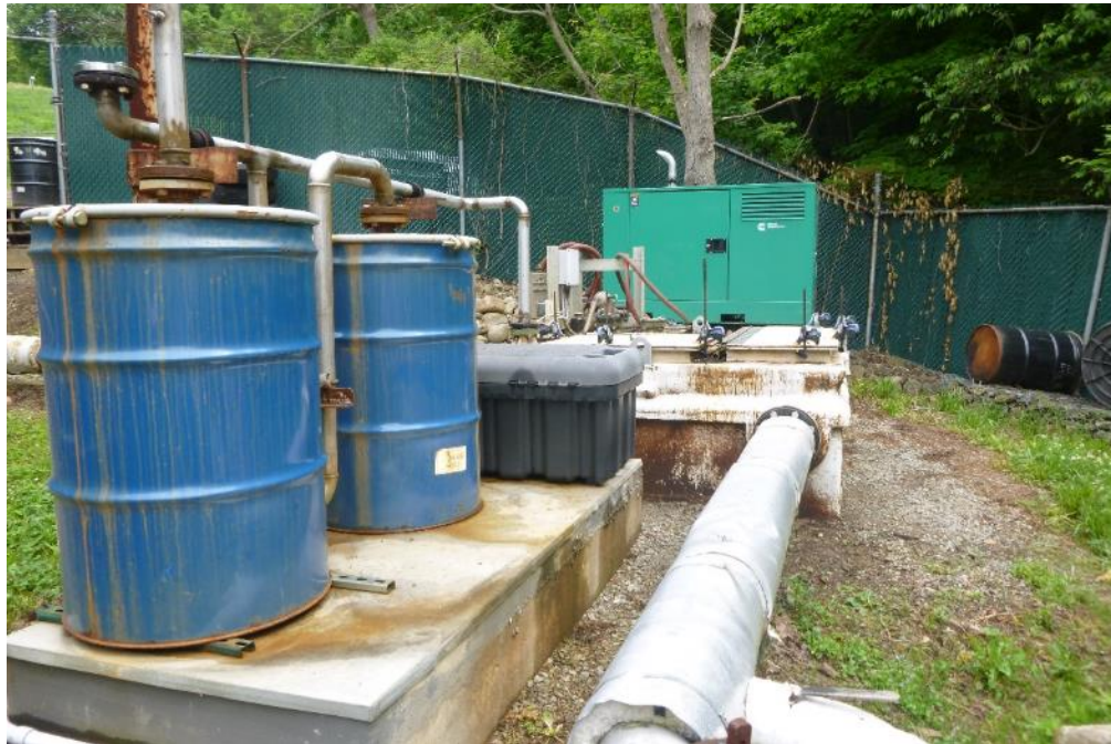
Activated carbon units, OWS and backup generator
