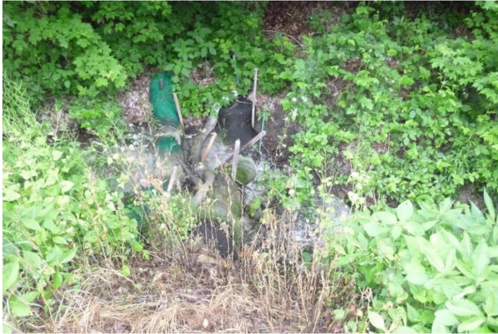
Sediment filter socks in the unnamed stream on site
