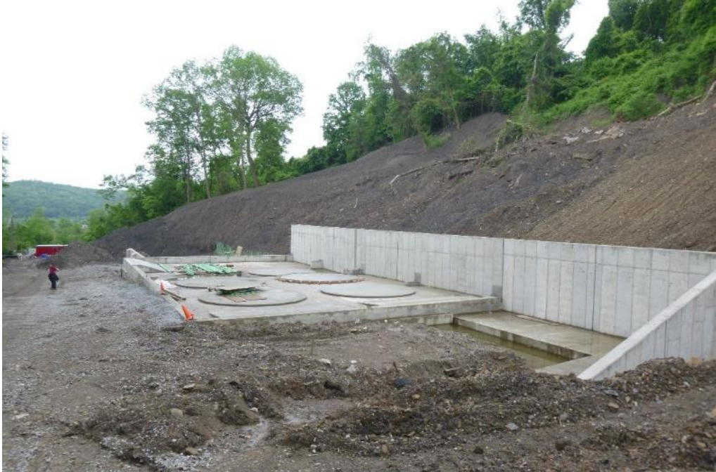
Concrete slab and retaining wall for new treatment system
