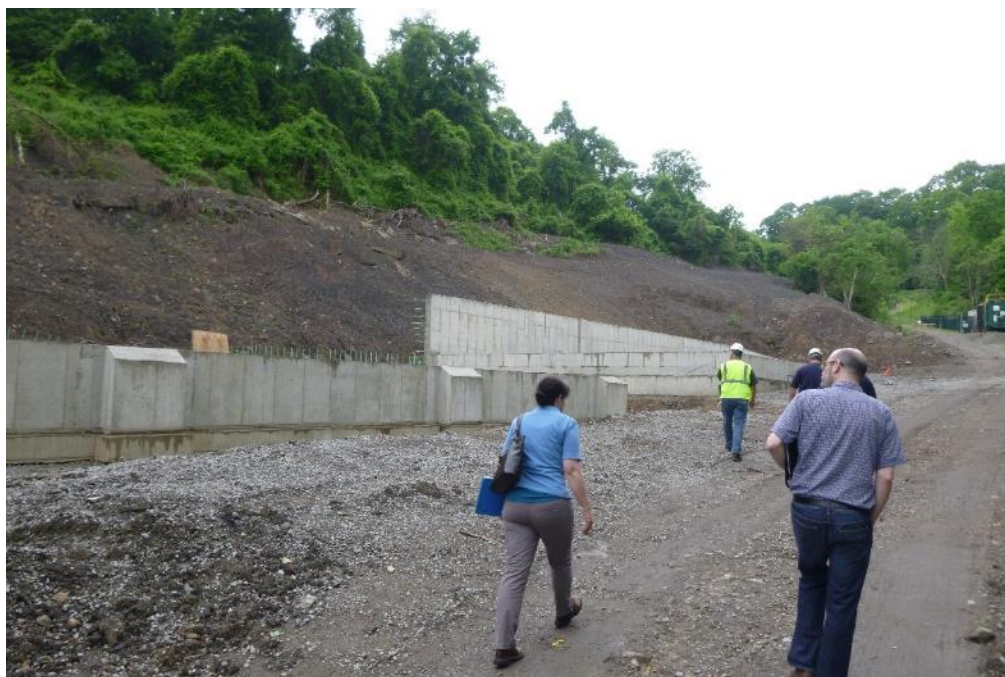
Concrete slabs and retaining wall for new leachate treatment system
