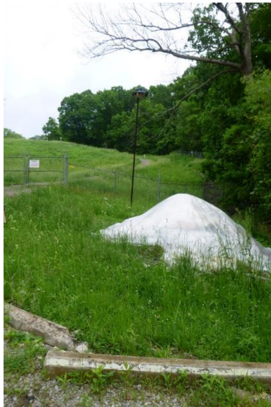
Covered contaminated soil pile generated during manhole replacement
