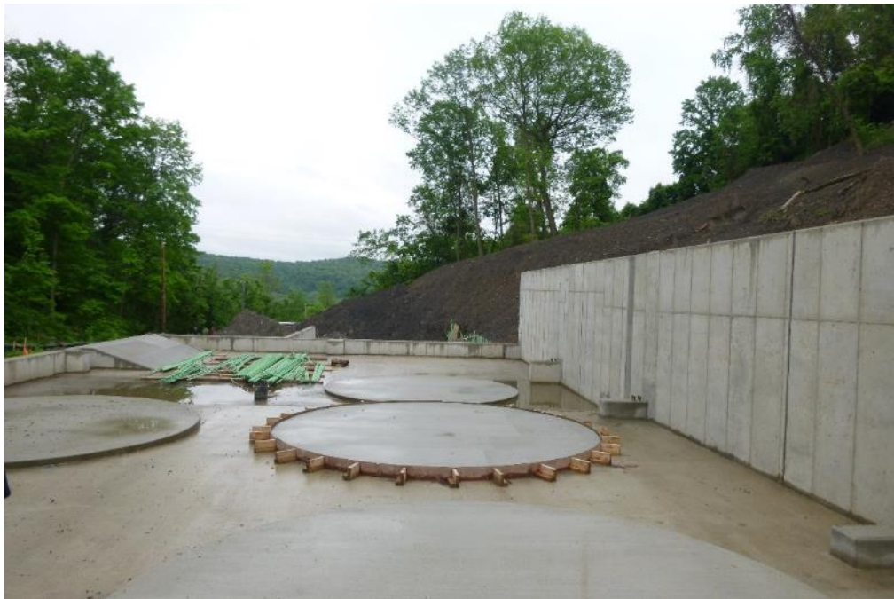
Concrete slab for new treatment system tanks
