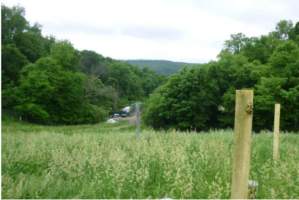
View of landfill cap looking downslope toward the leachate treatment system
