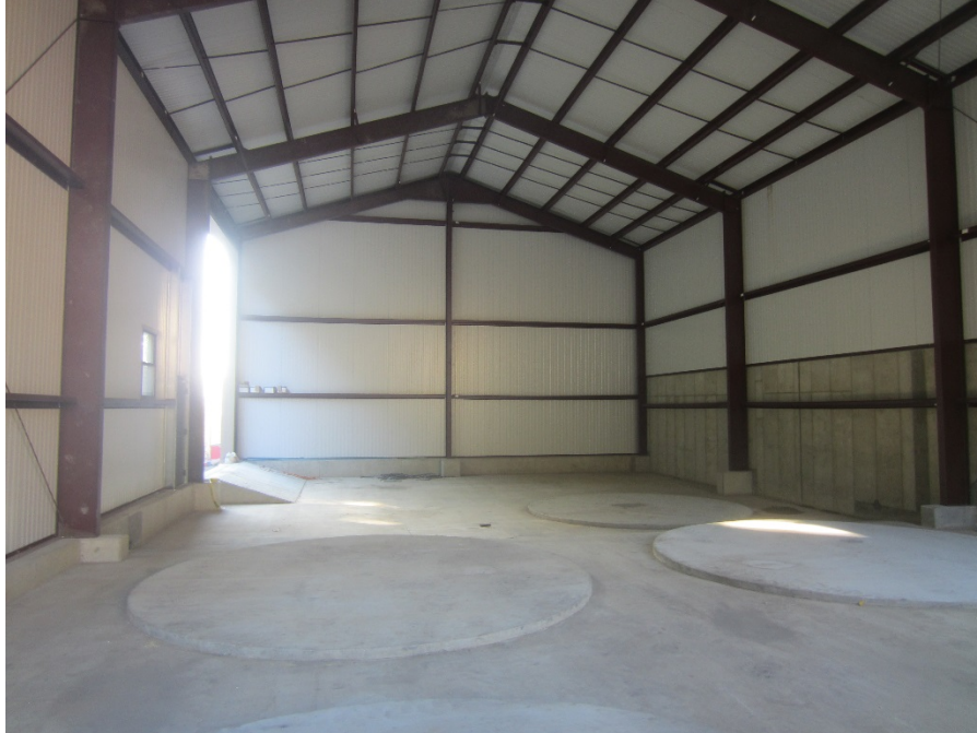
View of the treatment system enclosure interior during the September 2015 site visit
