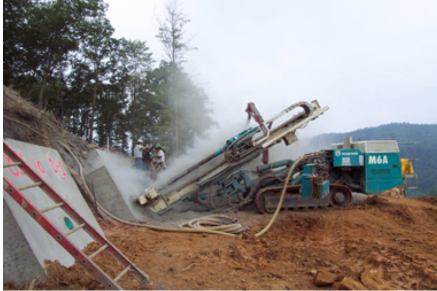
Soil Nailed Wall with Shotcrete Cover- Drilling for Nails
