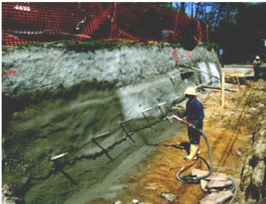
Soil Nailed Wall with Shotcrete Cover
