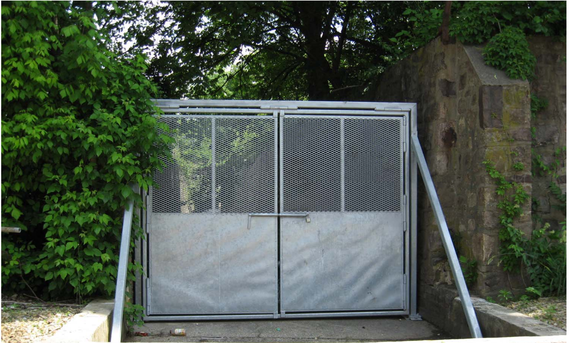
Rose Valley Creek at Maple Avenue Swing Gate after storm Lee cleanup. The swing gate opens slowly as pressure from the water builds up.
