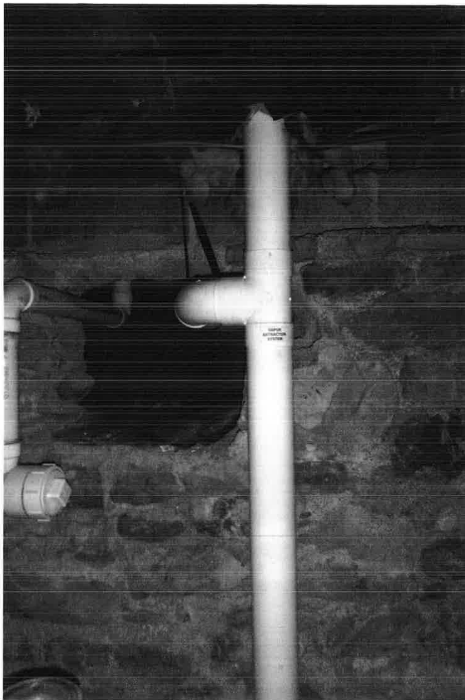
OU3 vapor intrusion piping at residence
