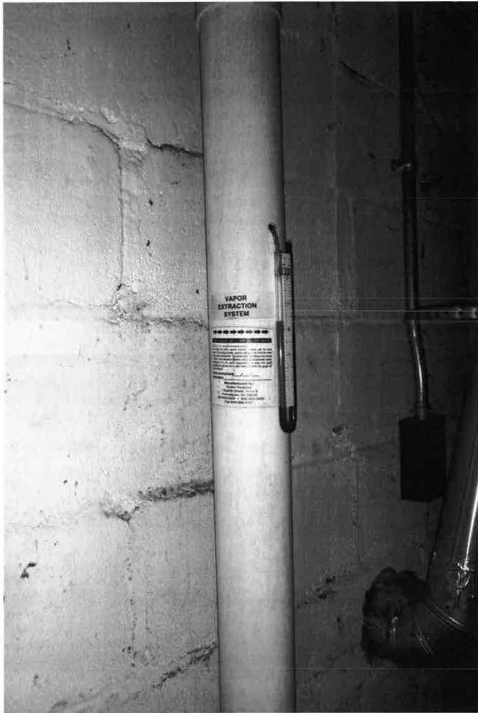
OU3 vapor intrusion piping with vacuum gauge
