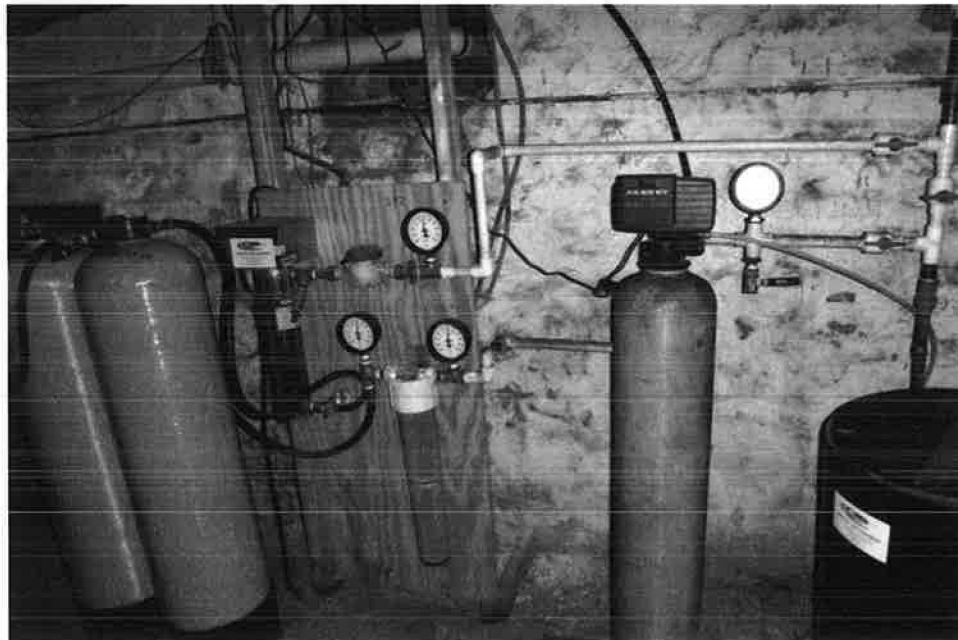
OU1 residence well filtration system and panel
