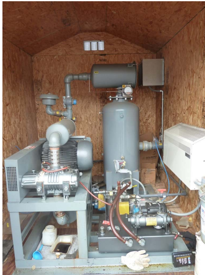
SVE system components within Shed 90B
