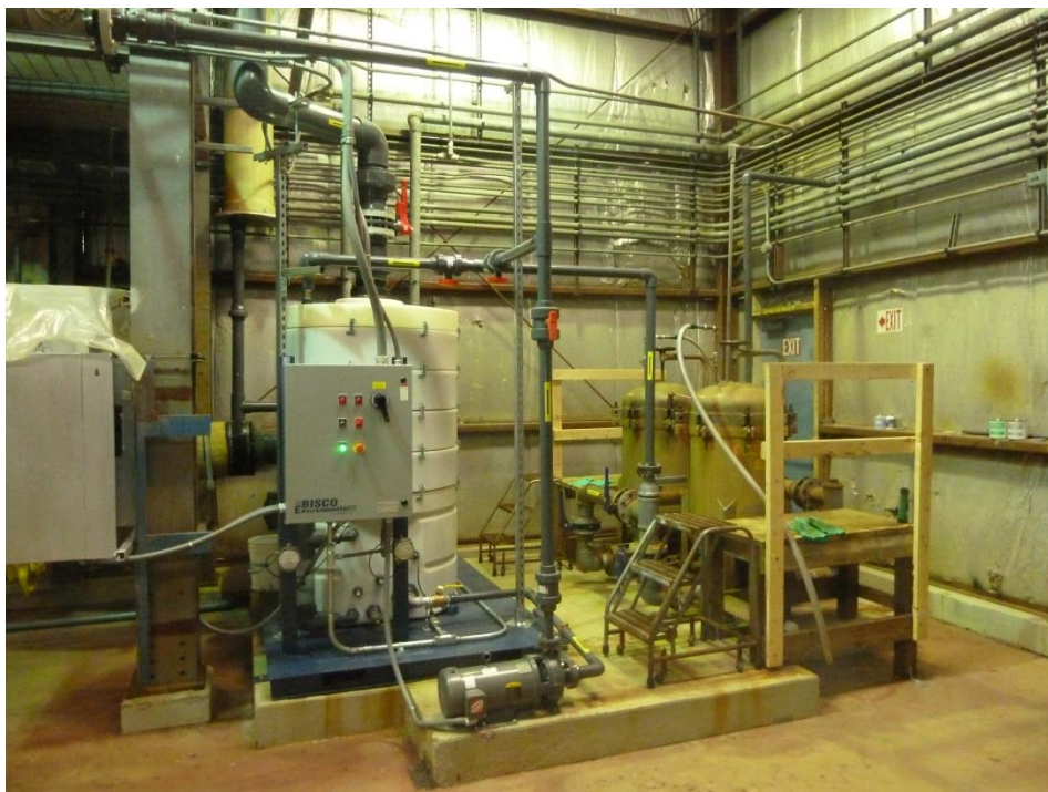
New air stripper inside ground water treatment plant
