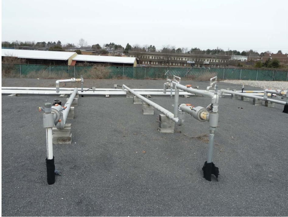
SVE system aboveground piping in former tank farm/process area
