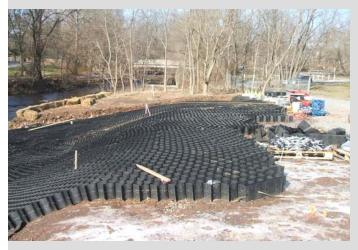
The next steps in stabilizing the stream bank will include rip rap stone placement along the bank, filling the geocells with soil and seeds, and the placement of erosion mats, and hydroseeding in the spring.
