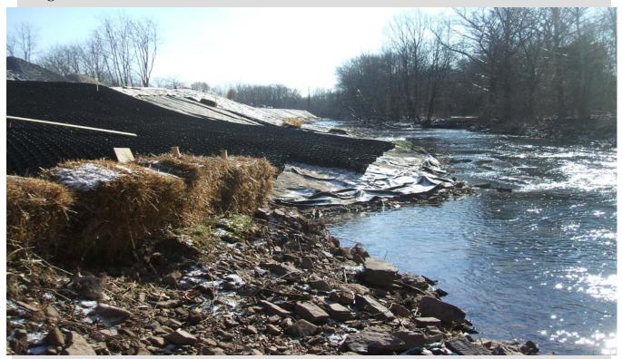
The picture above shows the stream bank of the Wissahickon Creek as the geotextile fabric and the geocells were being placed.
