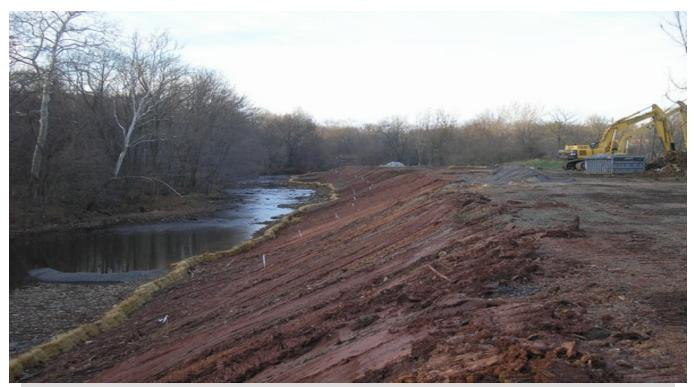
This picture shows the stream bank of the Wissahickon Creek before the geotextile mats and the geocells were placed. Appropriate erosion controls were placed while the prep work was being conducted.
