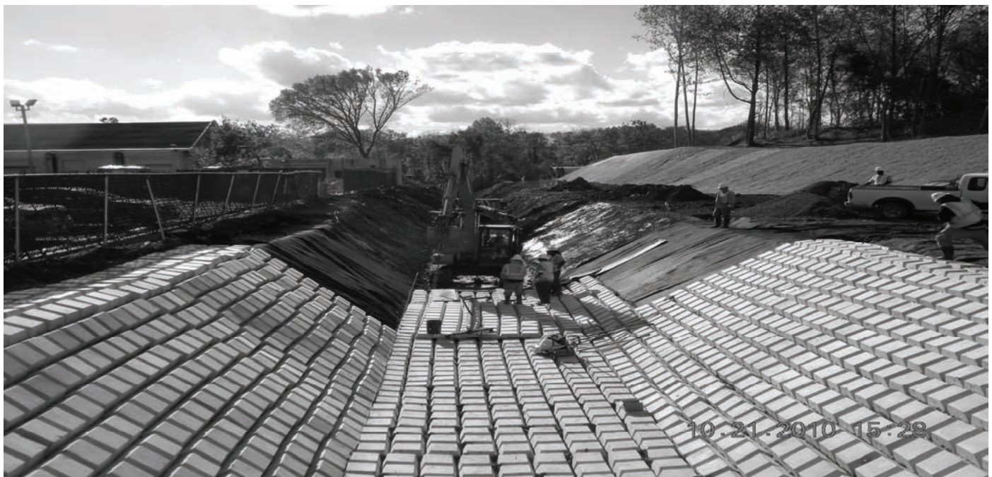
The photo above shows contractors placing concrete-cabled mats in Tannery in order to stabilize the stream bank.
