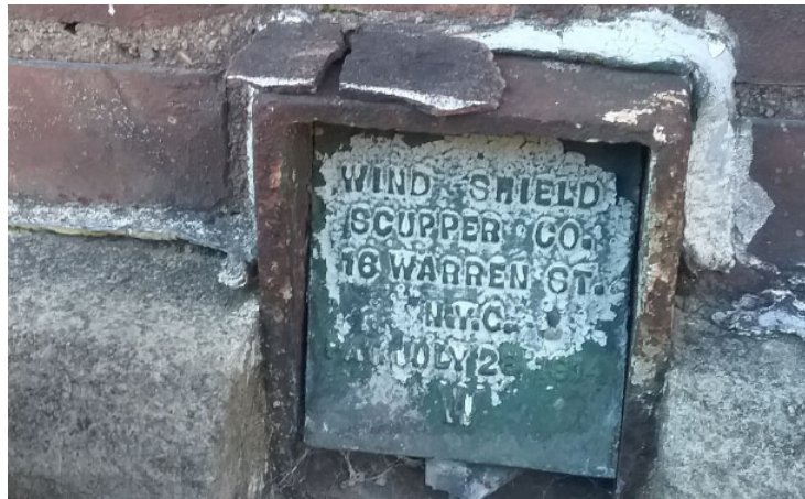
Typical “windshield scupper” located on Building #9 at the Site.
