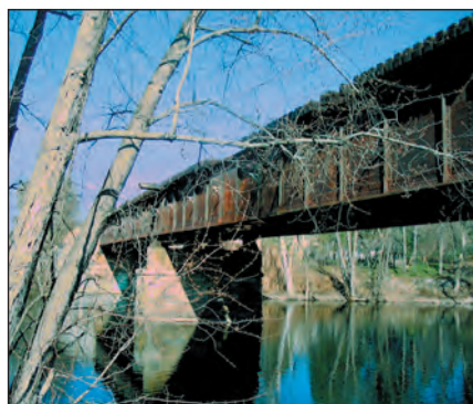
Rail Trestle over the Hudson River
