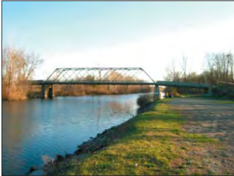
1 Champlain Canal Corridor, East Road Bridge
