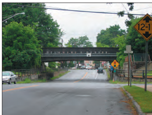
Rail Trestle over Route 4 in Fort Edward
