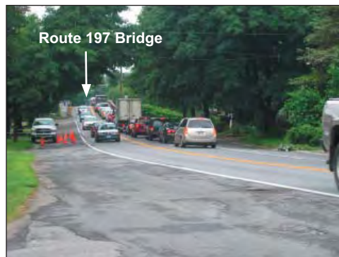
On Rogers Island, Looking East Towards Route 197 Bridge
