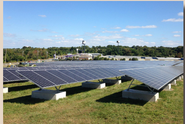
The panel mounting system installed as part of the Sullivan's Ledge solar array. The system consists of panels and ballast blocks mounted to concrete pads (see concrete pads without ballast blocks in the foreground). The pads allow the landfill cap to remain undisturbed.
