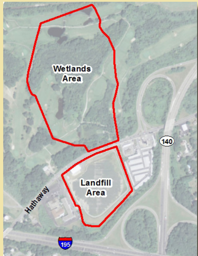
Aerial view of the site prior to solar installation.
