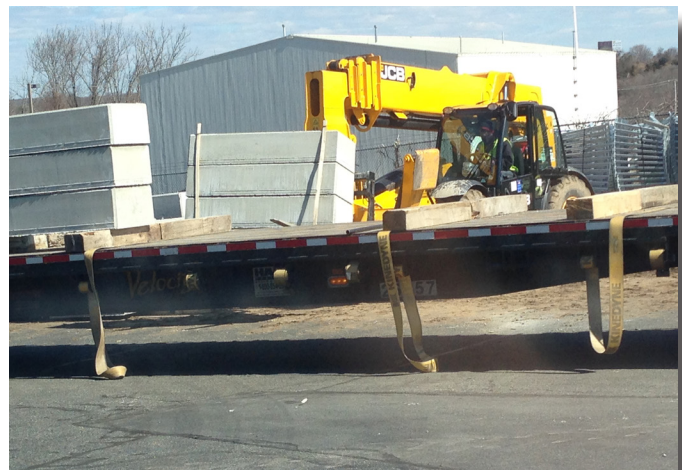
Unloading concrete ballast blocks at the site.
