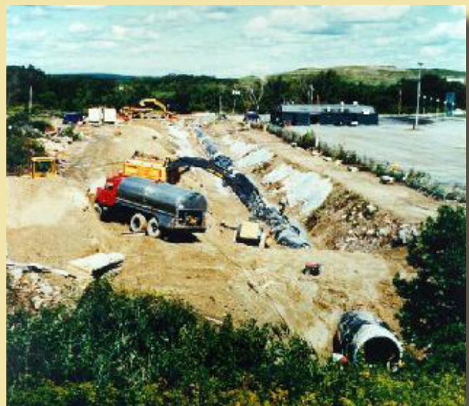
Construction of stormwater infrastructure near the landfill cap in 1998.
