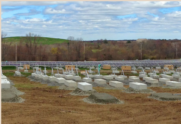
The panel mounting system installed as part of the Sullivan's Ledge solar array. The system consists of panels and ballast blocks mounted to concrete pads (see concrete pads without ballast blocks in the foreground). The pads allow the landfill cap to remain undisturbed.
