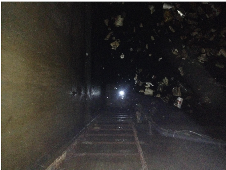
Picture 8 – Town 1 Debris in Holding Tank
