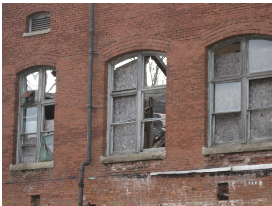
Photo 6: Collapsed roof and broken windows of the on-site building
